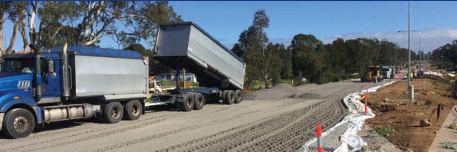
Placing road base on eastbound carriageway, Bringelly Road, looking west.
