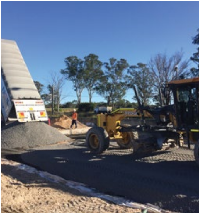
Placing road base on eastbound carriageway, Bringelly Road.
