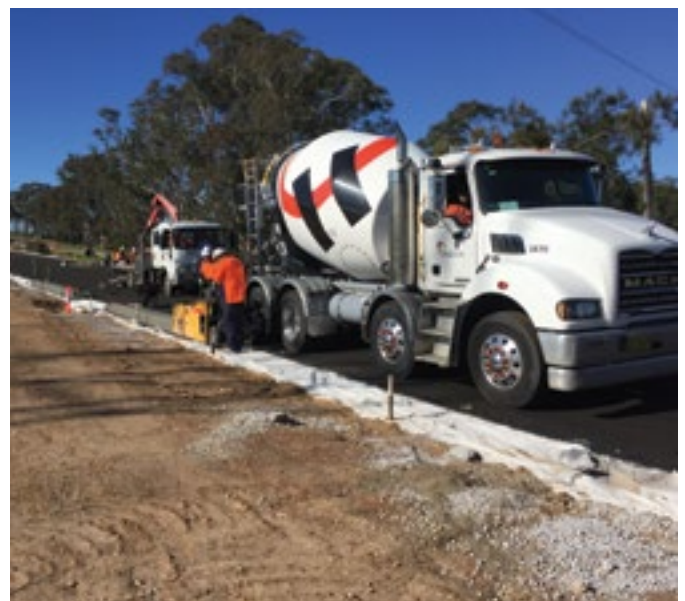
Construction of kerbing on eastbound carriageway, Bringelly Road.
