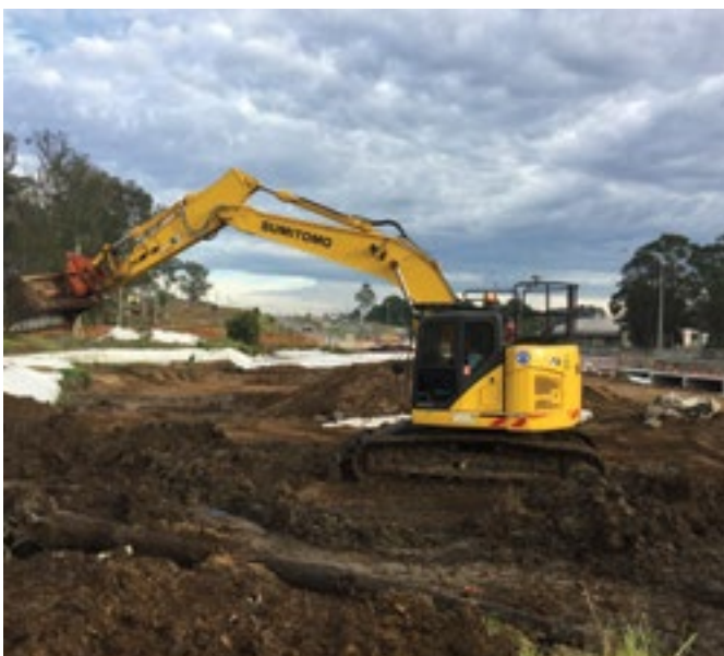
Excavation of Bonds Creek. Looking east.
