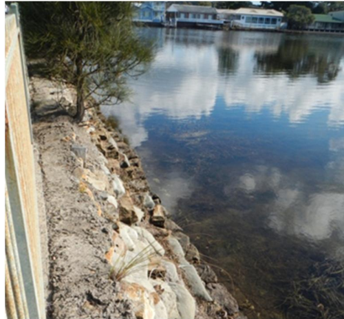
Figure 6-5 Stone construction of the causeway.
