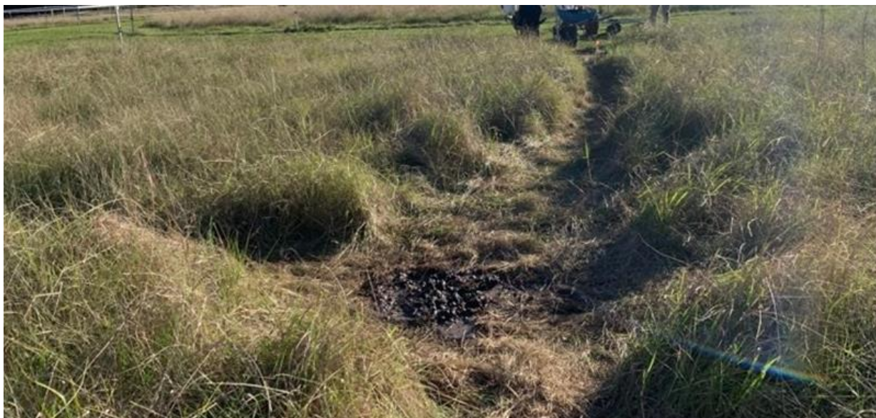
Photo 2-3 Example test pit after dry weather following backfill with wet sieving spoil and imported sand
