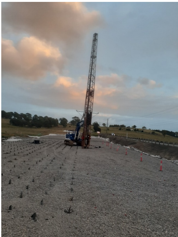
View of installation of wick drains – December 2020
