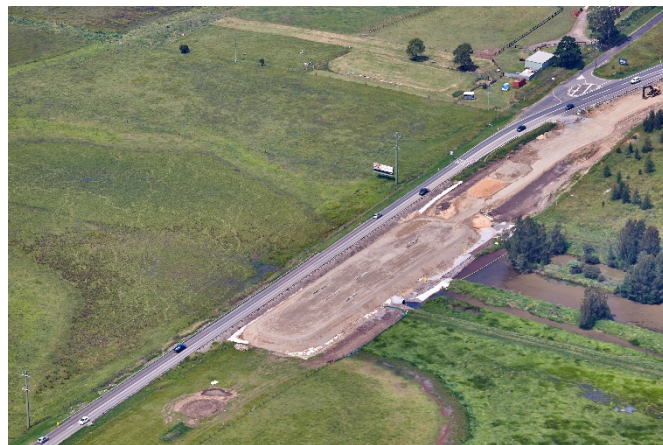
Aerial view of imported fill for preload embankment – February 2021
