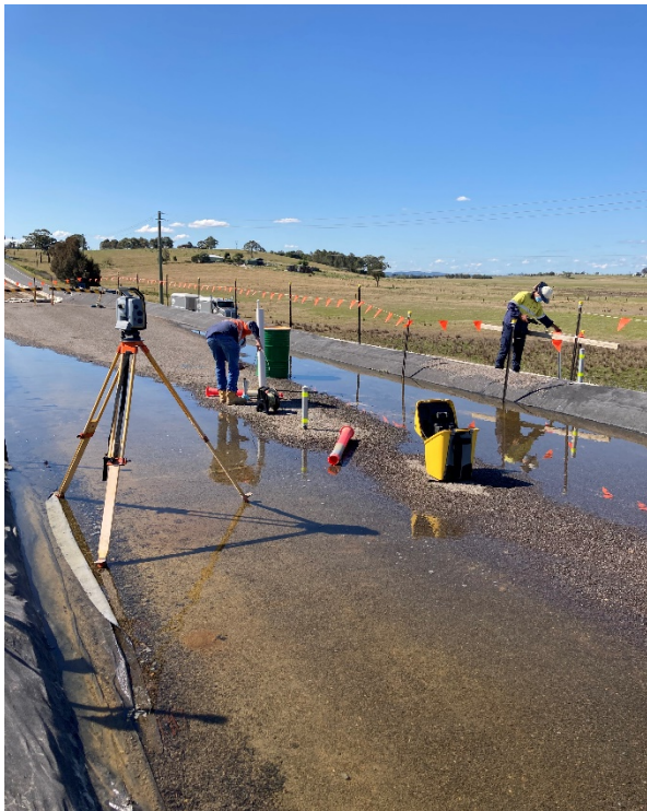
Weekly geotechnical monitoring was completed during the consolidation period
