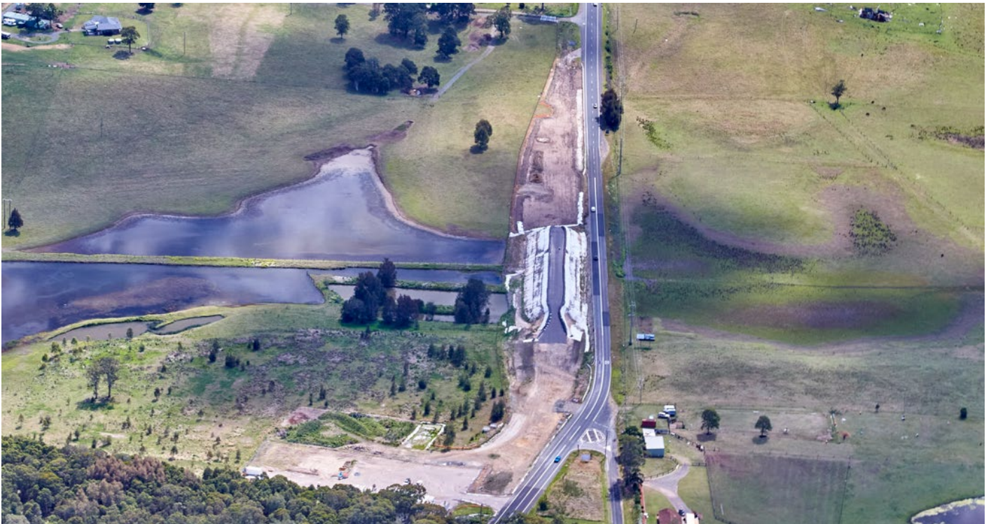
Aerial view of Main Road, looking north – October 2021
