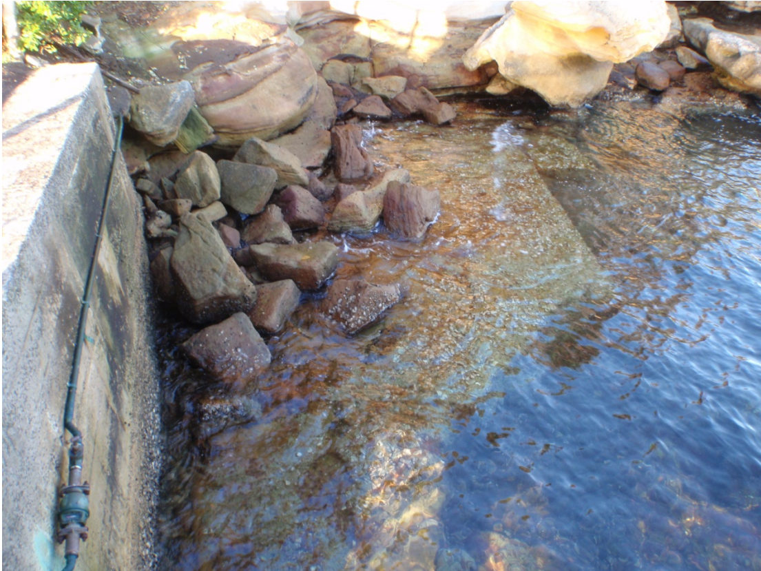
Figure 8 South side of wharf showing concrete and sandstone seawall with a natural rocky shore beyond.
