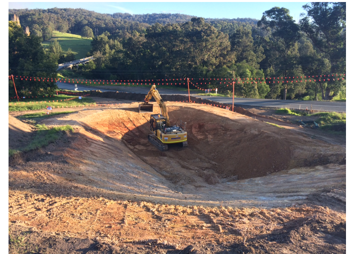
Construction of a sediment basin north of the Dignams Creek Bridge
