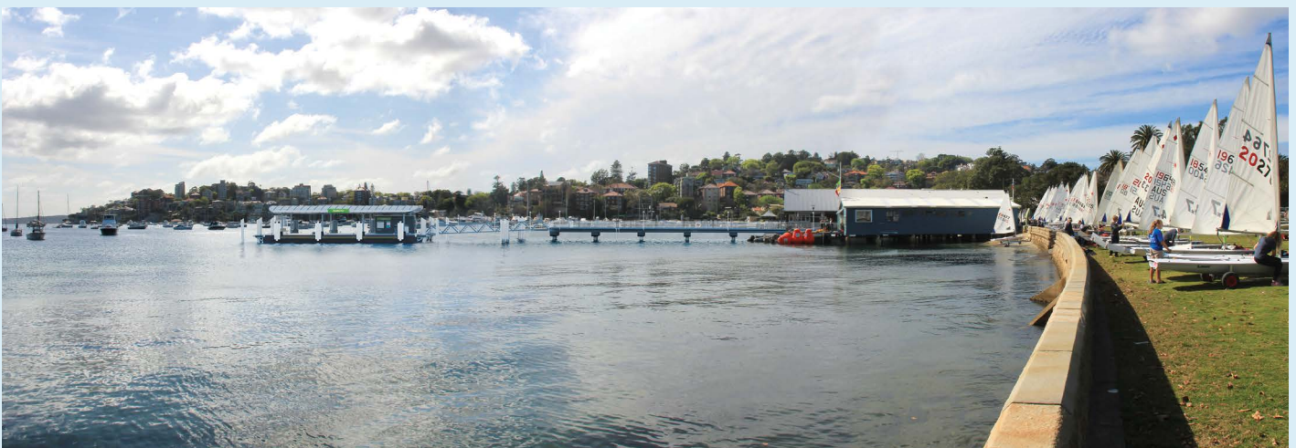
Pictured: An artist's impression of the Double Bay Wharf Upgrade, view from foreshore looking east
