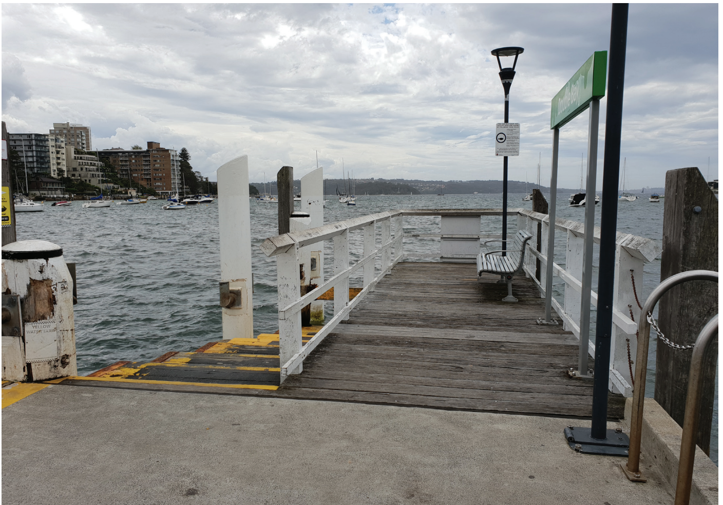
The existing Double Bay Wharf.
