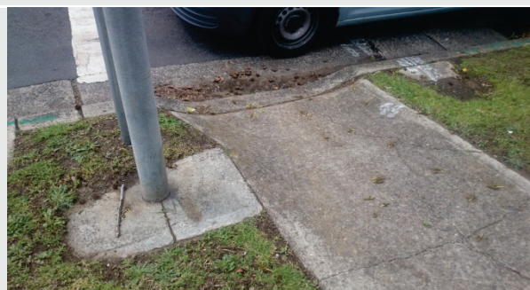
Southern approach – footpath leads to carriageway and ramps do not align
