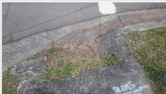
Damaged footpath on northern approach, east of Essex Street
