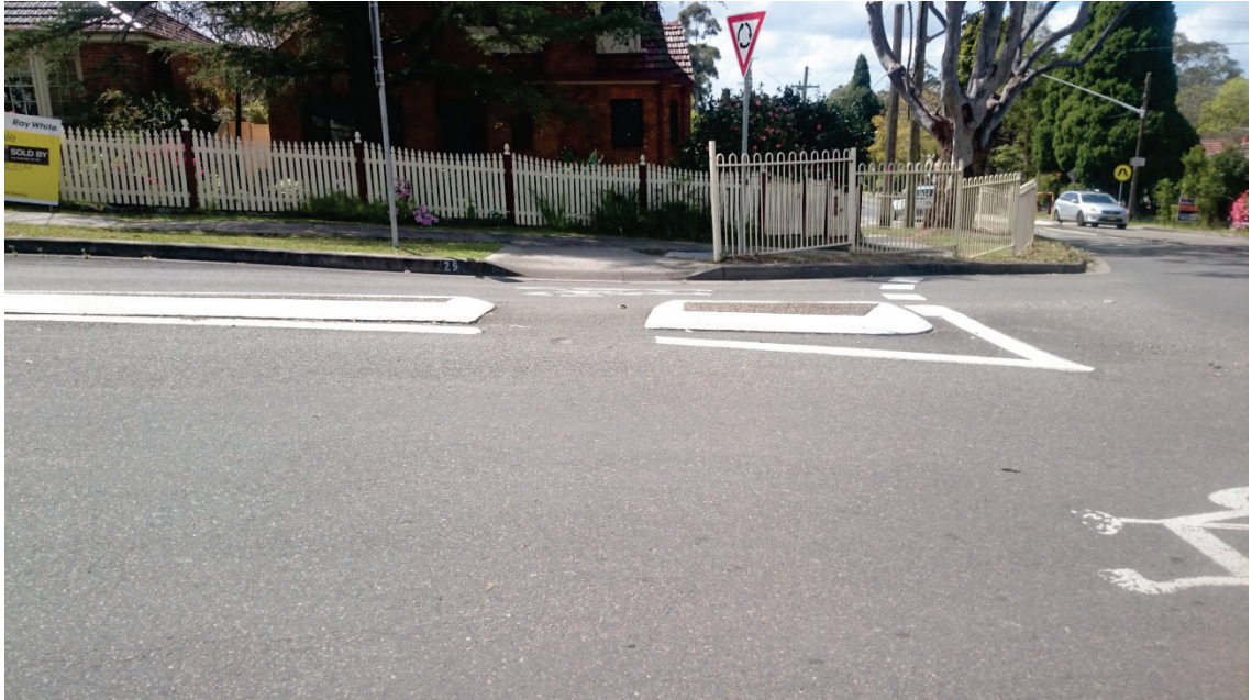
Photo 1 North approach pedestrian refuge island and fencing
