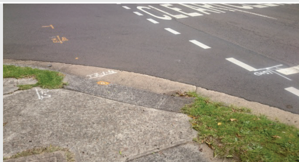
Pedestrian ramps not aligned correctly
