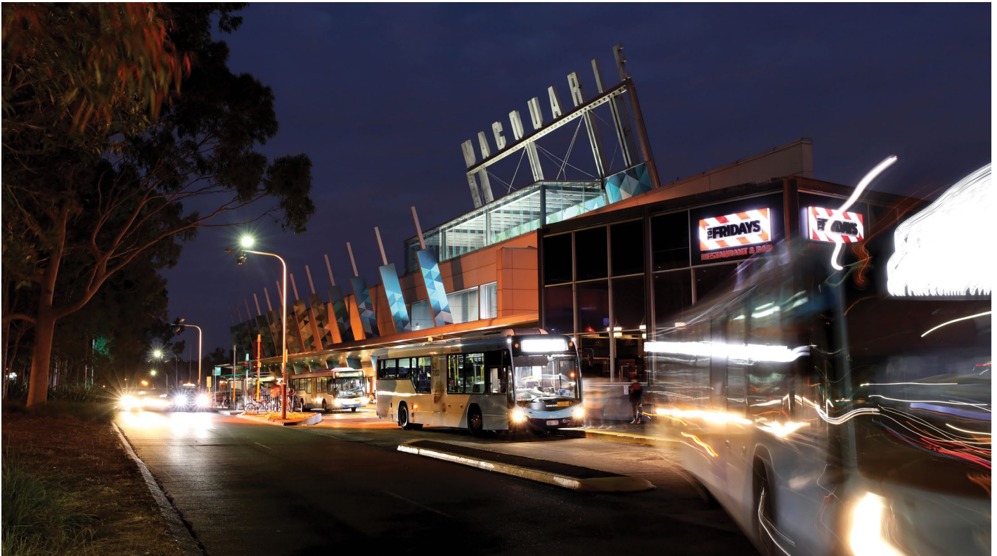
Macquarie Park bus interchange
