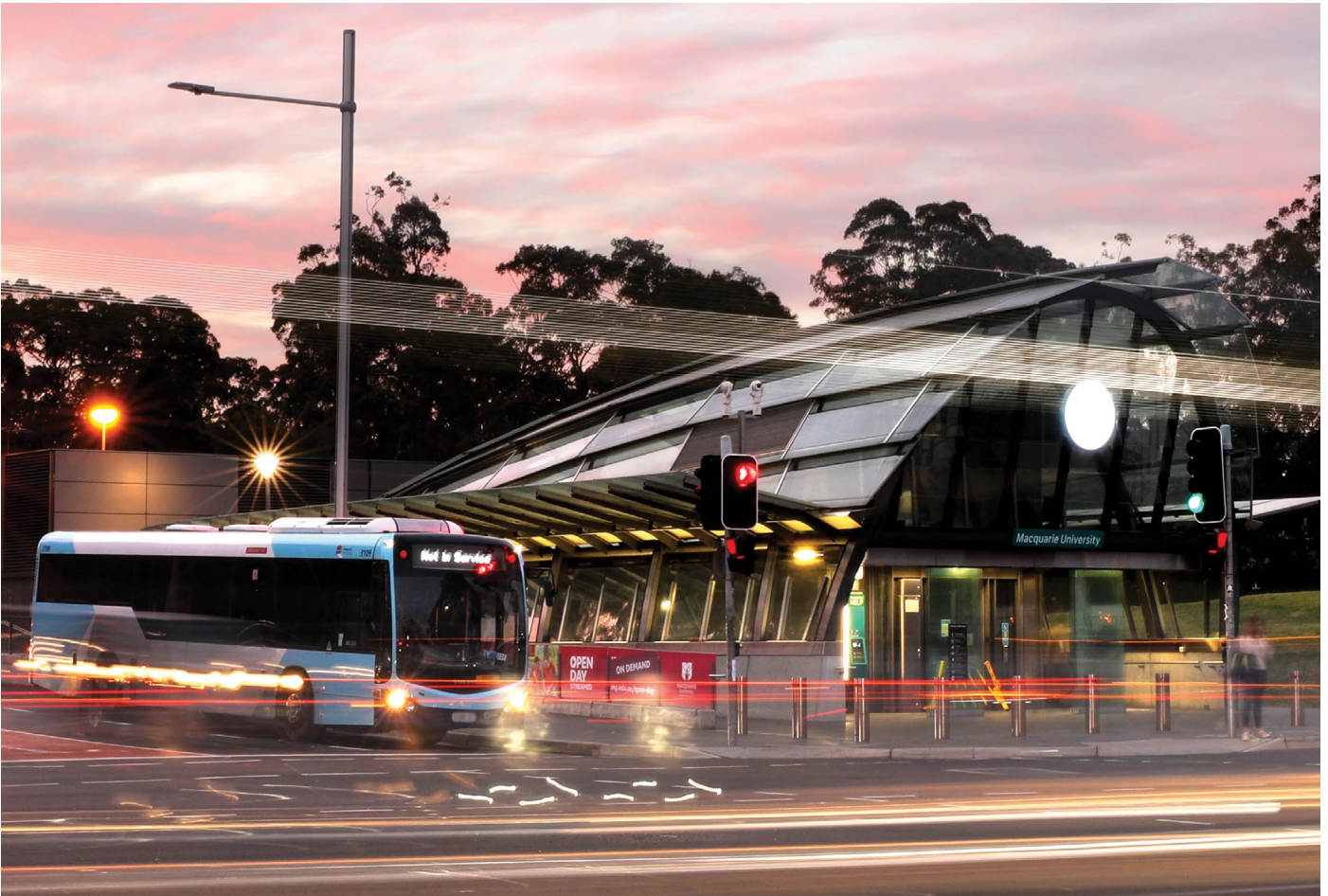
Macquarie University Metro Station on the intersection of Herring Road and Waterloo Road
