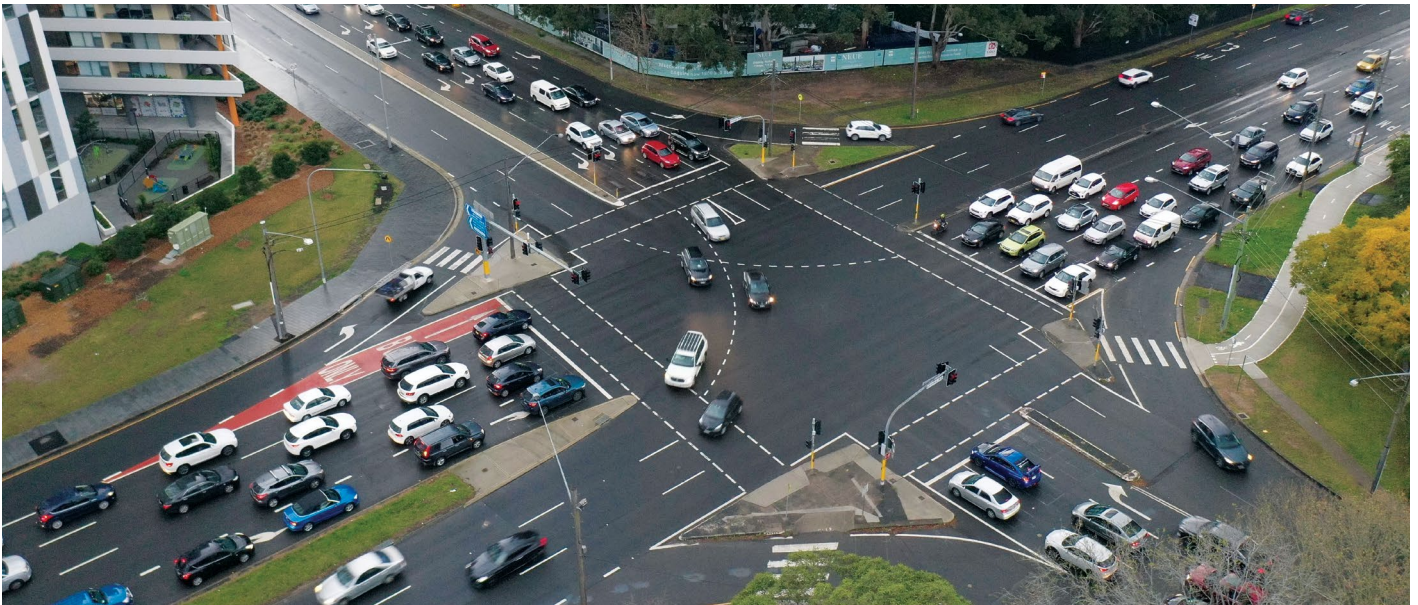
Congestion at the Herring Road and Epping Road intersection in Macquarie Park
