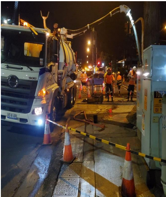
Macquarie Park night works – November 2022
