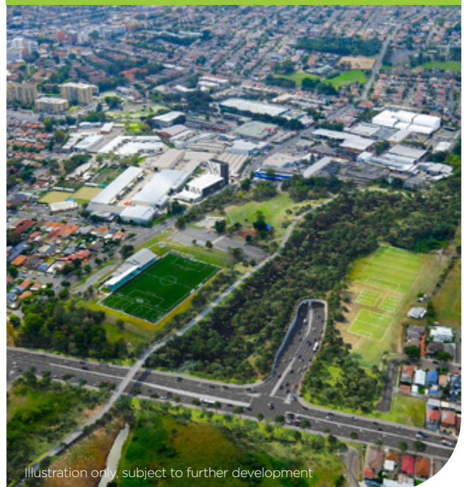
Entry and exit ramps of the F6 Extension Stage 1 tunnels at President Avenue, Kogarah.
