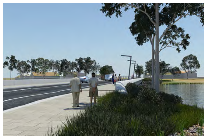
Figure 4.10 The parapet is terminated through a gentle transition back into the ground, creating a fluid end to the bridge.
