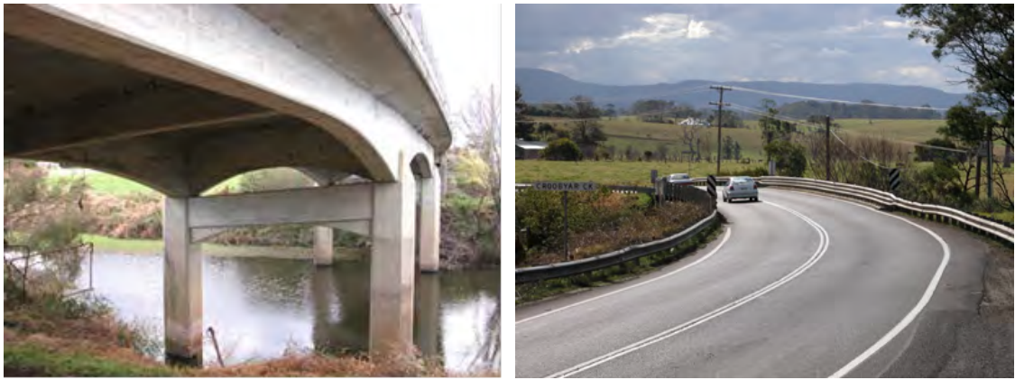
Figure 4-3 Croobyar Creek Bridge curved deck (Source: BRW)
