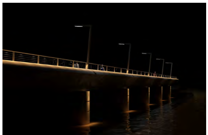
Figure 4.6 Feature lighting to accentuate the parapet would be incorporated within the handrail.
