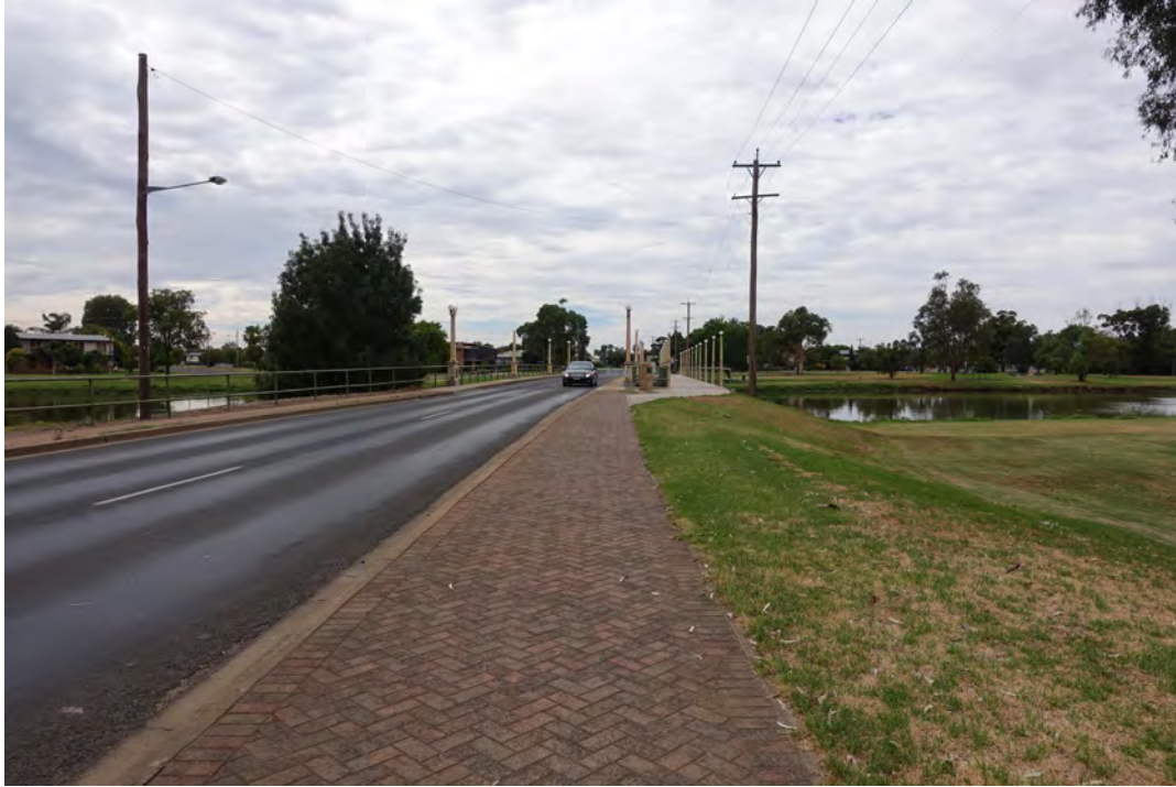
Figure 4.13 Existing situation looking towards the bridge approach with Camp Hill in the background.
