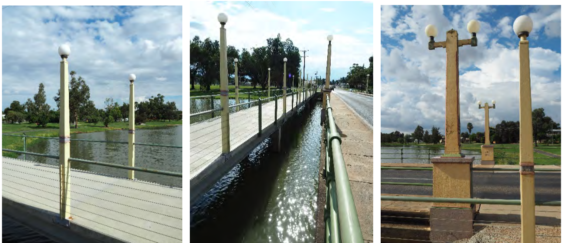
Figure 7-9 New pedestrian bridge lamp posts (Source: FBE)
