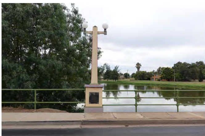
Figure 4.8 The existing light poles would be recycled as part of the approaches to the new bridge.
