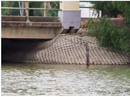
Figure 7-1 Abutment section (Source: FBE)
