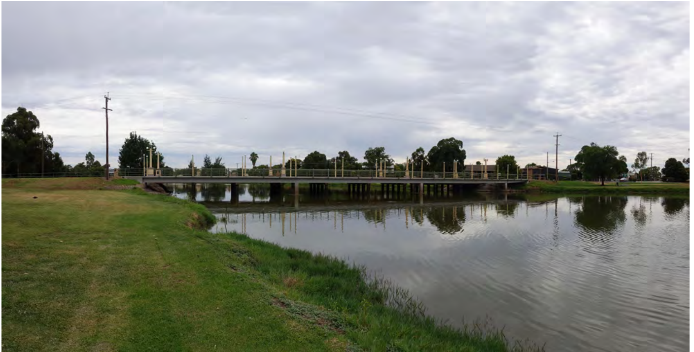
Figure 4.15 Existing situation looking east from the foreshore of Lake Forbes.
