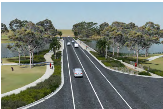
Figure 4.7 Feature pavers would be used for the shared use path and landscaped areas introduced at the approaches to the bridge.
