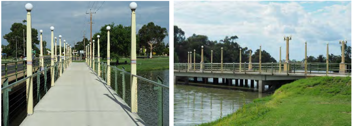
Figure 7-8 New pedestrian bridge (Source: FBE)
