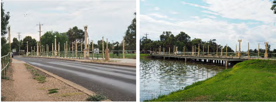
Figure 2-1 Camp Street Bridge (Source: FBE)
