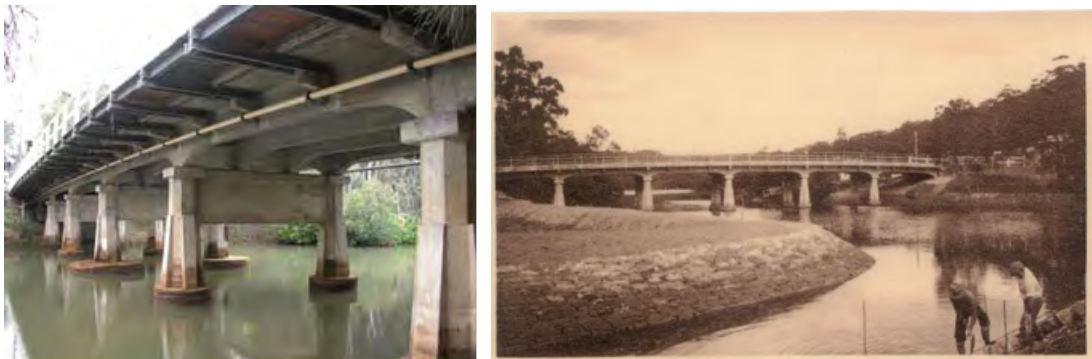
Figure 4-2 Fullers Bridge across Lane Cove River (Source: BRW)
