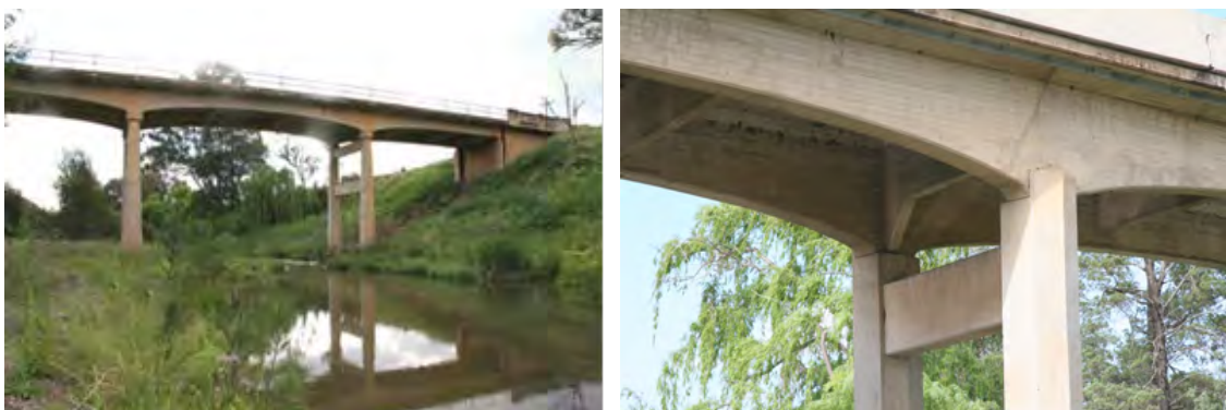
Figure 4-4 Manilla Bridge in Western Region curved deck (Source: BRW)
