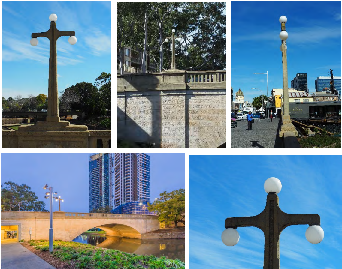
Figure 12-6 Lennox Bridge, Parramatta (Source: RMS)
