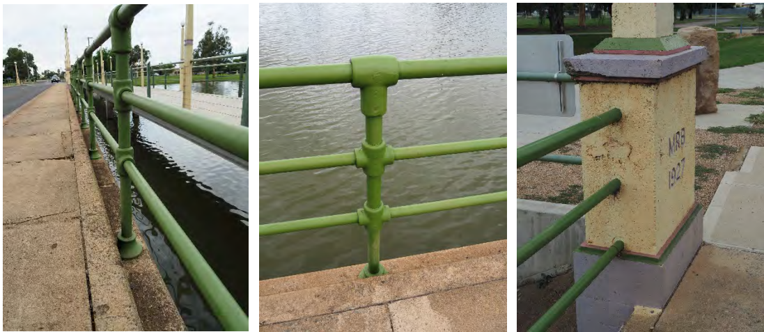
Figure 7-4 Pedestrian balustrade railing (Source: FBE)
