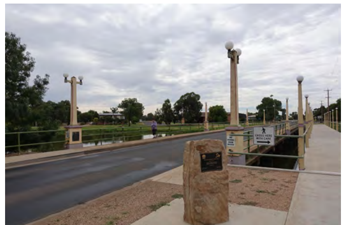
Figure 2.9 The original bridge to the left. The walkway to the right was recently added to provide better pedestrian amenity.
