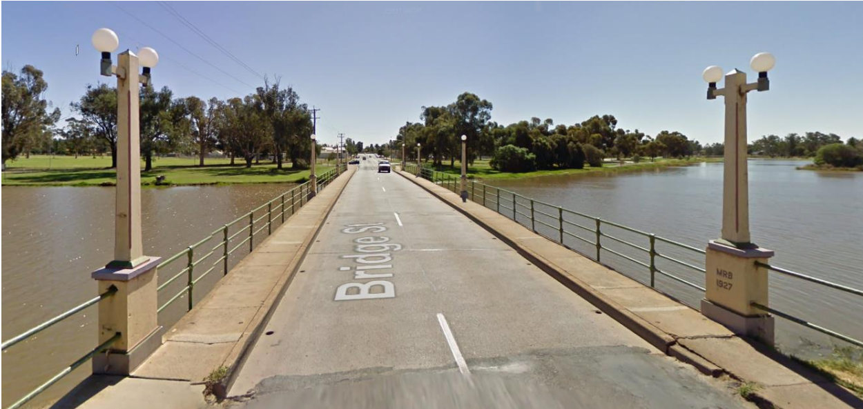
Figure 2-2: Camp Street Bridge showing art deco light fixtures
