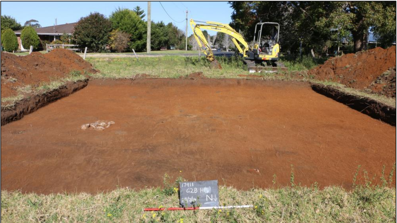
Plate 17: South facing post-excitation photograph of G2B H11 - East with 1 m scale, [005] and (006) is clearly visible (Source: Biosis, 2014).
