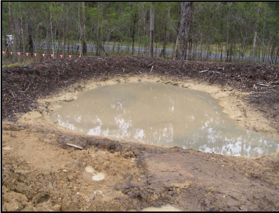
Plate 12: Mulch used as a bund for a temporary sedimentation catch dam. Mulch is effective as it can provide both containment and filtering of site water. Mulch should not be used as a control in areas of concentrated flow where it may be washed away. Any mulch containment control should have a defined and lined outlet that allows discharge from the control without washing mulch away. Note that this control does not have a defined discharge outlet which should be installed to prevent failure of the control in heavy rainfall events.
