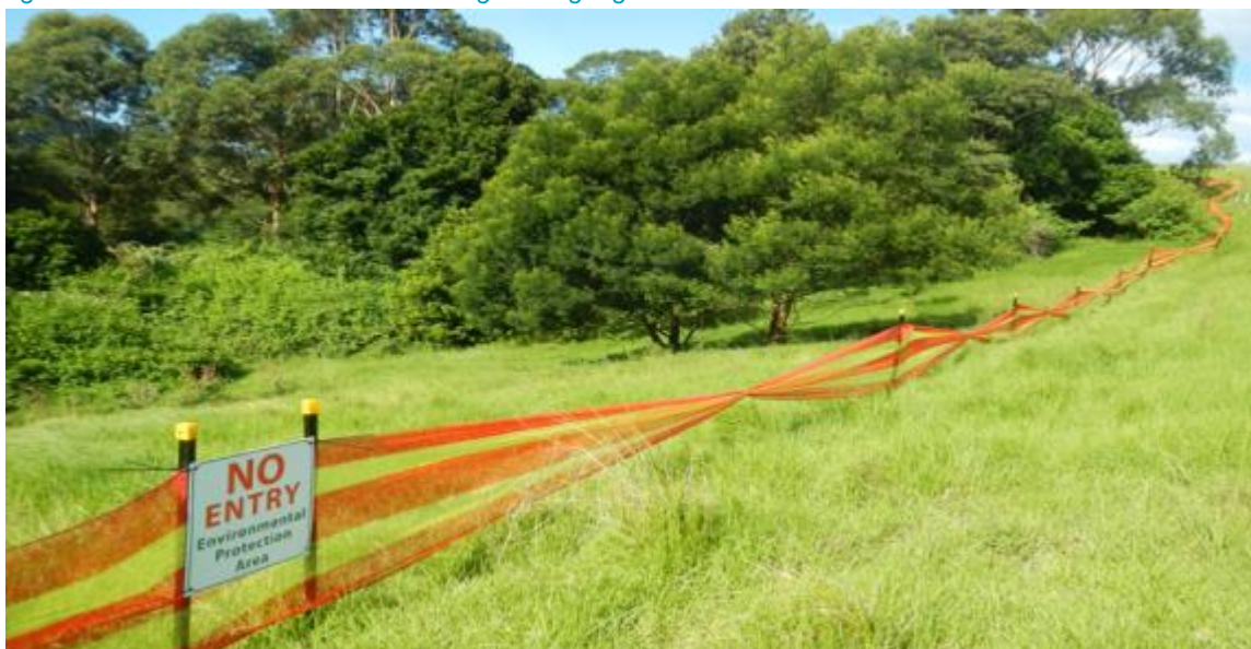
Figure 3-1: Installed sensitive area fencing and signage
