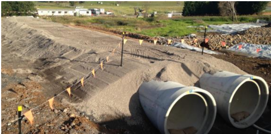
Figure 3-2 :Transverse drainage works at Austral Park Road realignment.
