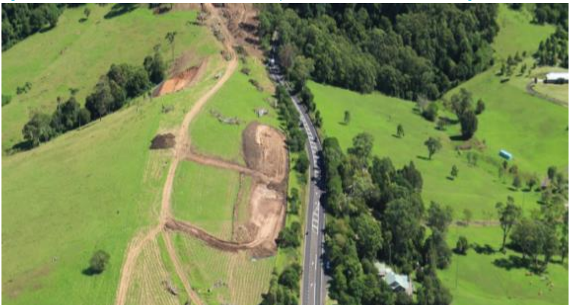
Figure 3-4: Construction of sediment basins in Cut 1, prior to bulk earthworks commencing.
