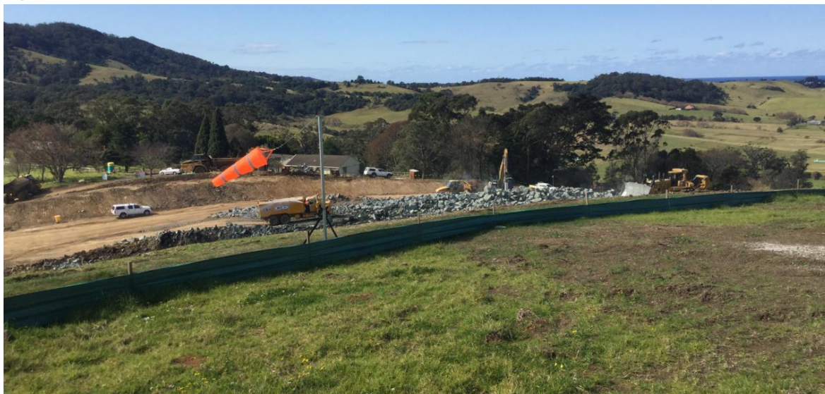
Figure 5-: Wind-sock installed as a visual indicator to plant operators of the direction and velocity of winds
