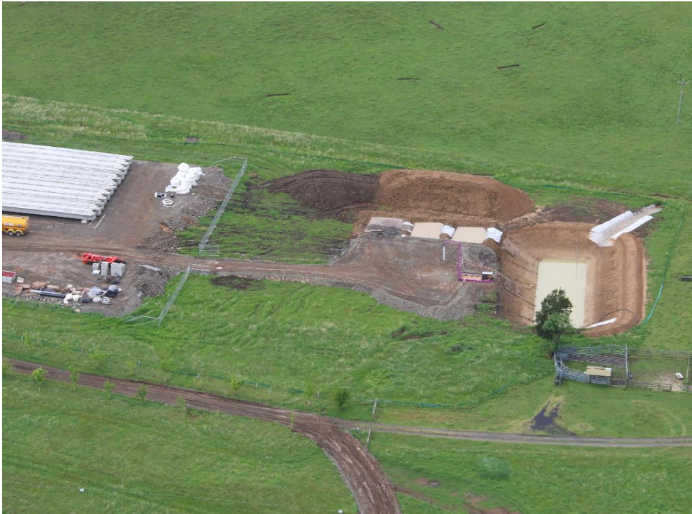
Figure 2-3: Construction of sediment basins at Austral Park stockpile site
