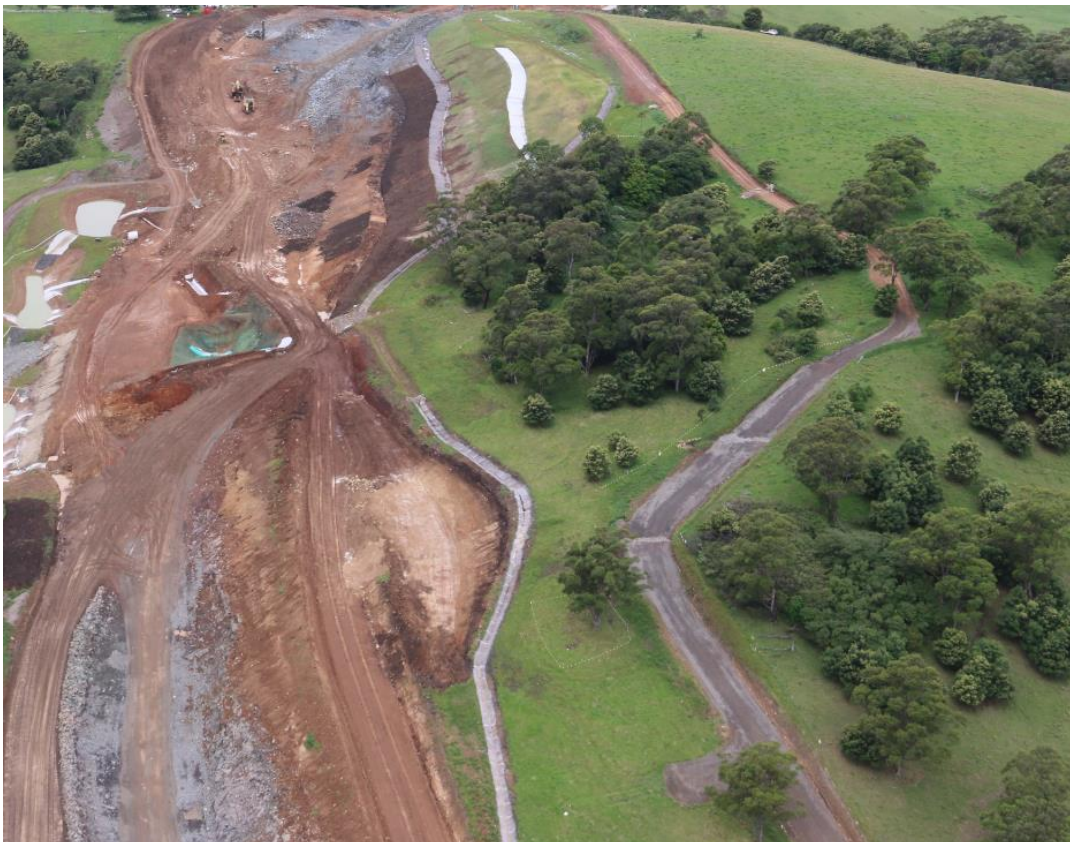
Figure 2-6: Light vehicle access track avoiding trees and separating light vehicles from heavy plant in cut 2
