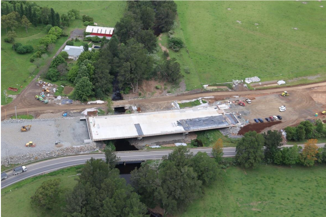
Figure 2-6: Light vehicle access track avoiding trees and separating light vehicles from heavy plant in cut 2
