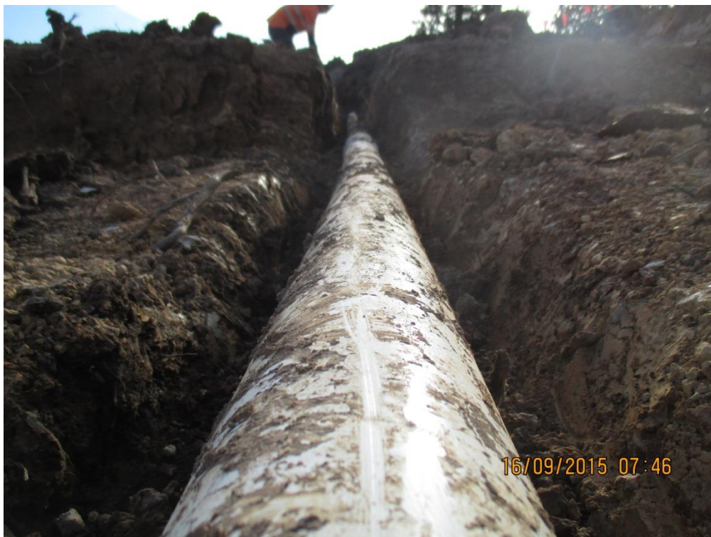
Figure 2-1: Services installed underground across the project
