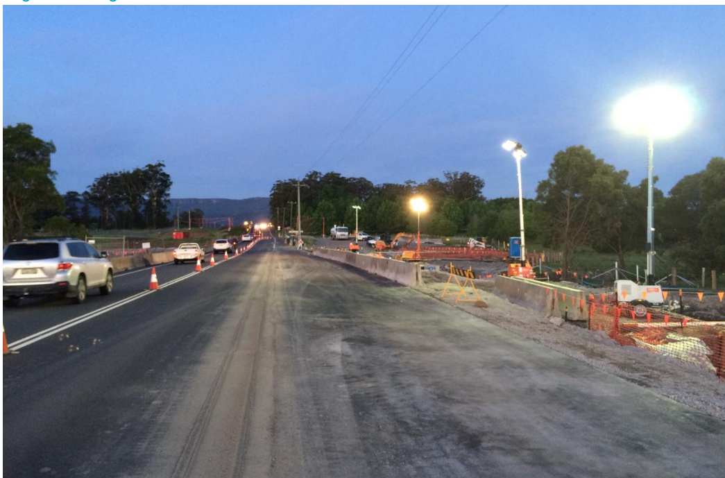
Figure 2-2: Night works for SB11
