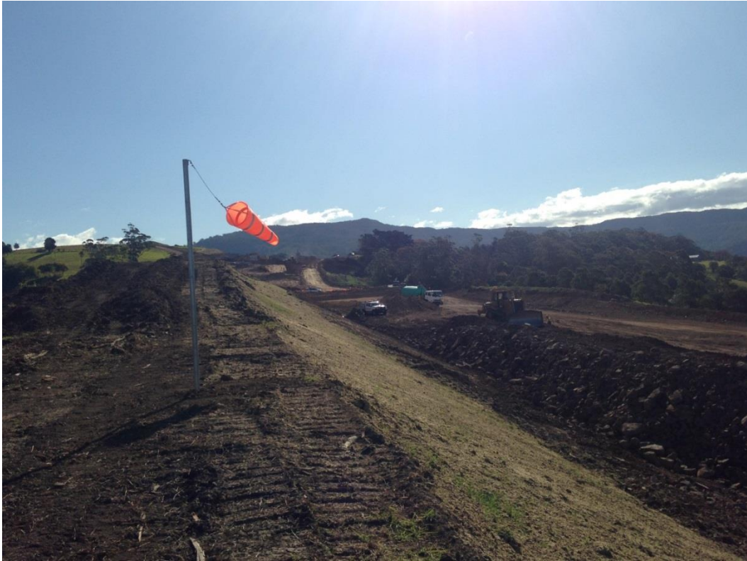
Figure 5-4: Visual wind socks give operators an indication of wind speed and direction.
