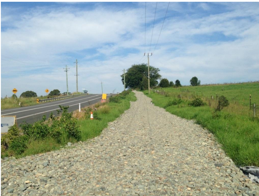
Figure 2-6: Temporary access track to enable power line relocations.
