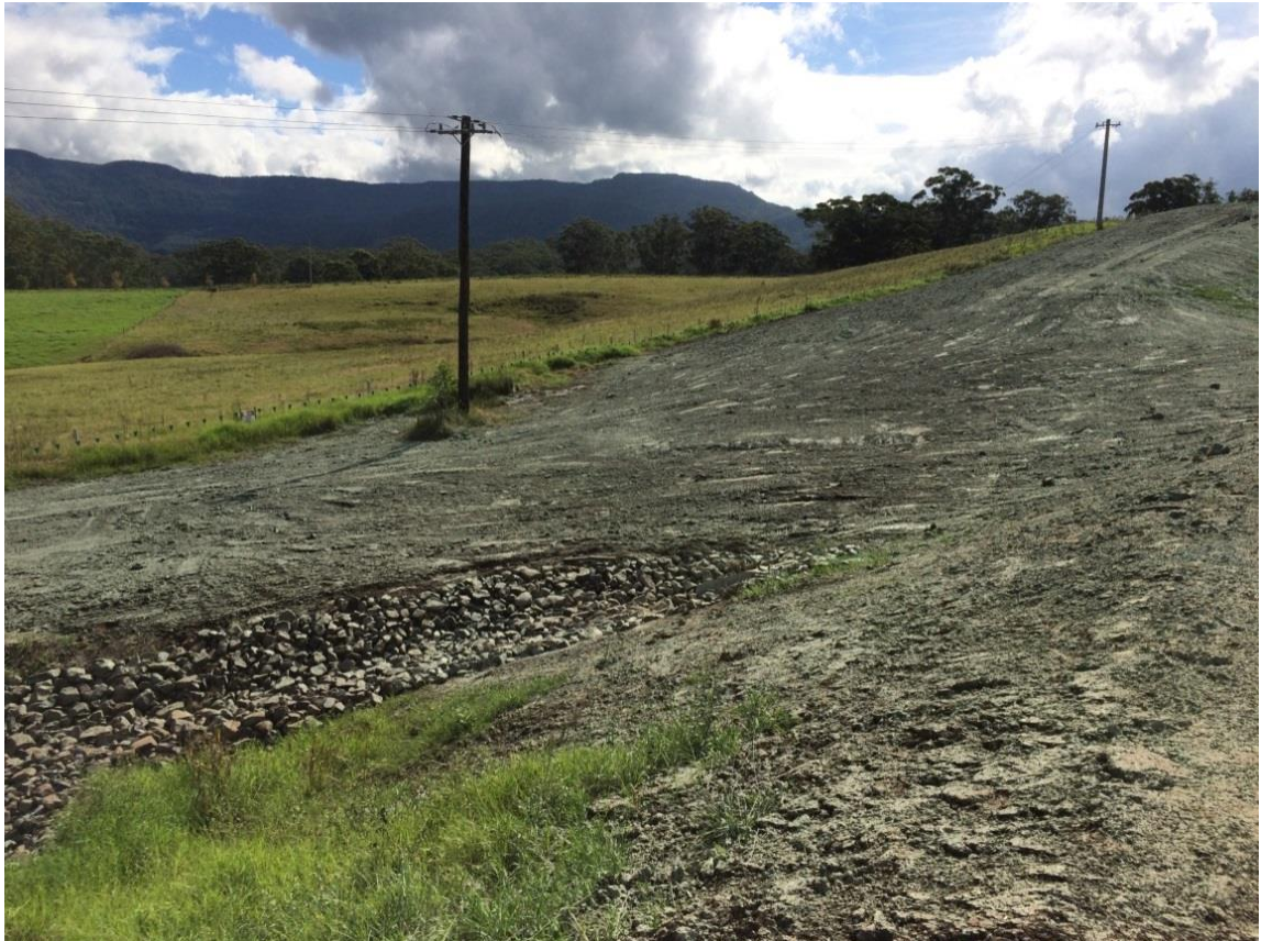
Figure 2-4: Rehabilitated area where a sediment basin was located.
