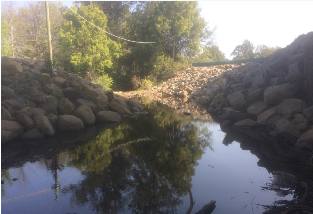
Figure 2-6: Removal of the temporary bridge structure crossing Broughton Mill Creek completed
