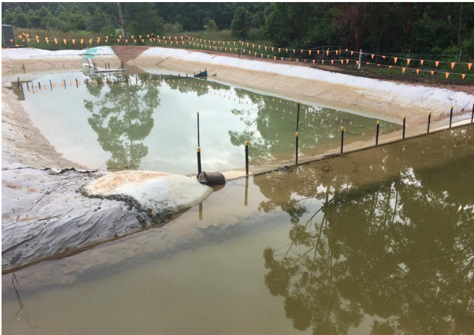
Figure 4-2: HES Basin looking from the fore-bay across the spreader bar and down to the decanting system after rain event
