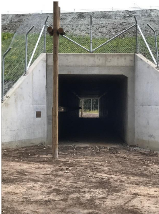
Figure 4-3: Fauna furniture installation at SC04
