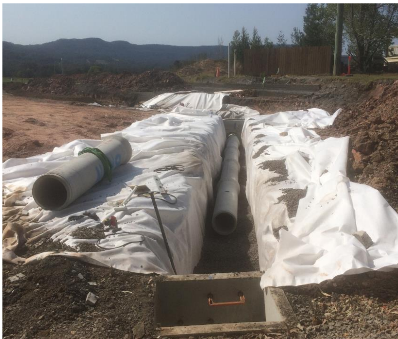
Figure 2-1: Final drainage on the project being installed at Queen St roundabout
