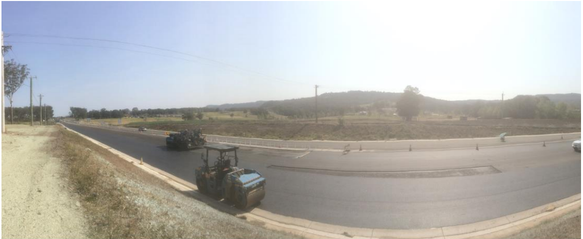
Figure 2-3: Final wearing coarse pavement being placed in cut 9 to cut 12
