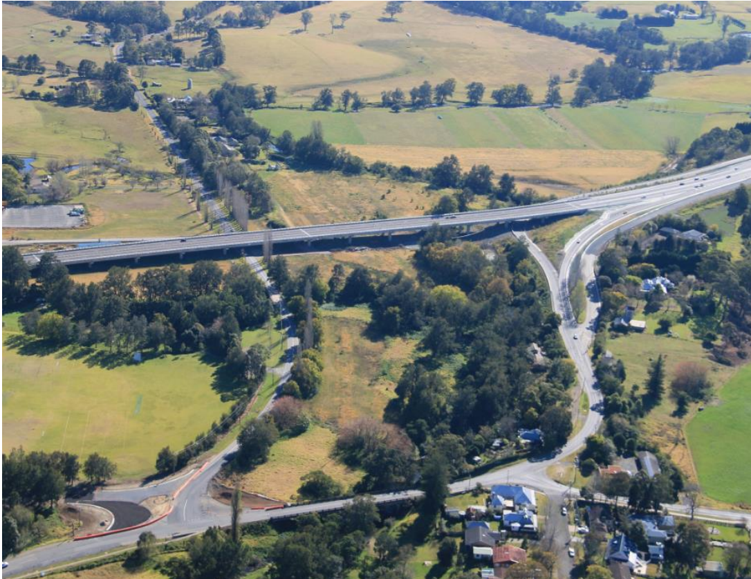
Figure 2-2: Berry Bridge open to traffic in both northbound and southbound lanes
