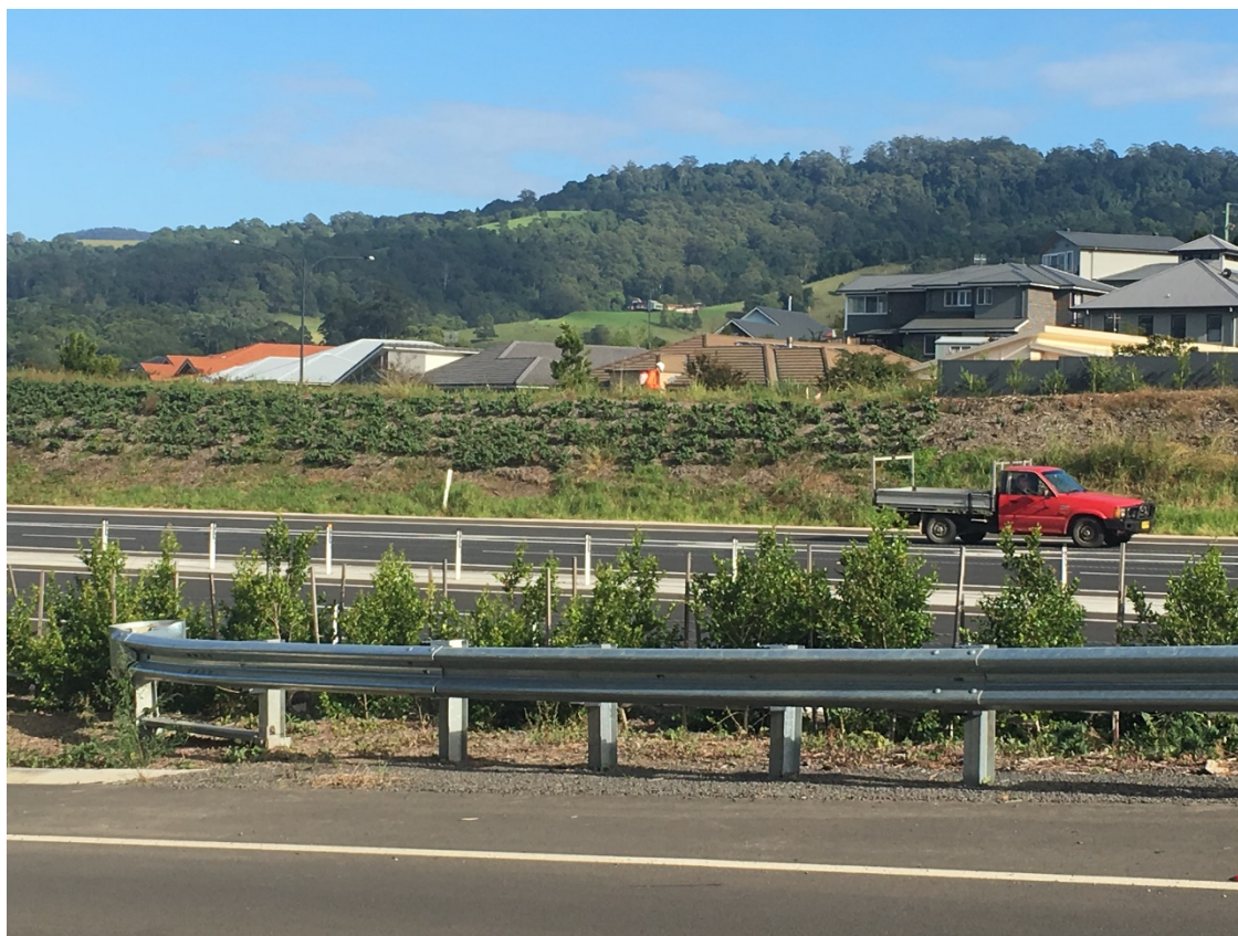
Figure 2-4: Landscape maintenance of the garden beds south of the southern Berry interchange
