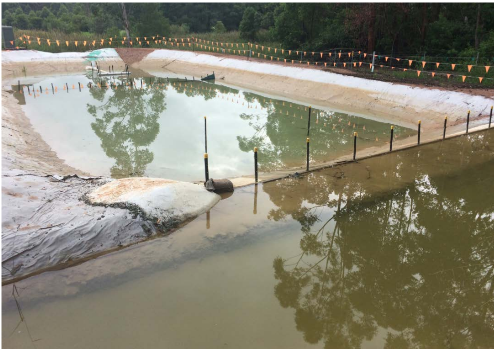
Figure 4-2: HES Basin looking from the fore-bay across the spreader bar and down to the decanting system after rain event
