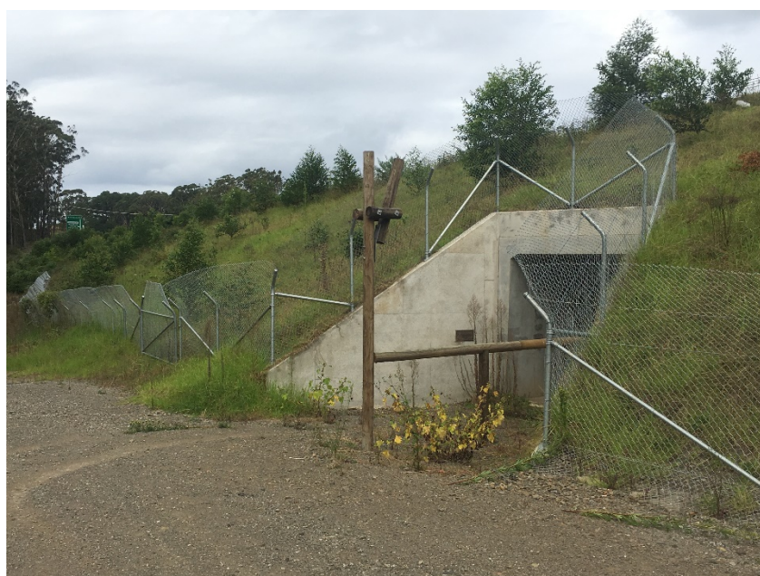
Figure 2-1: Fauna underpass complete with fauna furniture
