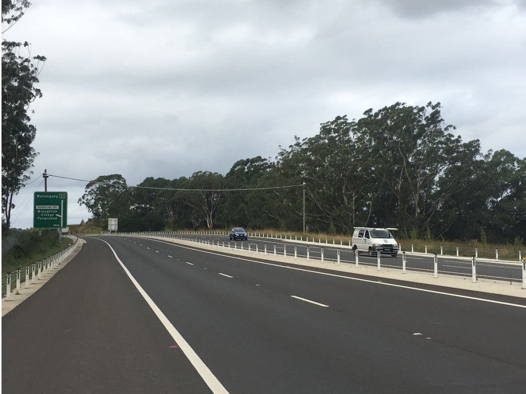
Figure 4-3: Rope bridge complete
