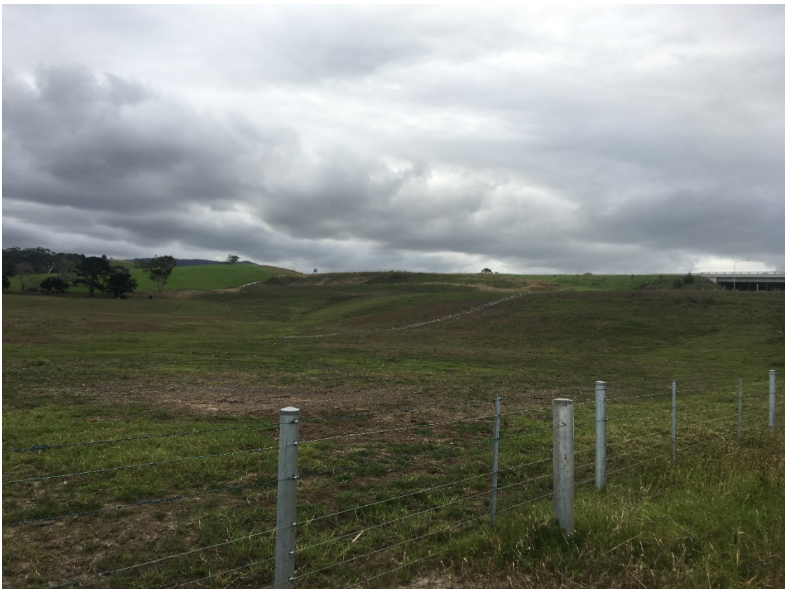
Figure 2-6: Rehabilitation of Toolijooa ancillary facility complete
