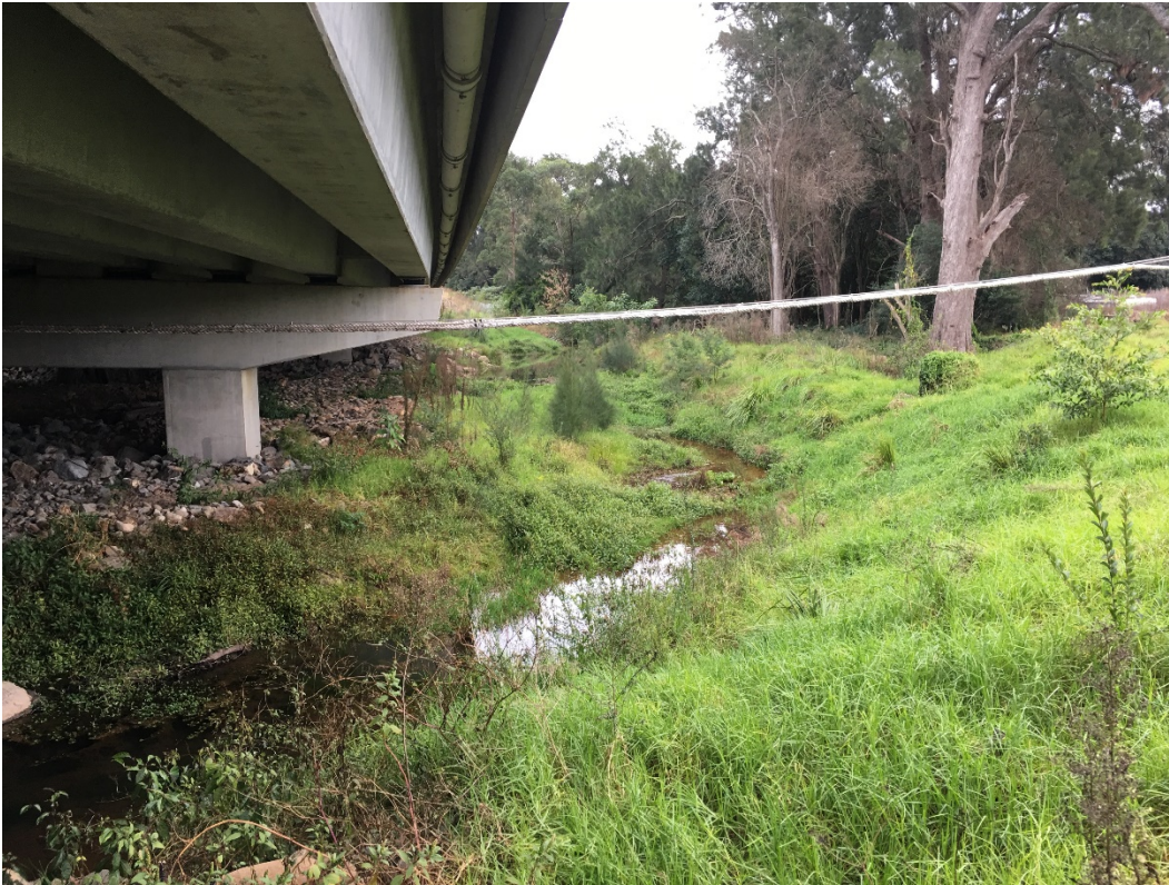
SW06 – Bundewallah Creek, upstream of works
