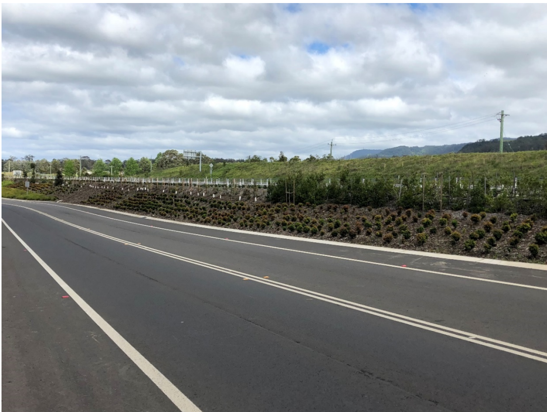
Figure 2-3: Landscape maintenance of the garden beds south of the southern Berry interchange
