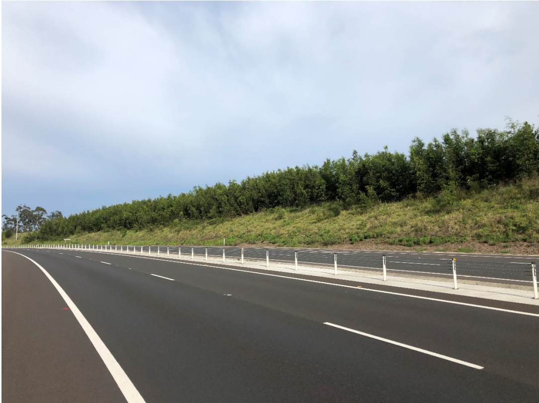
Figure 2-2: Permanent landscaping of Cut 6
