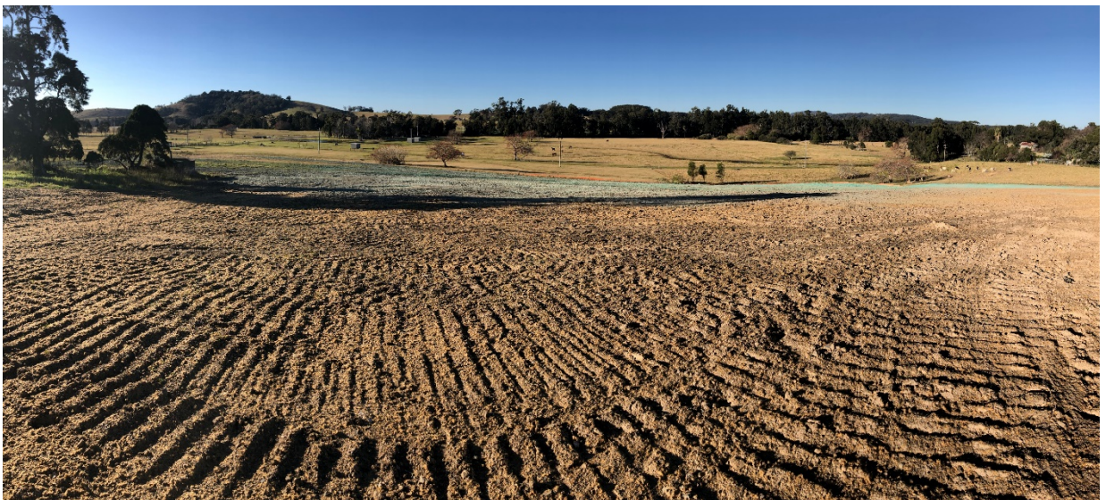
Figure 2-7: Rehabilitation of Austral Park ancillary facility
