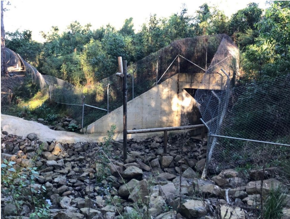
Figure 2-1: Combined fauna underpass and drainage culvert complete with fauna furniture
