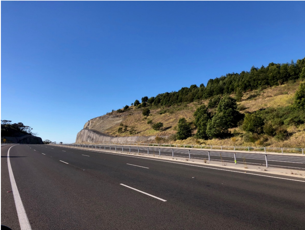
Figure 2-4: Permanent landscaping of Cut 2
