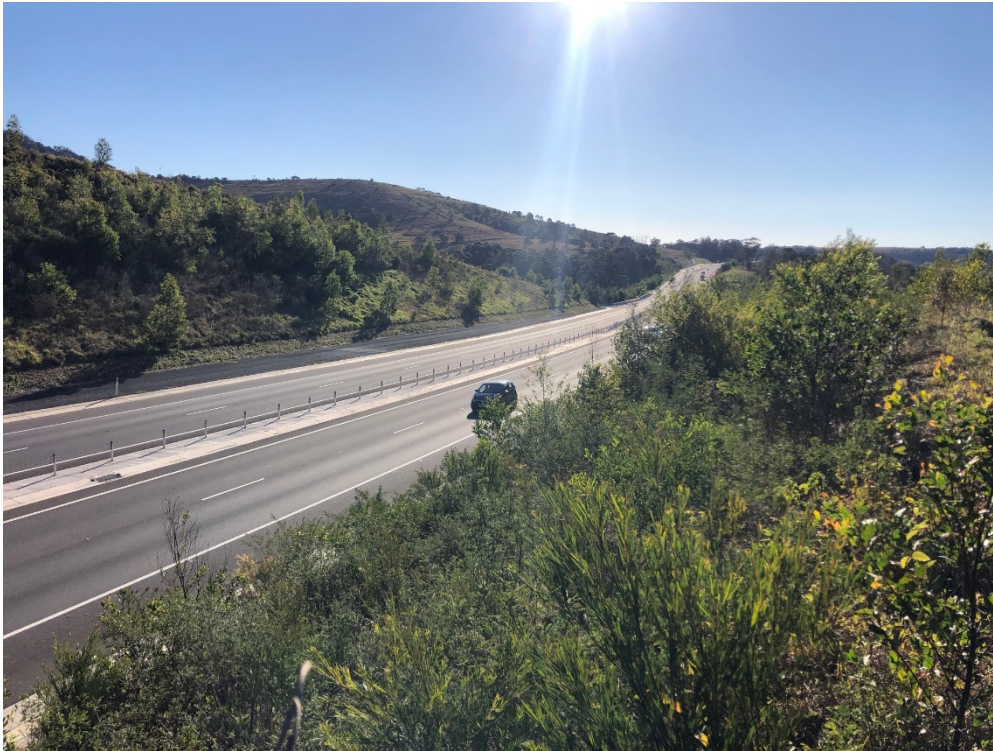
Figure 2-3: Permanent landscaping of Cut 5
