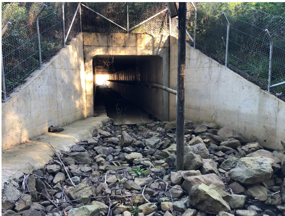
Figure 5-1: Fauna underpass complete
