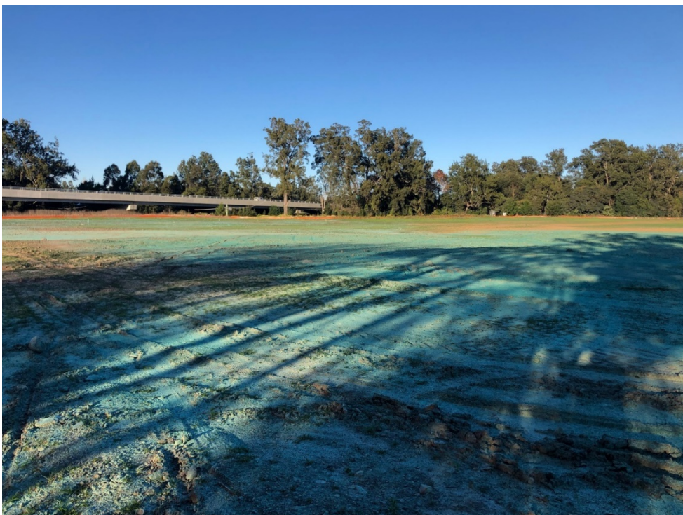
Figure 2-2: Woodhill Mountain Road Compound decommissioned
