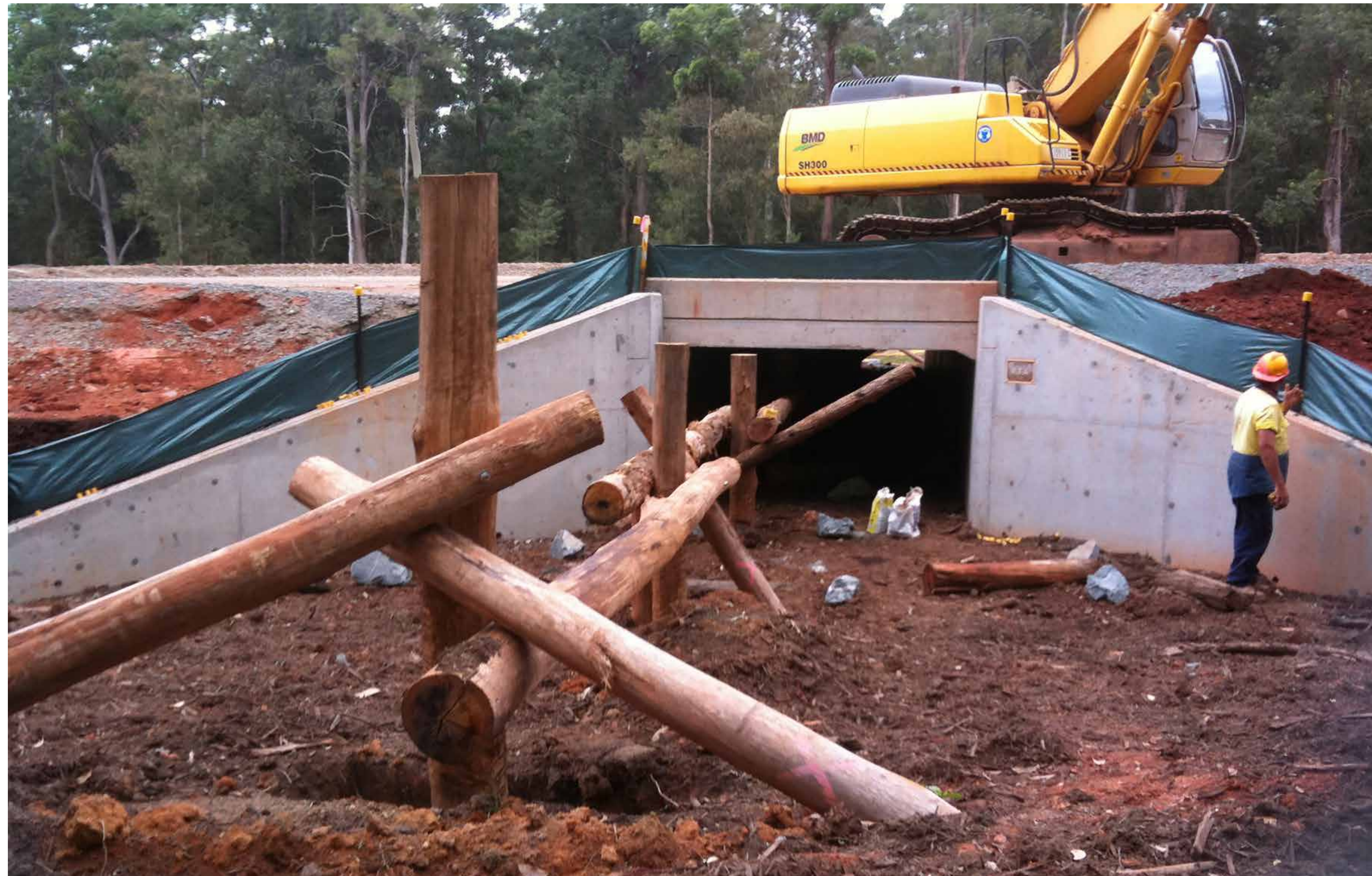
Indicative culvert style underpass
