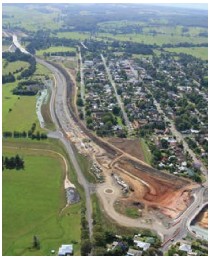
New highway being built adjacent to North Street looking north
