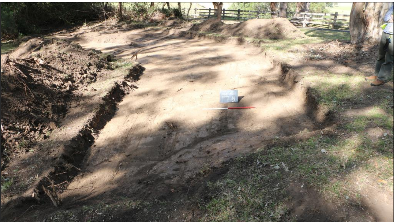
Plate 32: North facing post excavation photograph of G2B H53, 1 m scale (Source: Biosis, 2014).
