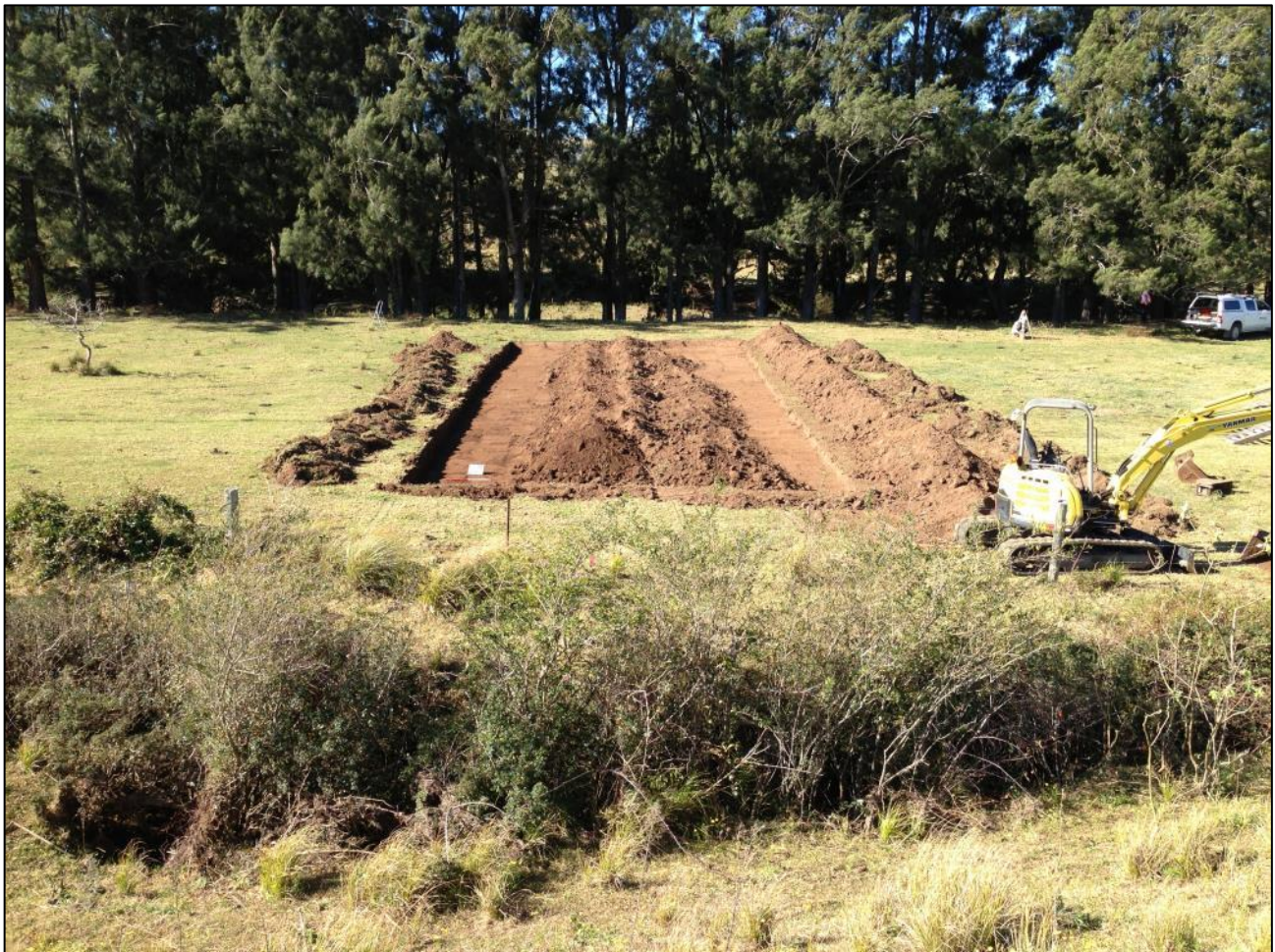
Plate 22: East facing photograph of G2B H28 showing entire stripped area (Source: Biosis, 2014)
