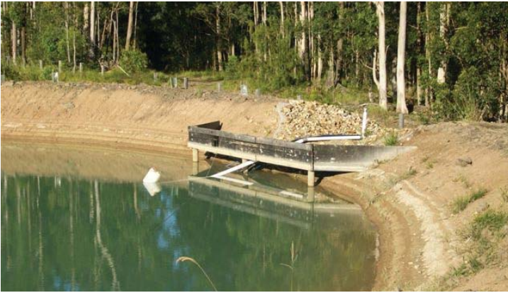
Figure 5. A siphon and float system used for discharging a basin without use of pumps. Floats may be useful for preventing inlets from falling into sediment zones.
