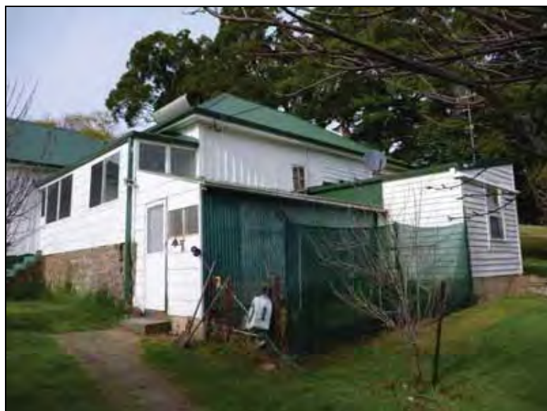
Figure G.101 View of back (northwest facing) portion of homestead, showing veranda infill and skillion additions, looking S
