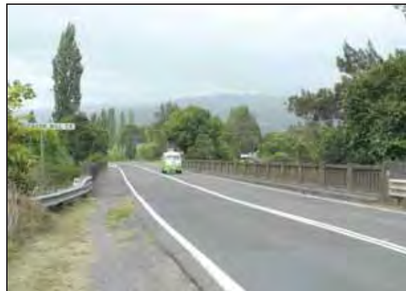
Bridge (constructed 1955) over Broughton Mill Creek, Berry
