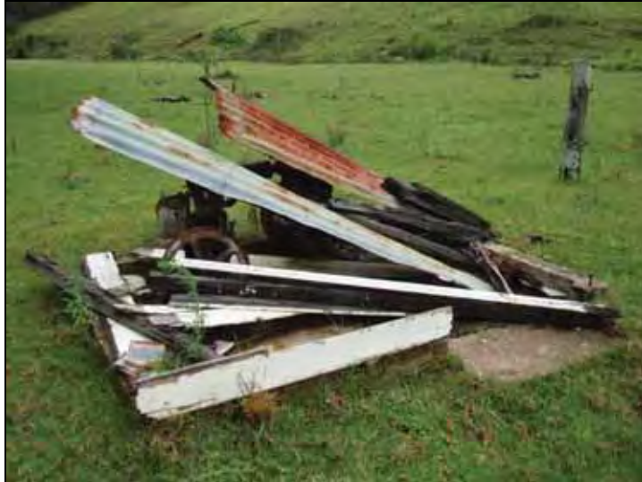
Figure G.133 Remains of a water pump and shed at the edge of a former orchard area (behind pump), looking SW
