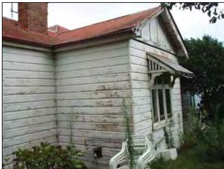
Figure G.164 View of Federation style extension at SW corner of building
