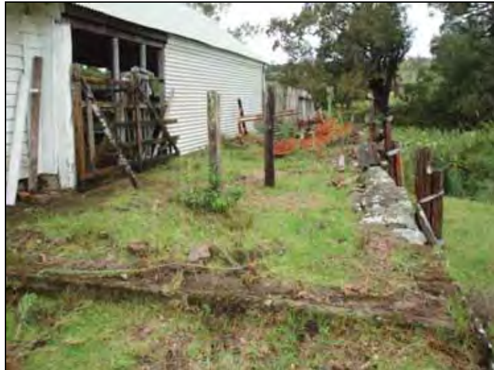
Figure G.130 earth platform behind (south of) storage shed, with cement footings, drains, in situ poles and sandstone retaining wall, probably indicative of a former dairy complex, looking E
