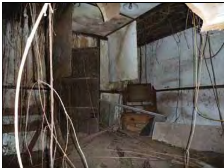
Figure G.177 Interior view of north eastern room
