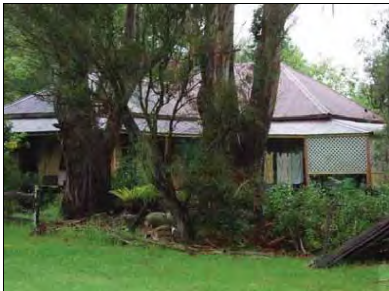
Figure G.144 Detail of southern side of homestead, looking NE
