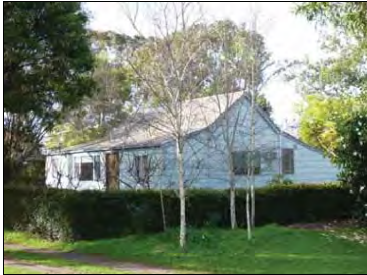
Figure G.65 General view of house, looking SE
