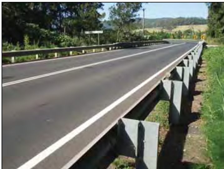
Figure G.139 General view of road top and approaches to bridge, looking NE
