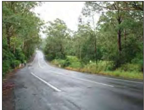
Highway alignment west of Glenvale
