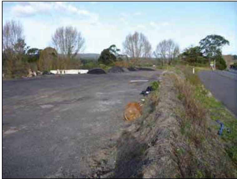
Figure G.53 View of the G2B H24 area, looking SW, note filling and levelling across site
