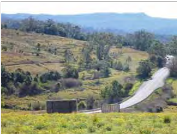
Highway alignment at the 'Big Dipper', Broughton Village
