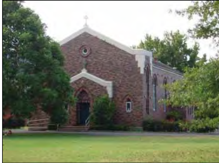
Figure G.152 Front view of St Patrick's Church, looking N
