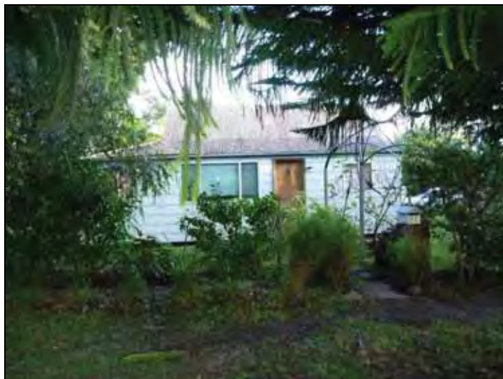
Figure G.67 Detail of front of house, looking S
