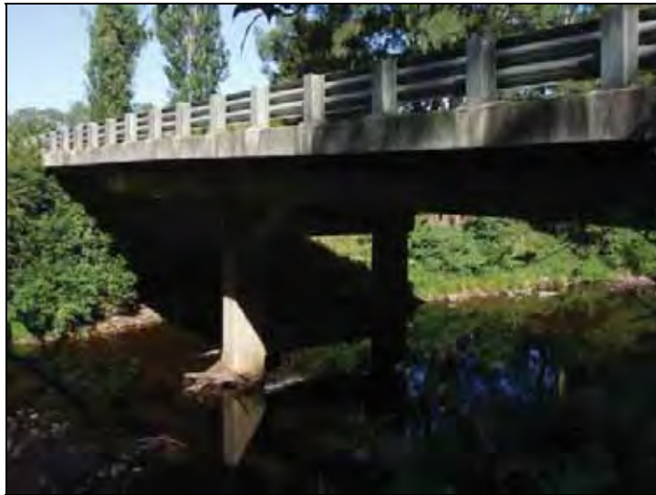
Figure G.137 General view of bridge from upstream west bank
