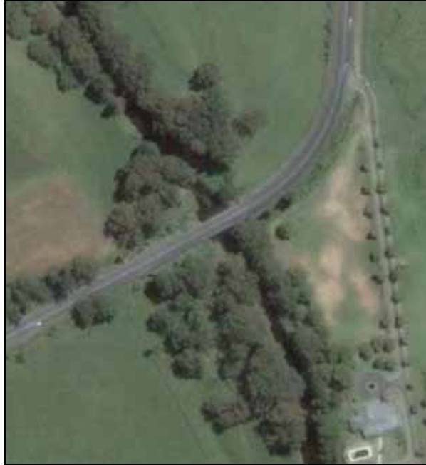
Figure G.140 Aerial image (2007) of bridge (Google Earth Pro 2011)
