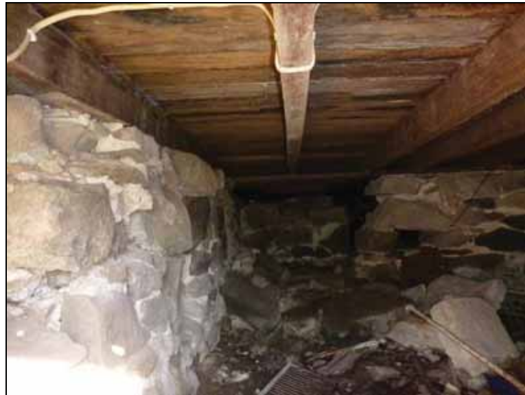
Figure G.106 Rough sandstone wall foundations under original portion of homestead
