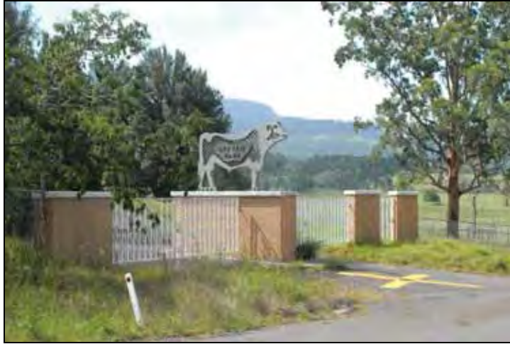
Figure G.168 General view of entrance to Graham Park (2007 image)
