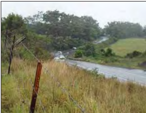
Highway alignment west of Sedgeford
