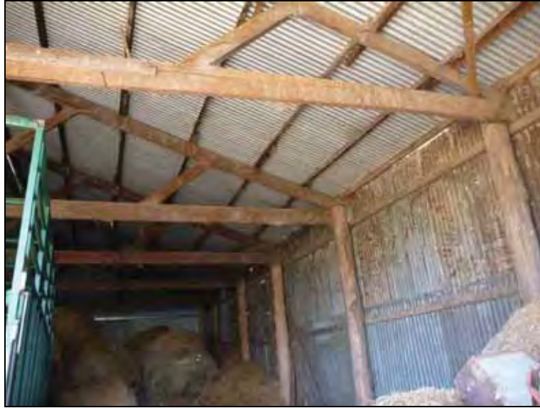
Figure G.111 Detail of internal wooden frame in downslope shed
