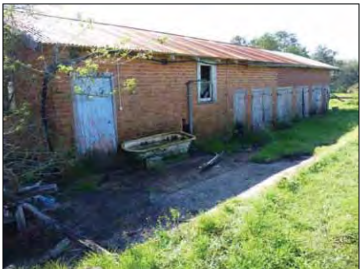
Figure G.180 Southern side of disused dairy, looking NE
