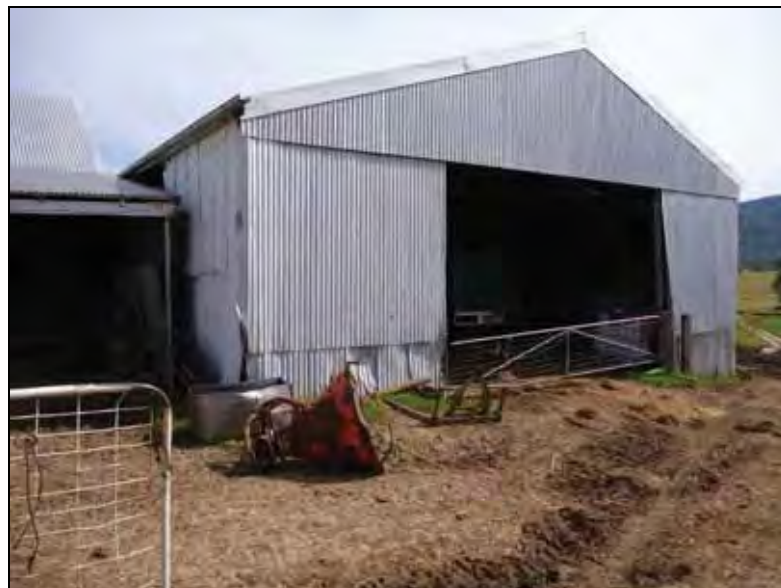
Figure G.110 Front of downslope shed, built using components from a Port Kembla shed used for processing immigrant workers
