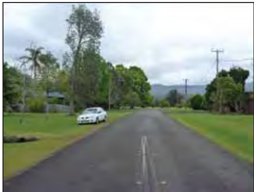
Looking north along Edward Street
