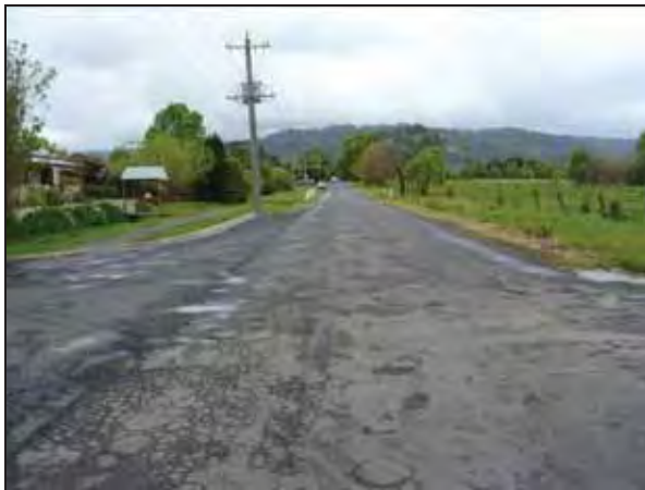
Looking west along North Street, from intersection with Albany Street
