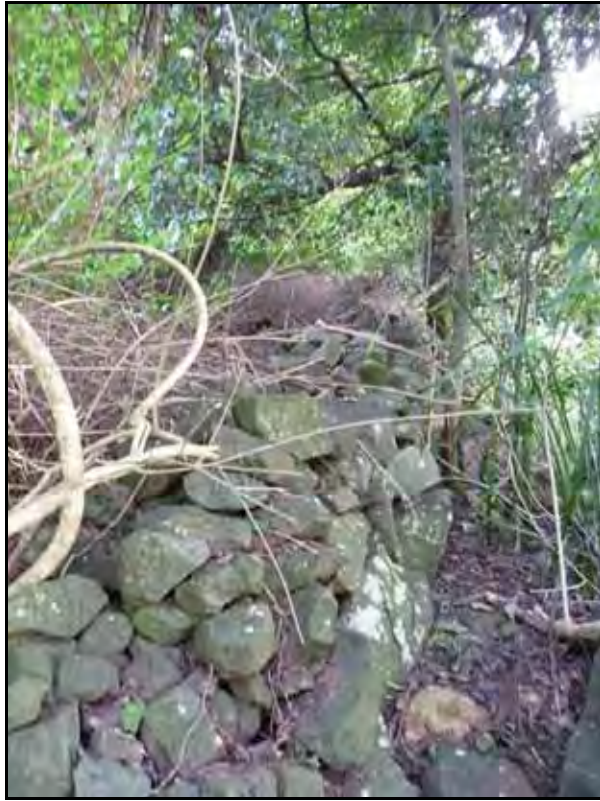
Figure G.233 Detail of dry stone wall , looking NW from near the southern known extent of the wall. Note partial collapse in foreground and large foot stones
