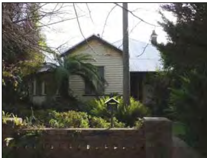
Figure G.73 Detail of front of building, looking N
