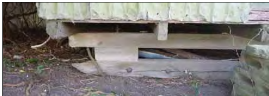
Figure G.240 Detail of wood skid mounted below floor (door side)
