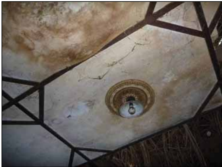
Figure G.178 Detail of ceiling and light fitting
