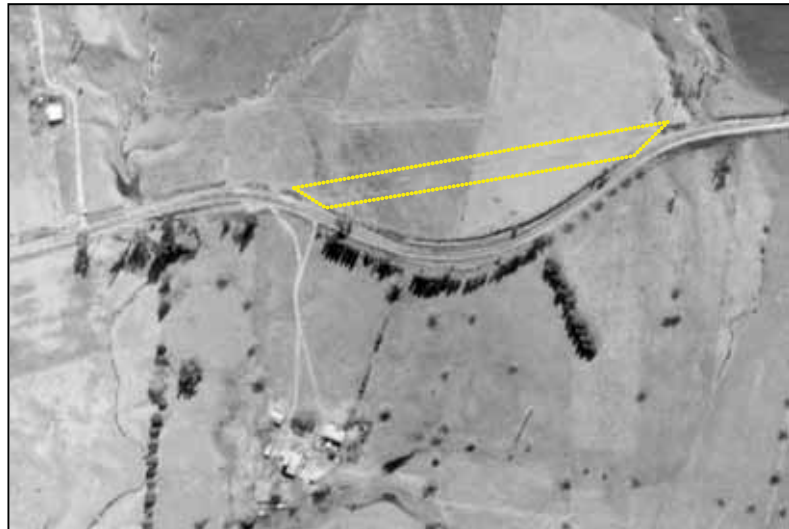
Figure G.10 Road remnant visible on 1958 aerial photo (outlined in yellow), (NSW 699-5029, SH.I Dapto-Ulladulla Run GK11 23/07/58)
