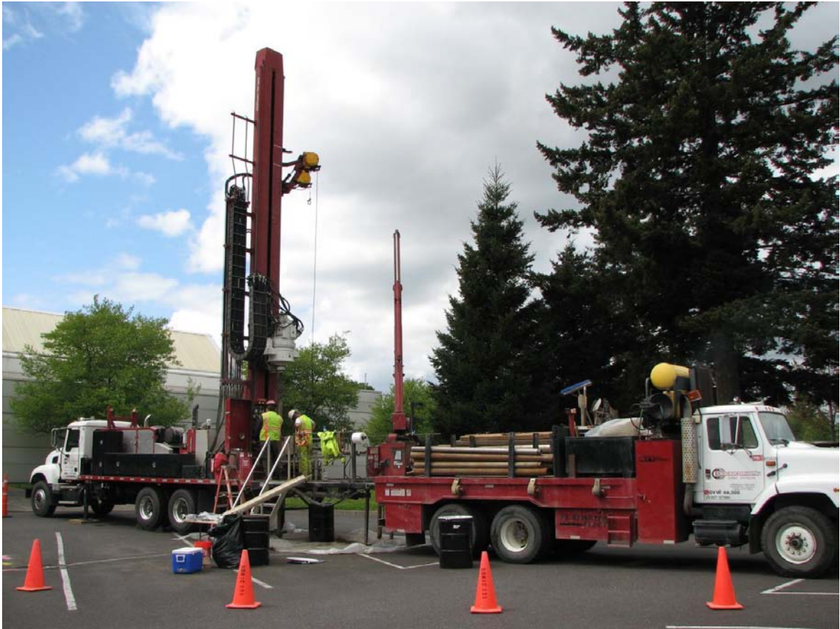
Figure 5.2 Example of process to obtain boreholes
