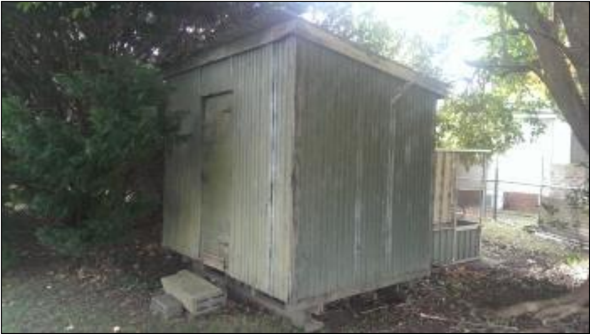
Plate 1: Southern and eastern elevation of skid mounted shed (G2B H60). Source: Biosis 2014
