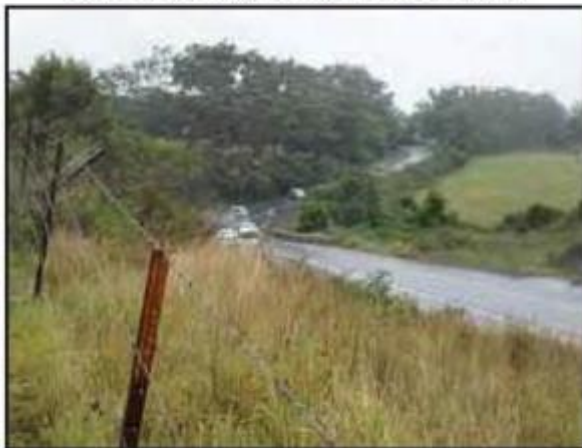
Highway alignment west of Sedgford
