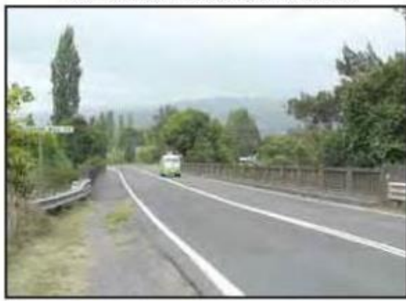
Bridge (constructed 1955) over Broughton Mill Creek, Berry
