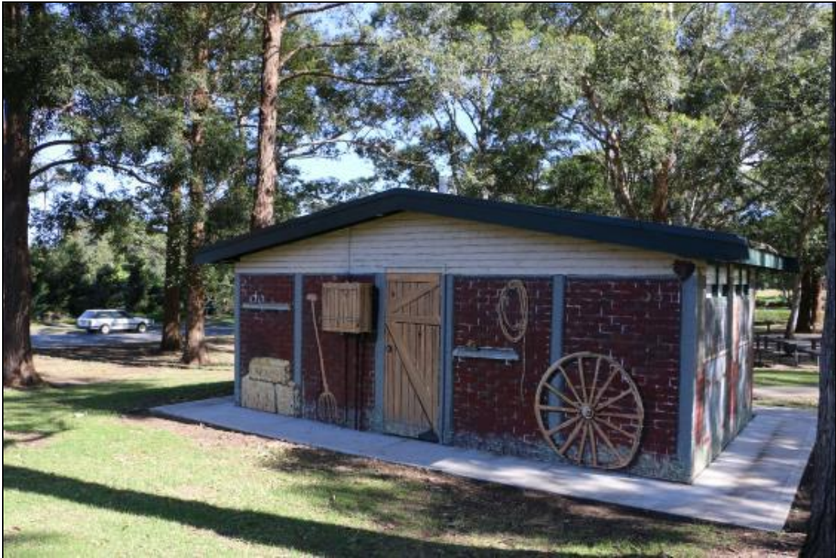
Plate 9: Mark Radium Park, detail of mural painted on toilet block, view to SW. Source: Biosis: 2014
