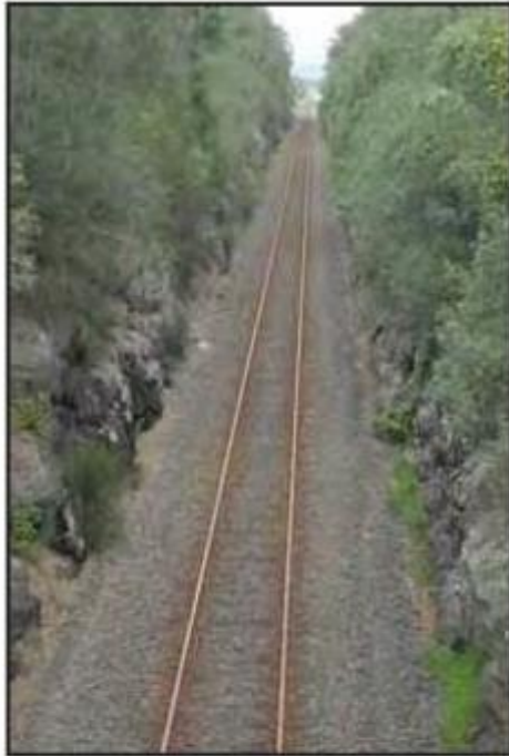
Railway cutting, Dooley Road, Toolijooa
