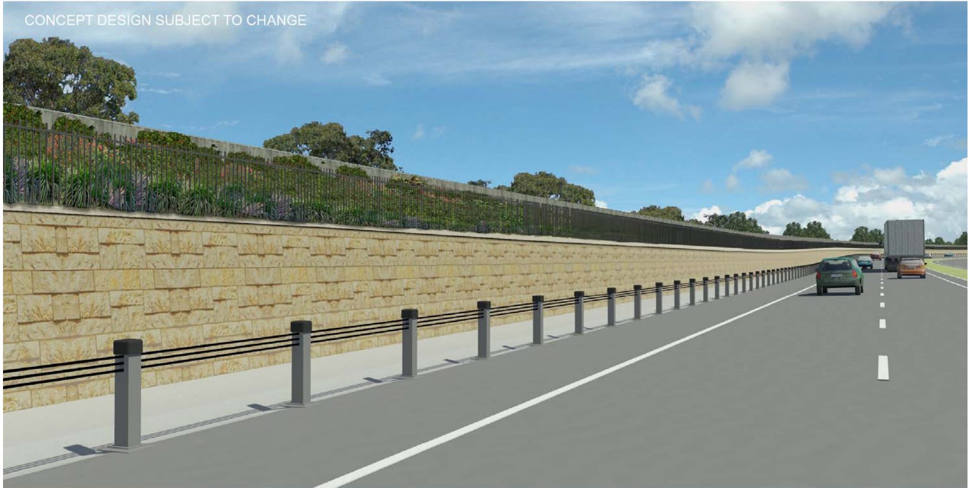
Northern Route - Noise Barrier Design
