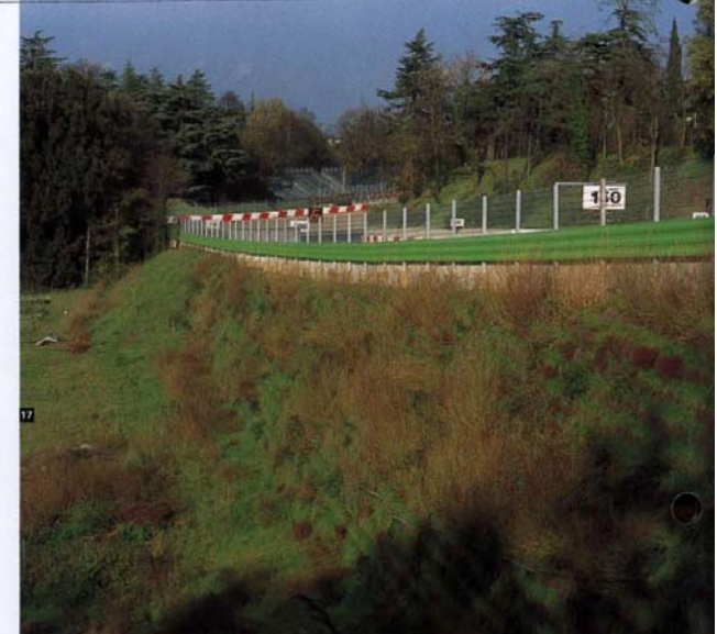
14-15-16-17. Retaining work along race track at Imola carried out by using soil type reinforced Green Terramesh ® , Imola-Italy.
