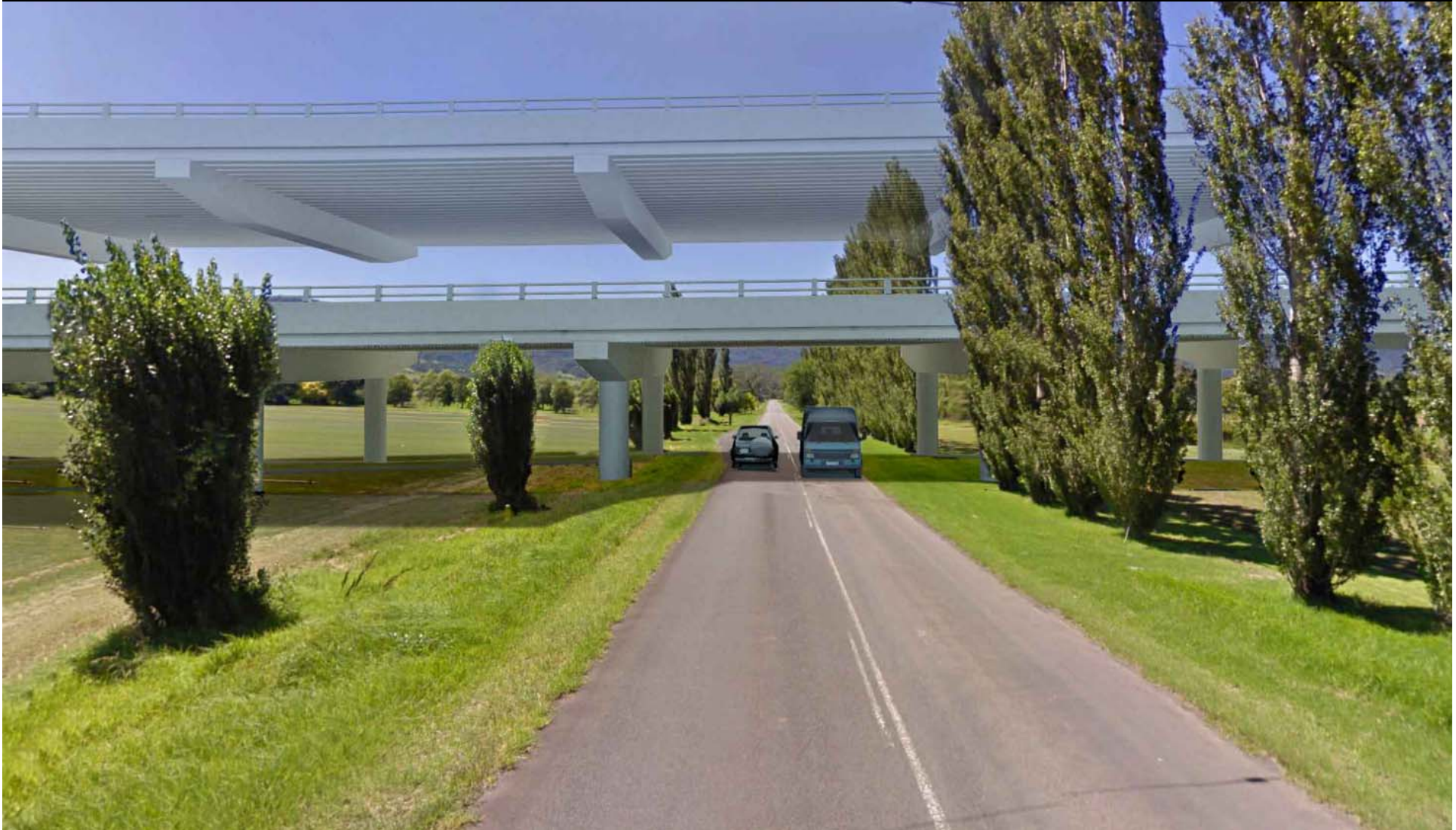
Woodhill Mountain Road crossing bridge height comparison
