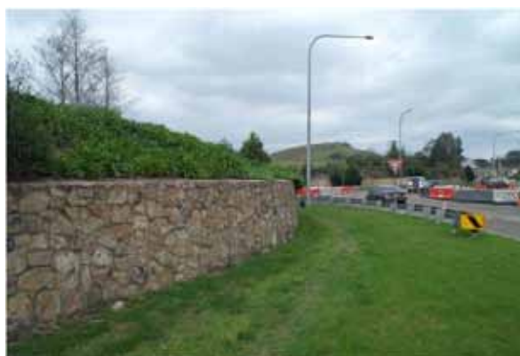
Stone faced retaining wall.
