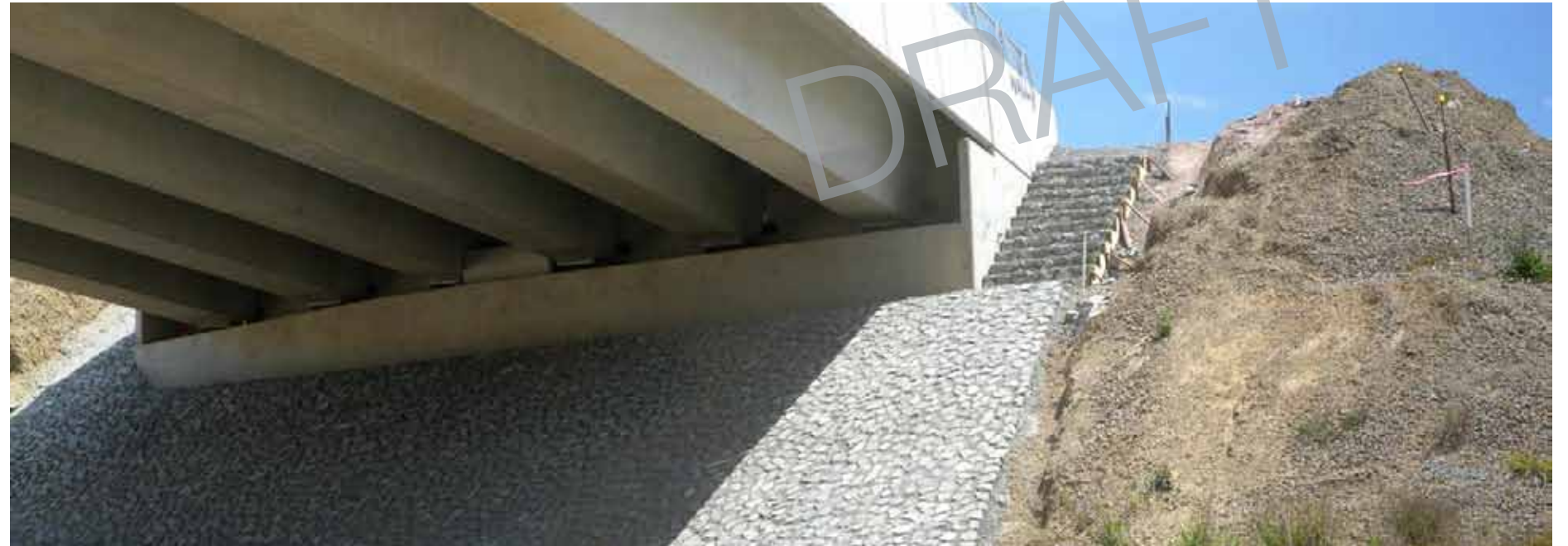
Figure 7: Stone faced abutment.
