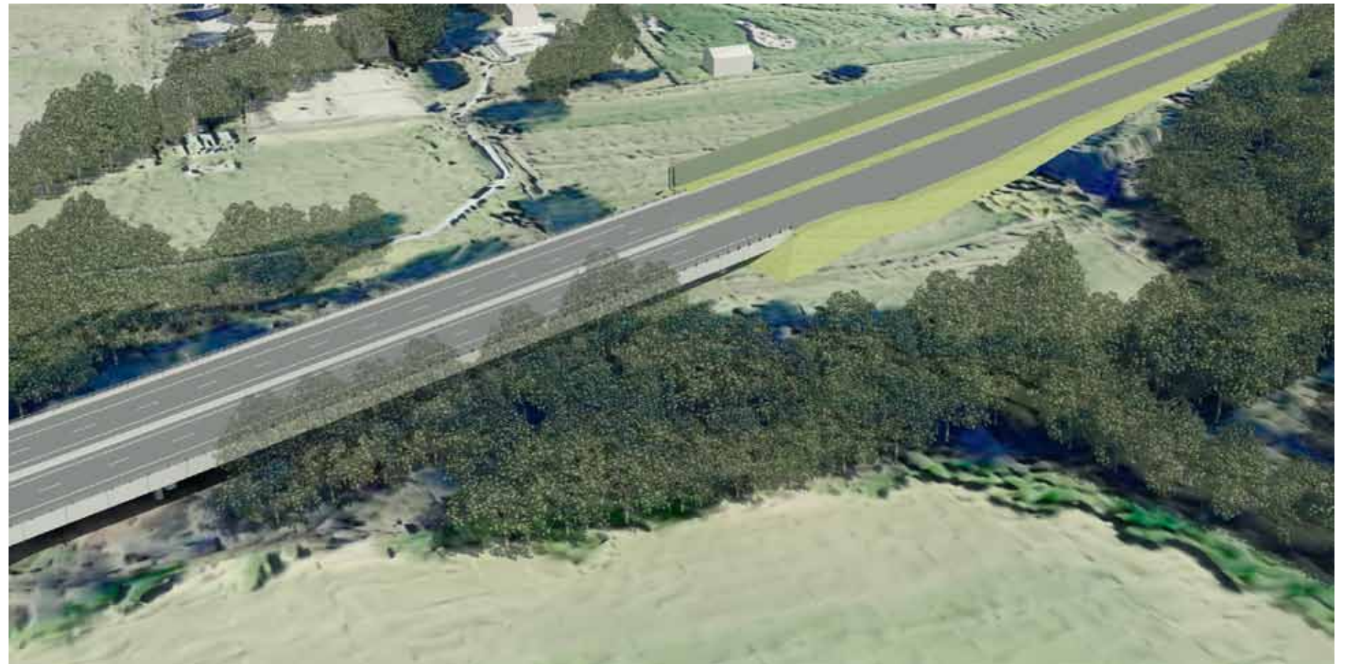
Figure 10: Aerial view of south abutment.
