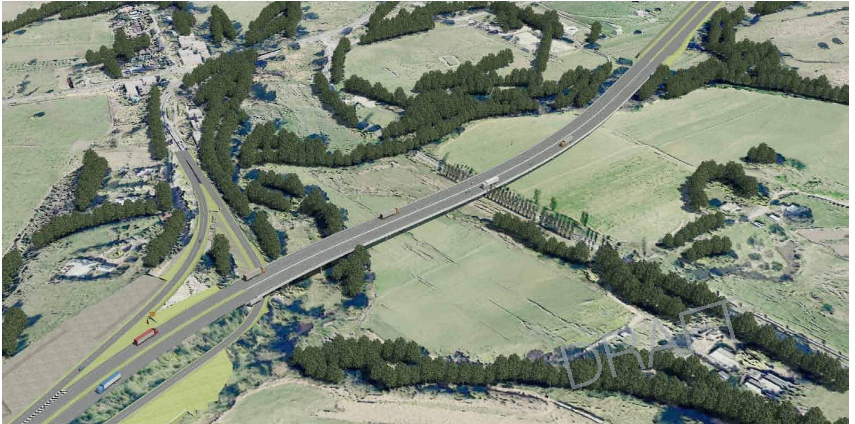
Figure 5: Berry Bridge - Aerial view from northeast.
