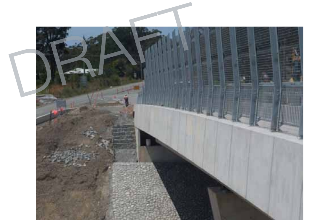
Figure 9 : Stone faced abutment - showing maintenance access stair.
