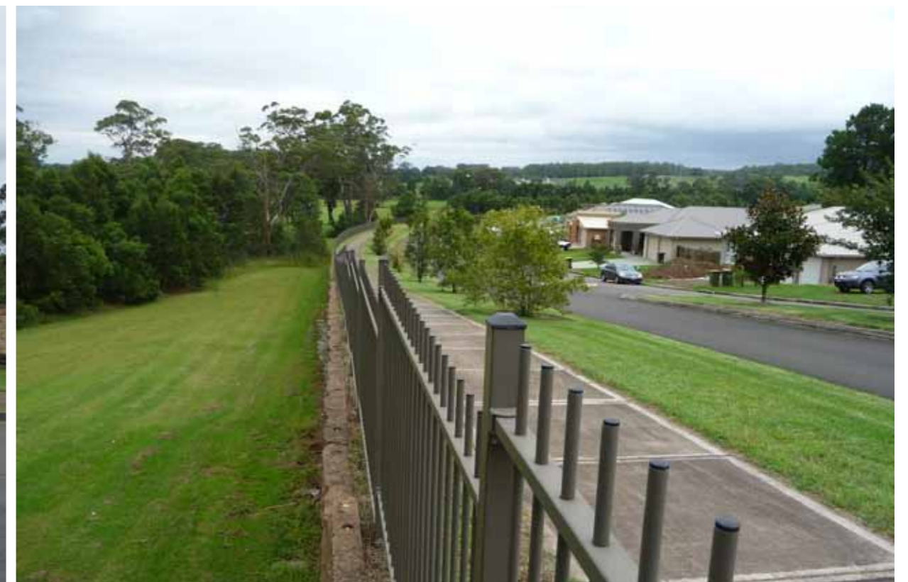
Large retaining wall supports east side of Huntingdale Park Road.
