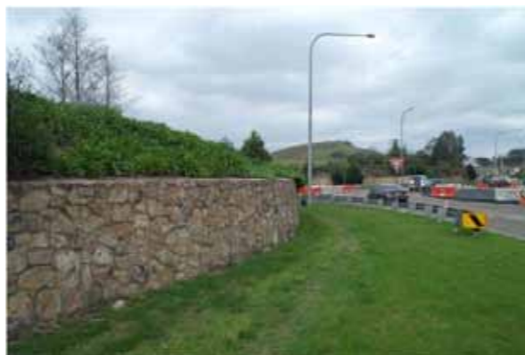
Stone faced retaining wall.
