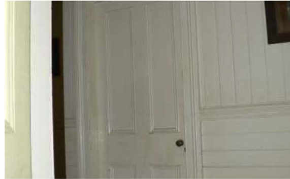
P1230603 Typical corridor wall & doorway
