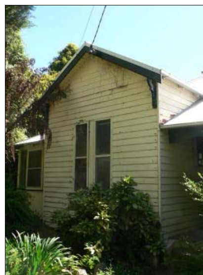
Figure 9: Kitchen Gable and canopy
