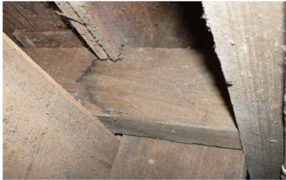
P1230566 Stud continuing past floor boards
