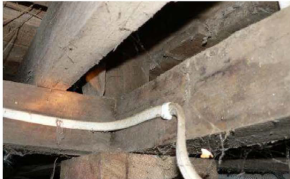
P1230568 Floor framing
