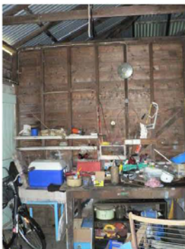
P1230642 Wall around laundry from garage
