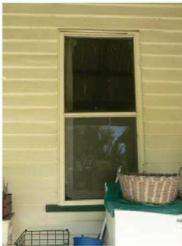
P1230590 North window - lounge
