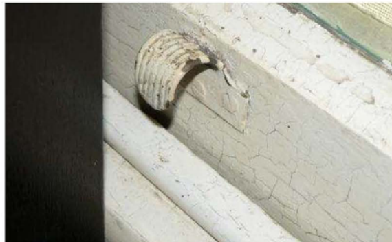
P1230619 Typical sash lift
