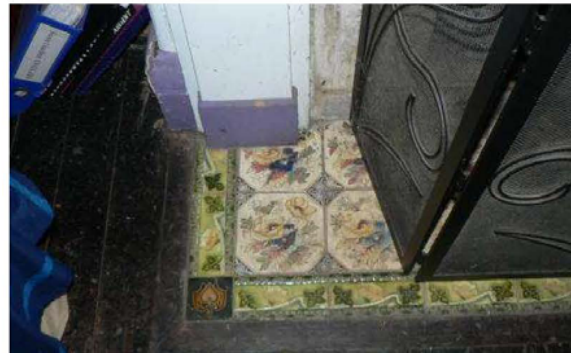
P1230607 Hearth tiles Bedroom 2
