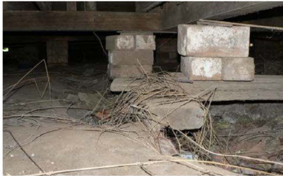
P1230563 Floor framing under rear entry door
