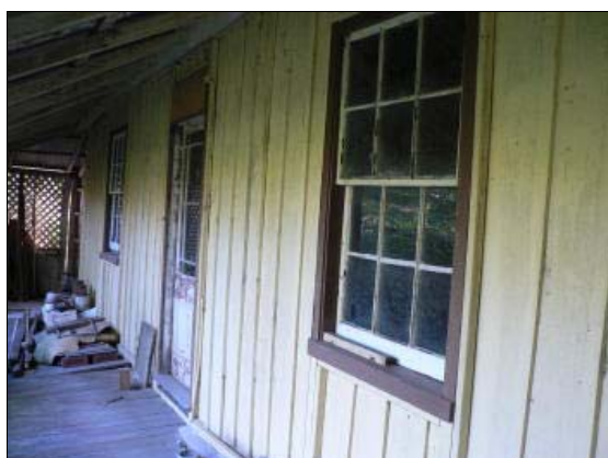
Figure 34: Front verandah view
