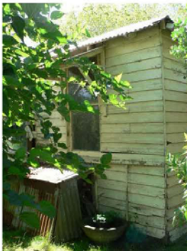
P1230638 Part west wall garage
