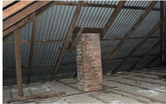
P1230553 Roof framing east chimney
