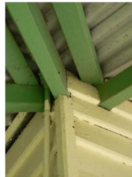
P1230594 Detail at verandah roof & wall junction
