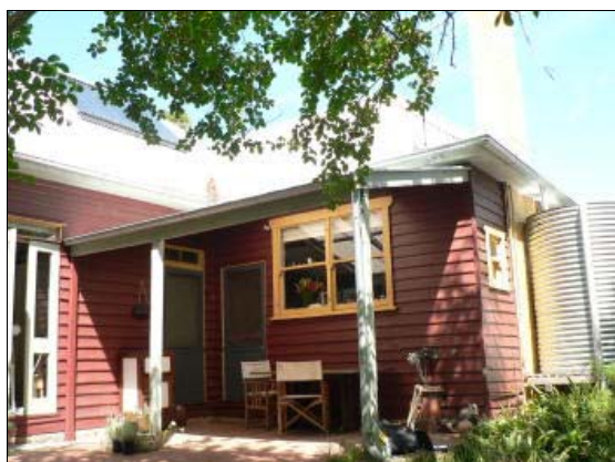
Figure 26: External view of Kitchen
