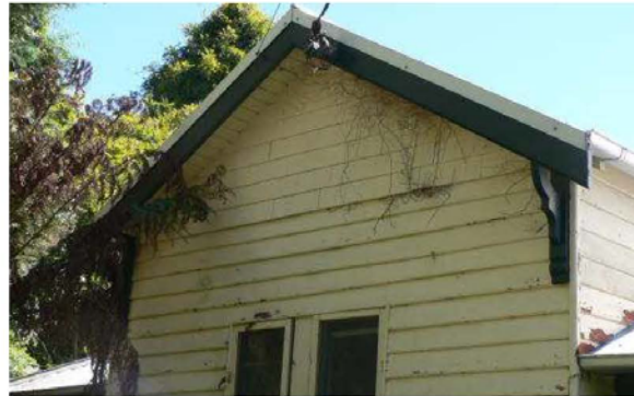
P1230575 Shingle cladding to gable
