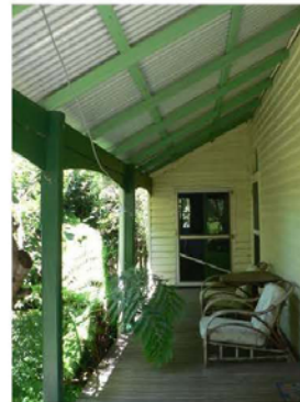
P1230597 View of eastern verandah
