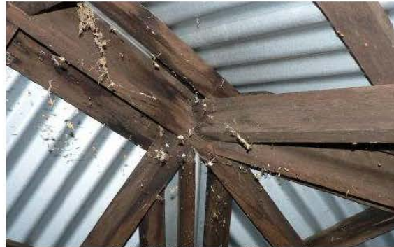
P1230556 Ridge framing detail
