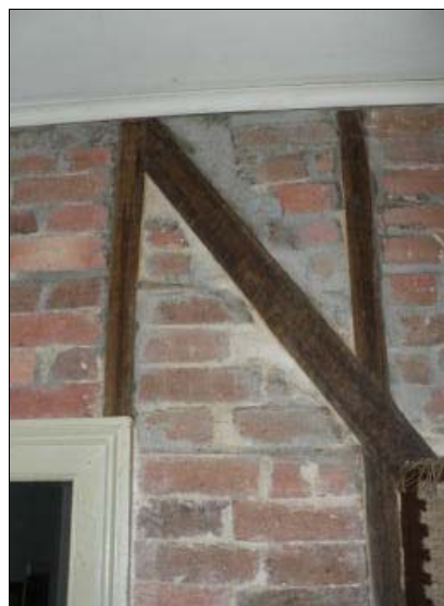
Figure 25: Brick Nog detail
