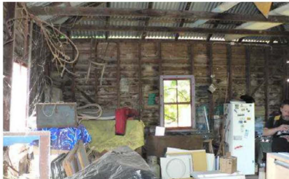
P1230645 West wall of Garage
