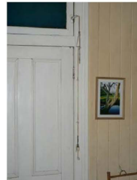
P1230610 Highlight window opening mechanism
