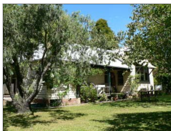
Figure 5: Cottage from North East
