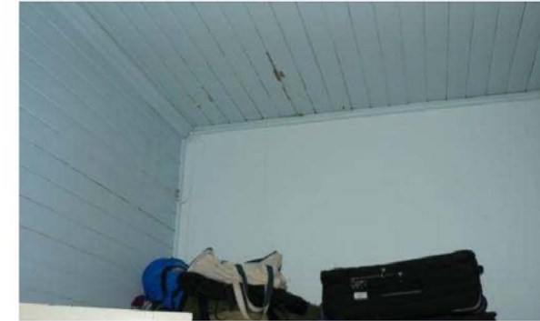
P1230604 South wall & ceiling Detail Bedroom 3
