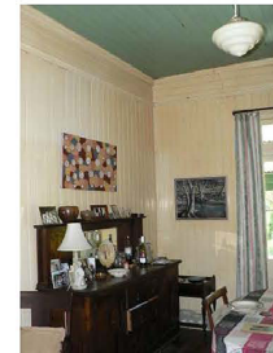
P1230608 Wall & ceiling detail dining room
