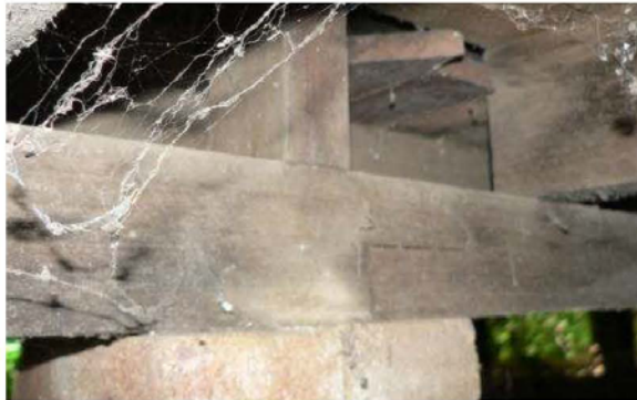
P1230569 Floor framing detail
