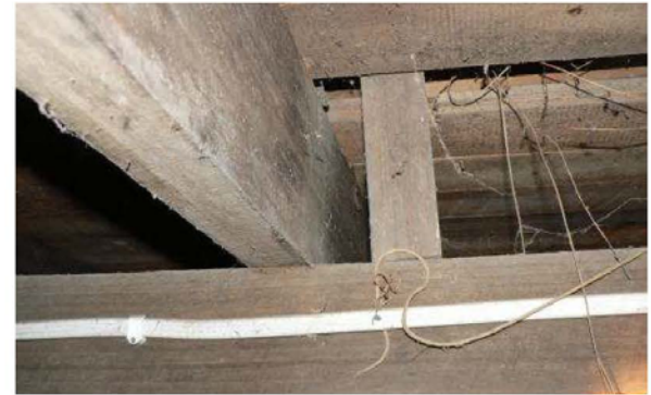
P1230567 Wall stud continuing to bearer
