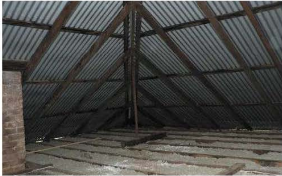
P1230552 Roof framing south east corner
