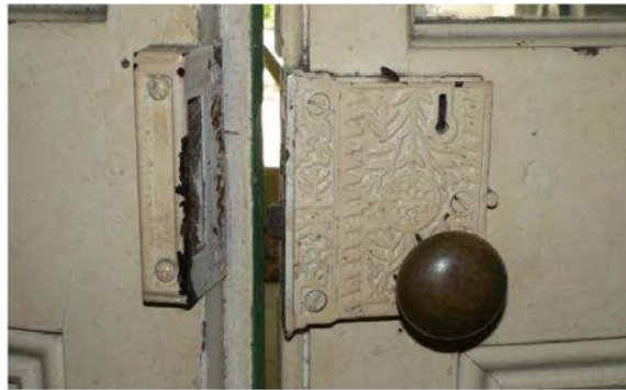
P1230612 Typical lock to verandah doors
