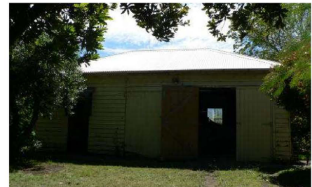
P1230633 South wall of garage
