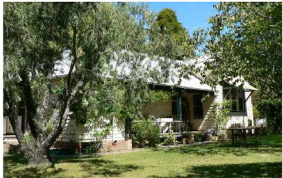
P1230588 Bathroom & kitchen section of north elevation
