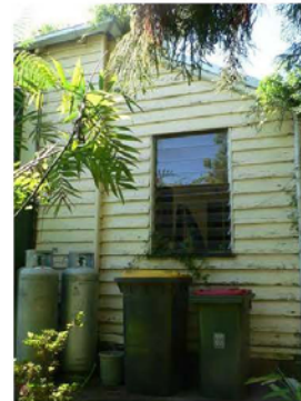
P1230578 Kitchen extension west wall
