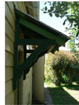
P1230637 Detail of canopy over laundry door
