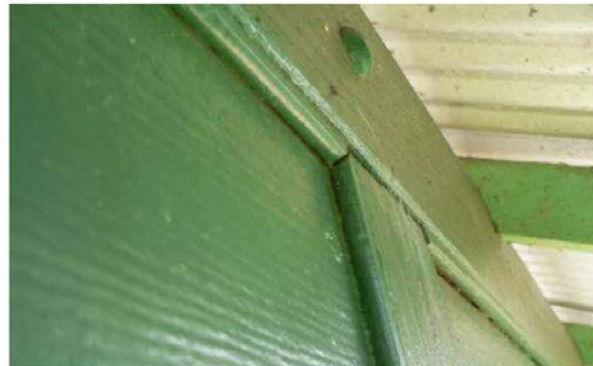
P1230593 verandah wall cladding
