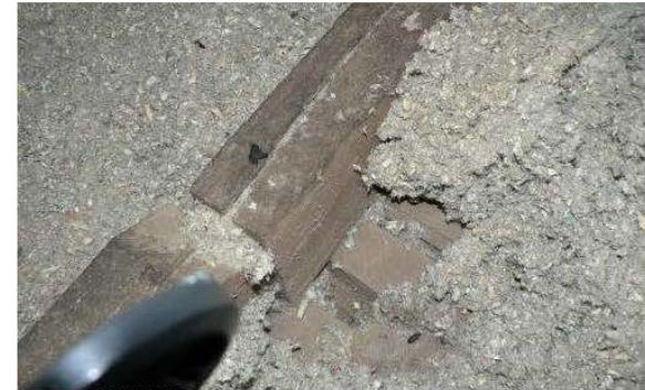
P1230557 Mortice & tenon joint in top plate
