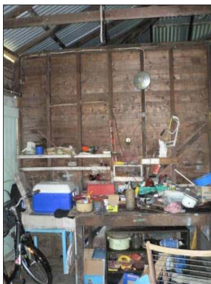
Figure 20: Wall around Laundry
