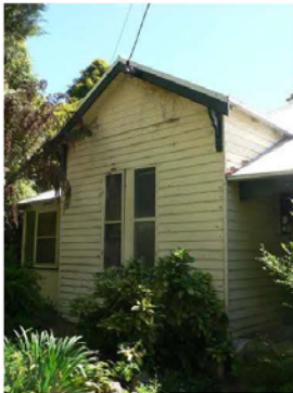
P1230574 Front wall gable projection
