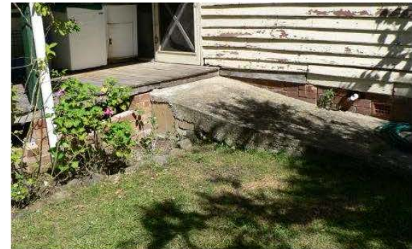
P1230561 Rear bathroom & ramp addition
