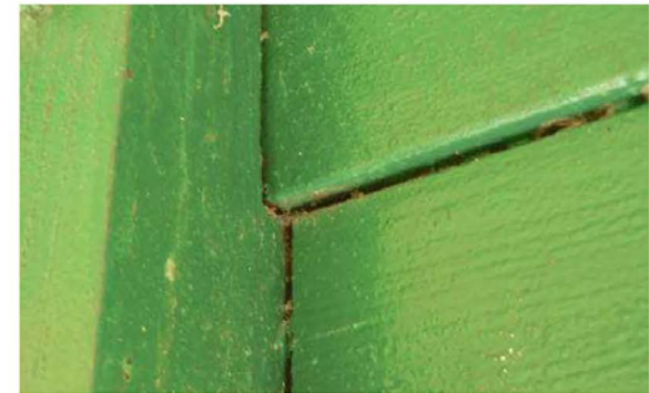
P1230592 verandah wall cladding
