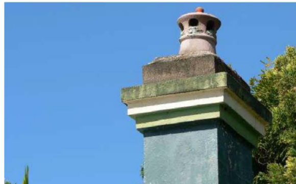
P1230582 Top of kitchen chimney
