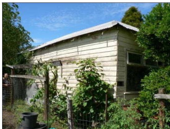
Figure 11: Shed from North West
