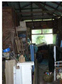
P1230643 View to area behind laundry
