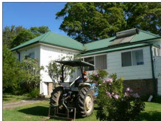
Figure 29: Cottage from rear showing added wing on right
