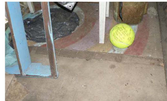
P1230644 Evidence of former wall line back area of garage
