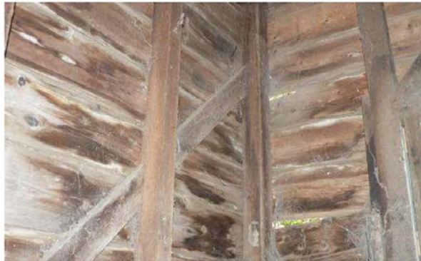
P1230649 Wall bracing details
