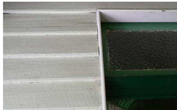
P1230632 Typical wall to door frame detail
