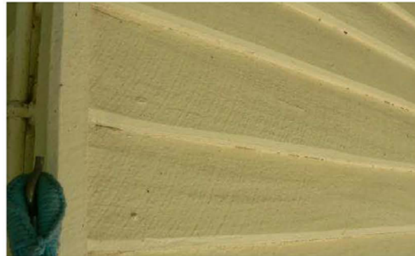
P1230596 Representative weatherboards showing profile & saw marks
