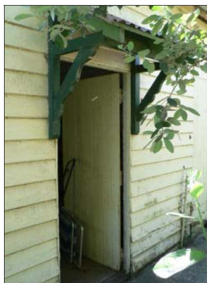
Figure 13: Laundry door and canopy
