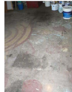
P1230651 Location of filled in service pit
