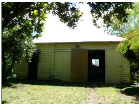
Figure 10: Shed from driveway
