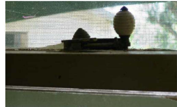
P1230618 Typical sash lock
