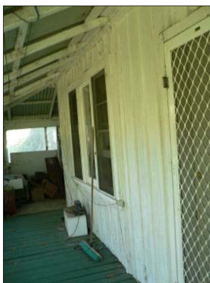
Figure 30: Front verandah construction
