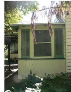
P1230576 South wall of west verandah
