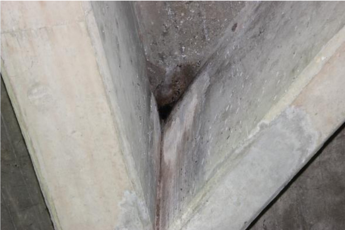
Photo 2 Southern Myotis roost location Broughton Mill Creek Bridge
