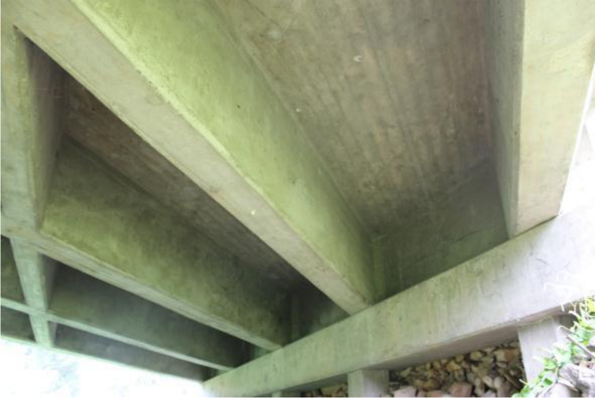
Photo 1 Broughton Mill Creek Bridge with Southern Myotis
