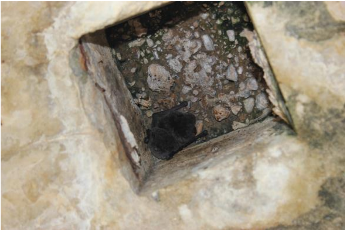
Photo 4 Southern Myotis roost location in Flying Fox Creek culvert
