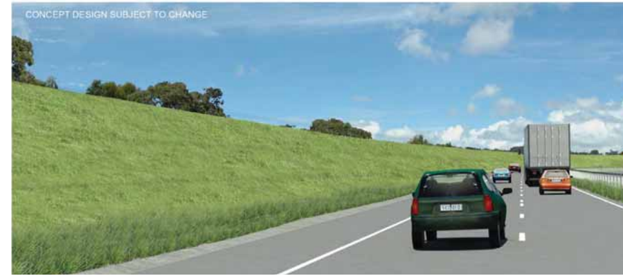
Fig. 6.16: North Street noise barrier EA Concept Design option 2 – planted soil reinforced mound
