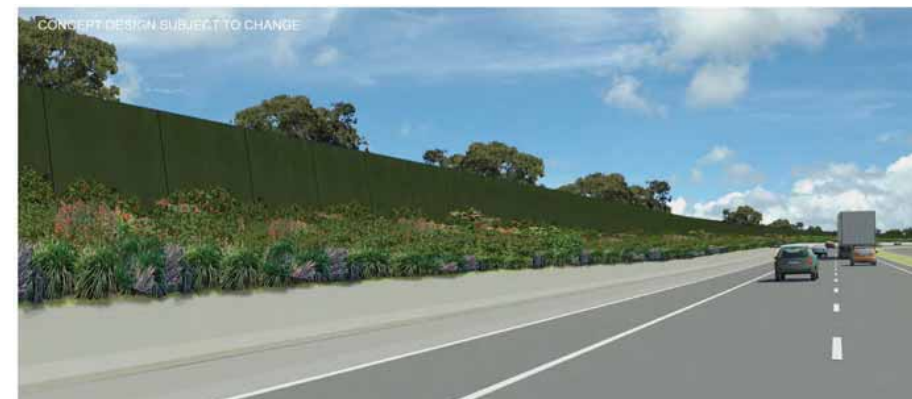
Fig. 6.15: North Street noise barrier EA Concept Design option 1 – precast concrete wall (Source: EA Appendix I, Roads and Maritime Services, 2012)
