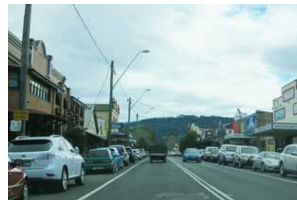
Fig. 2.9: Retail and commercial areas of Berry along Queen Street
