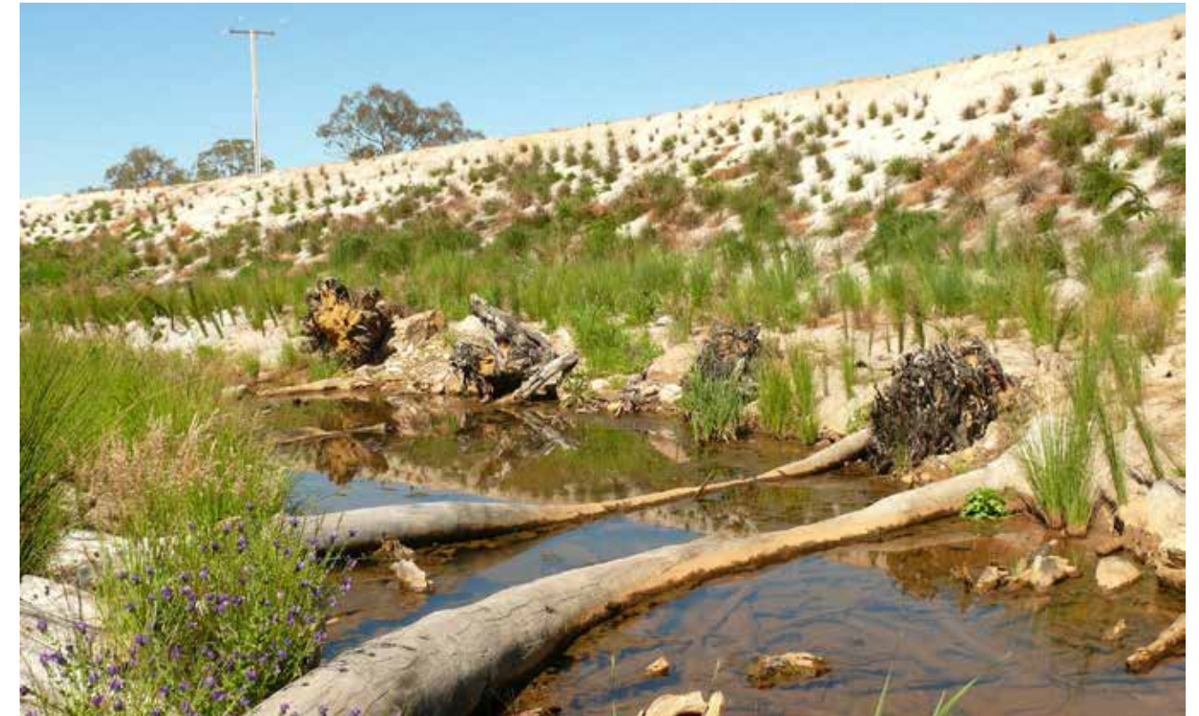
Fig. 6.34: Naturalistic treatment to creek realignment
