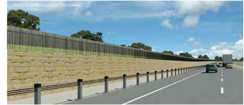
Fig. 6.17: North Street noise barrier EA Concept Design option 3 – combined stone wall and timber fence
