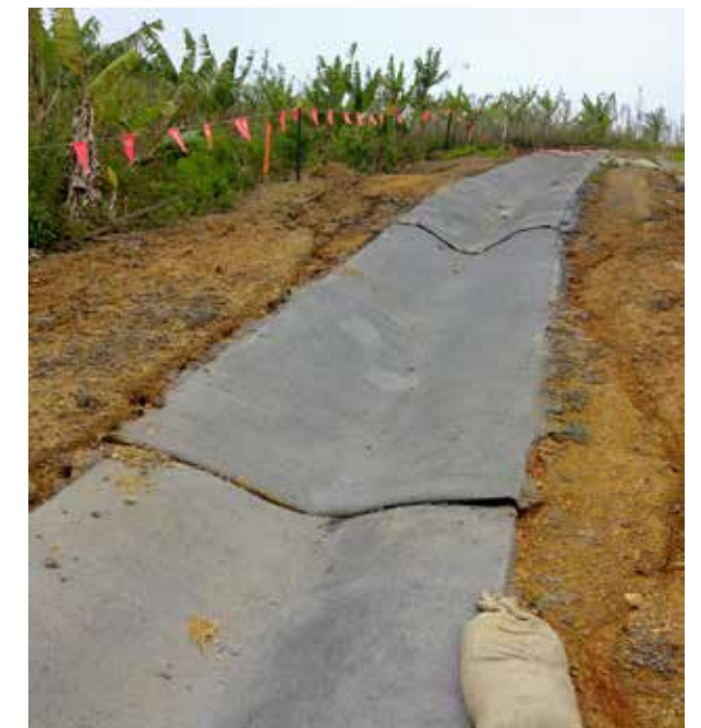
Fig. 6.35: Example of a concrete lined channel
