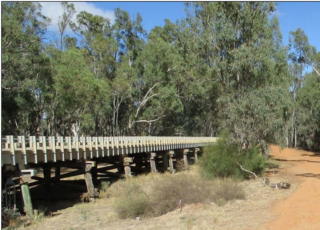
Figure 2.2: Gee Gee flood relief bridge
