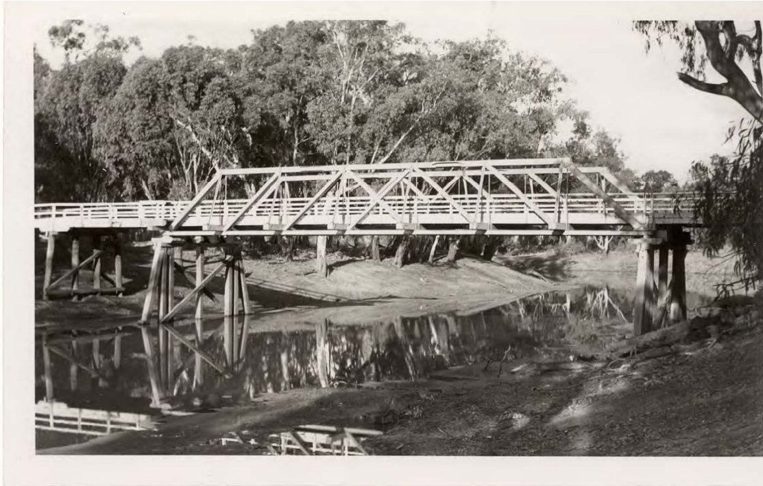
Figure 5: Gee Gee bridge, 1940s. (Source: Transport for NSW).
