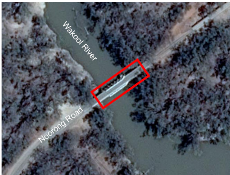
Figure 1: The Gee Gee Bridge over the Wakool River, on Noorong Road, Cunninyeuk. (Base image: Google Earth).
