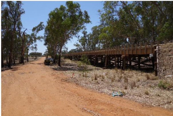
Image 13 – Access track and fill at south west abutment
