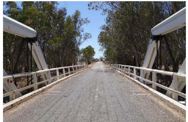
Image 2 - Main channel bridge, towards Wakool
