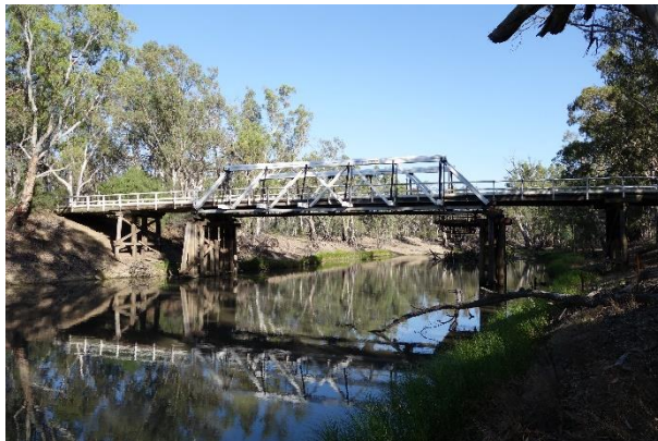
Image 1 - Main channel bridge from the east
