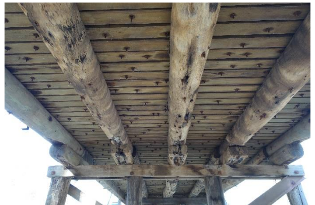
Image 8 - Underside of bridge from north east bank
