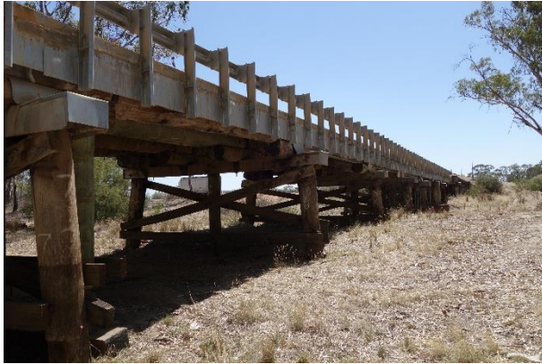
Image 11 - Flood recovery bridge from south
