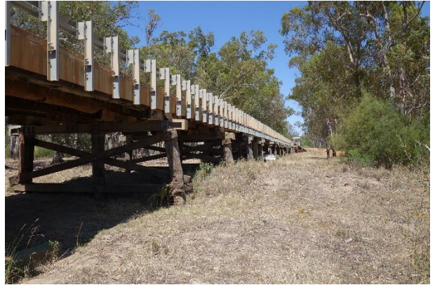
Image 12 – Flood recovery bridge from north
