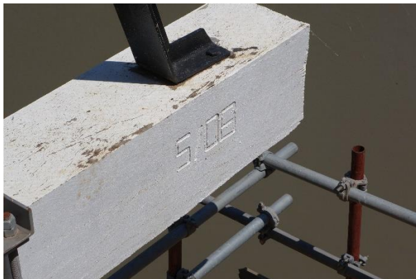
Image 9 - Truss span repair works dated May 2008
