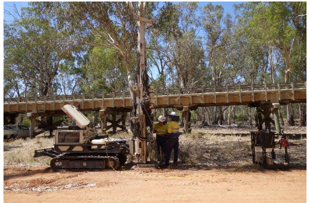
Image 14 – CPT rig to north of bridge
