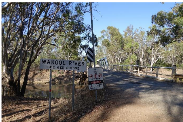
Image 3 - Main channel bridge, north east abutment
