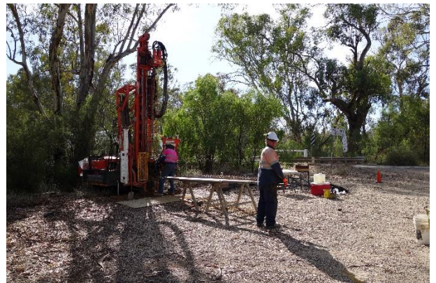
Image 10 - Drilling at proposed south west abutment
