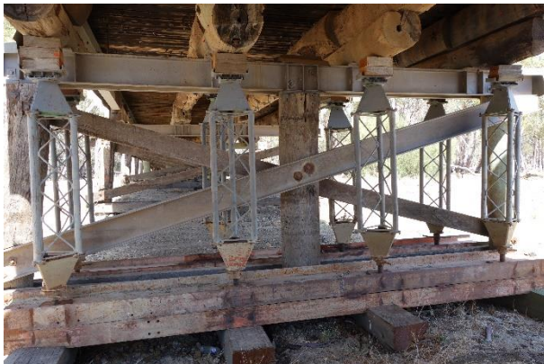
Image 15 – Steel truss props
