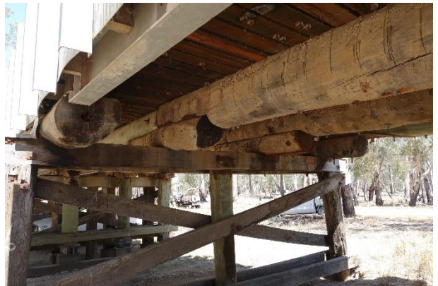
Image 16 – Steel beam replacing timber log
