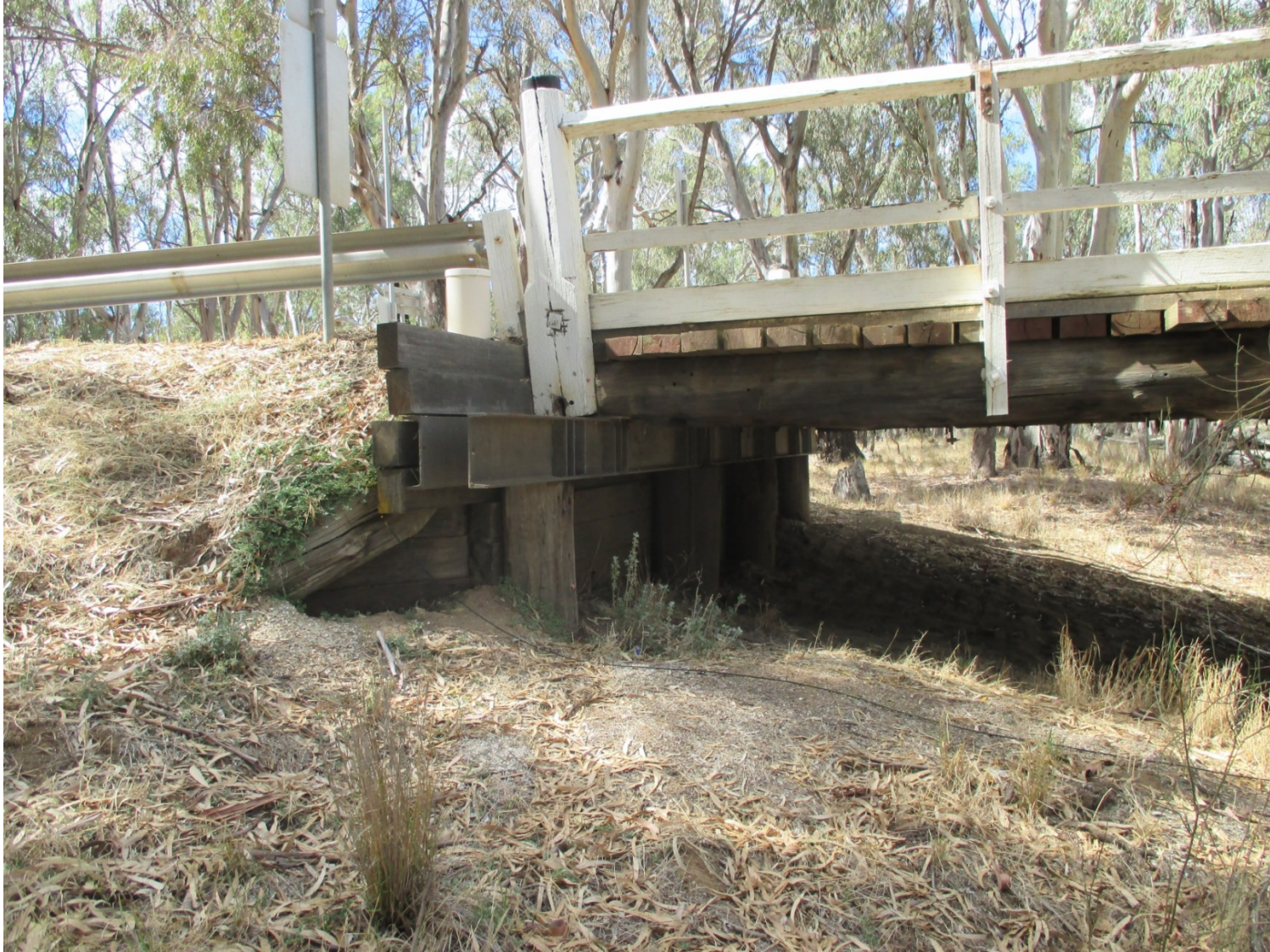
Plate 8 – Main Bridge Abutment A
