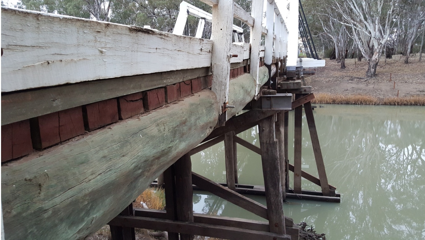
Plate 13 – Replaced timber on Main Bridge
