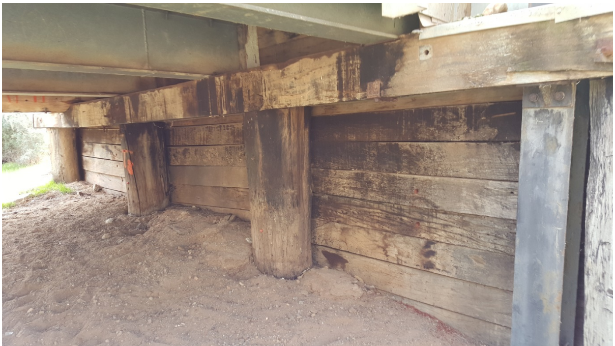
Plate 14 – Approach Bridge Abutment A
