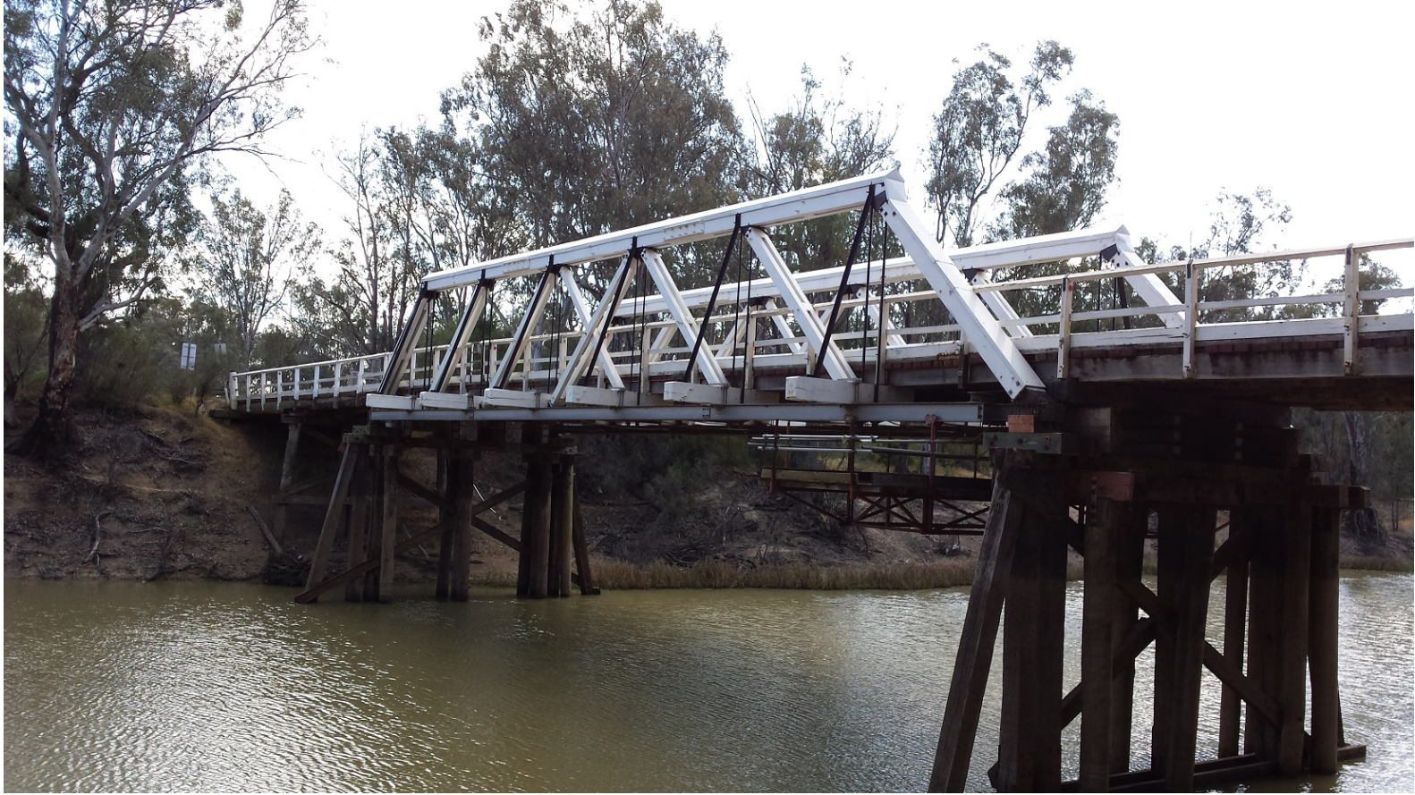
Plate 21 – Main Bridge from south western bank
