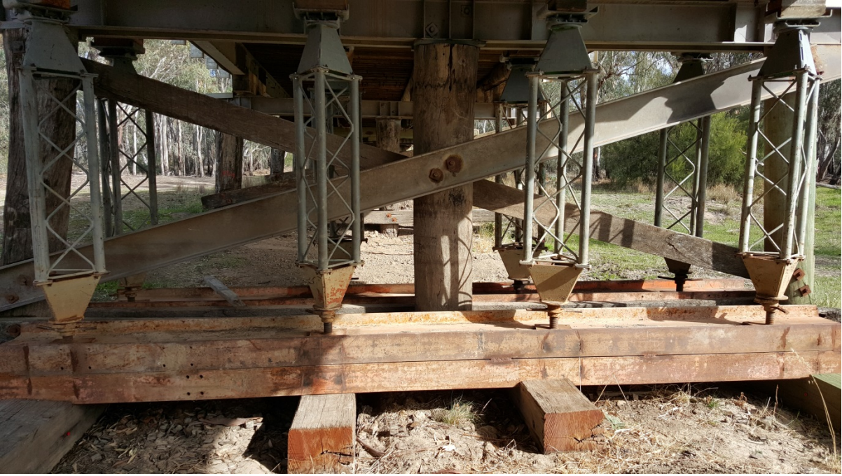
Plate 3 – Temporary replacement steel TOMs
