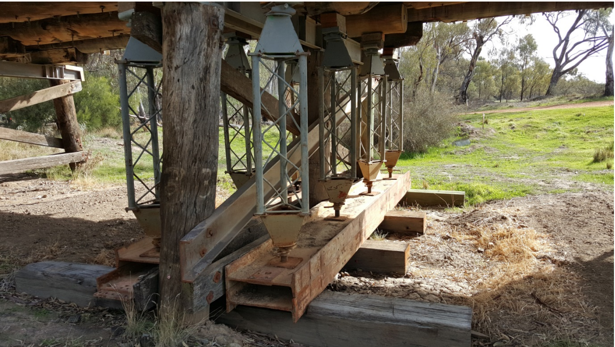
Plate 2 – Temporary replacement steel TOMs
