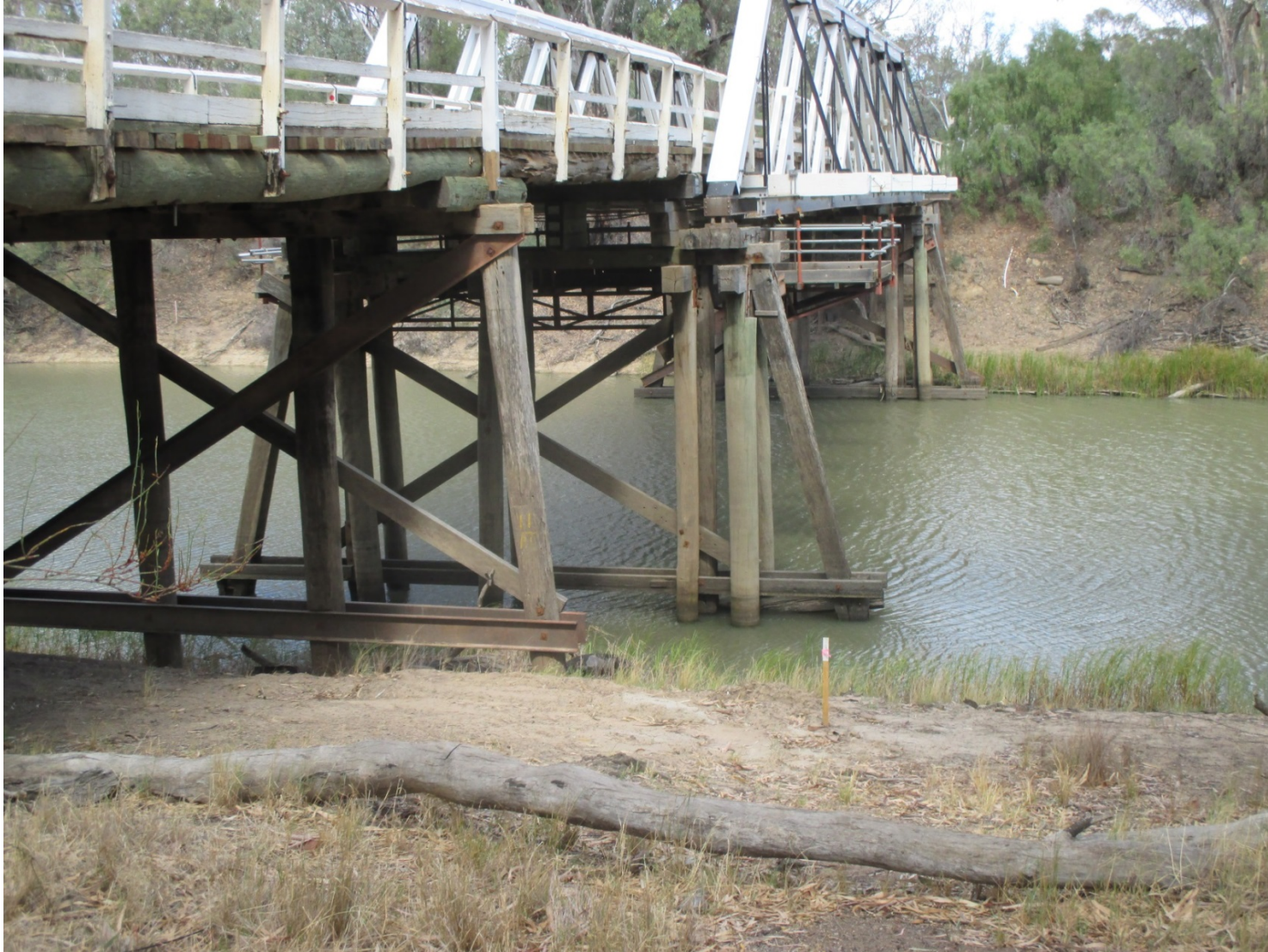
Plate 7 – Main Bridge from the north west bank
