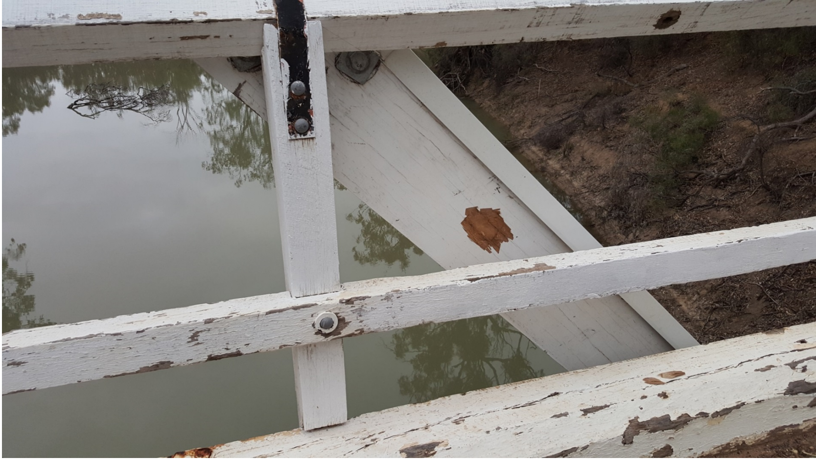
Plate 9 – Truss bridge sample First diagonal
