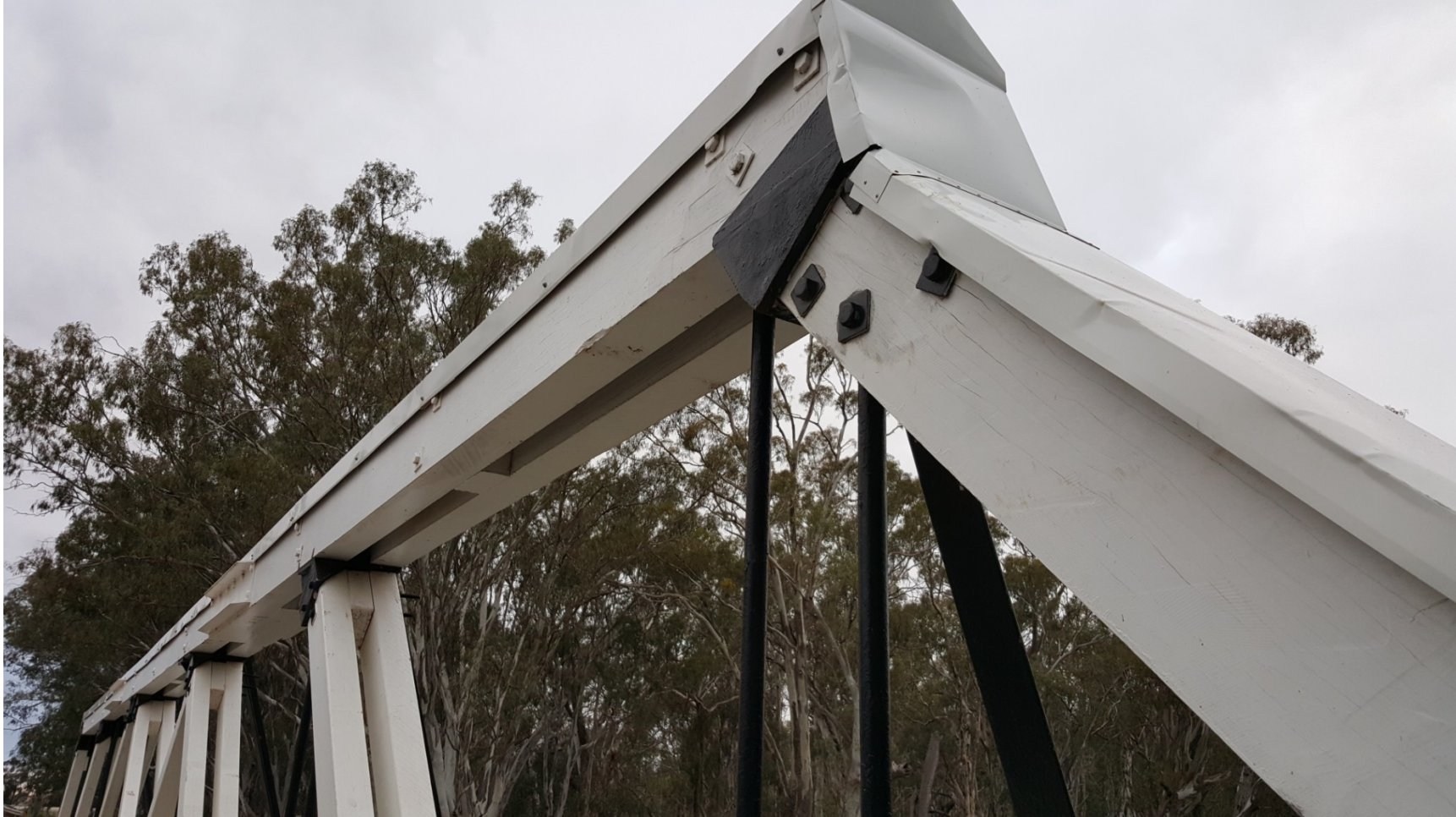
Plate 10 – Truss Top Chord
