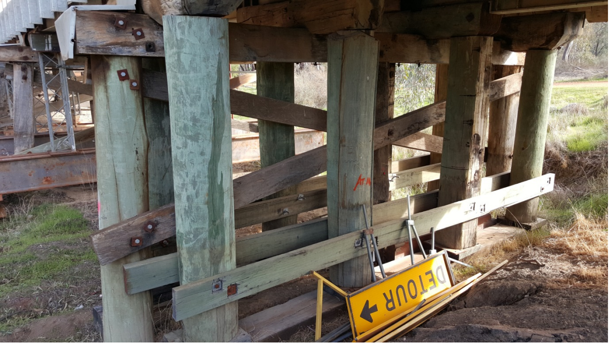
Plate 1 – Piers with replaced treated timber
