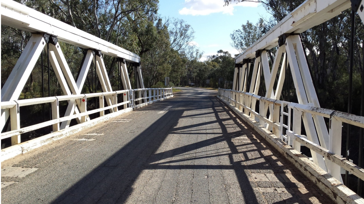
Plate 20 – Main Bridge looking south
