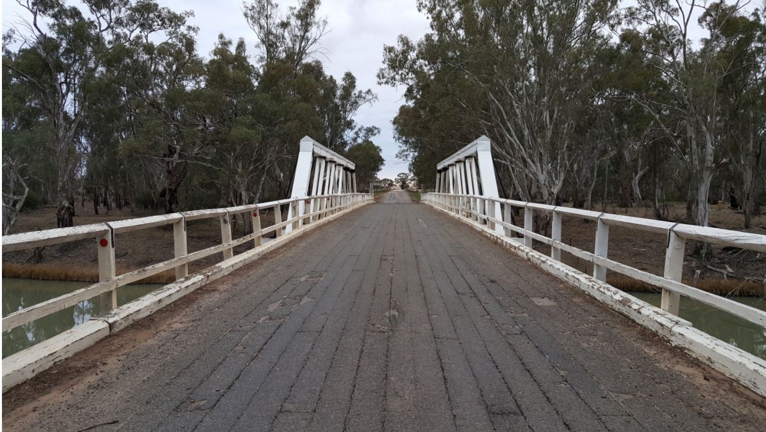
Plate 12 – Main Bridge Decking
