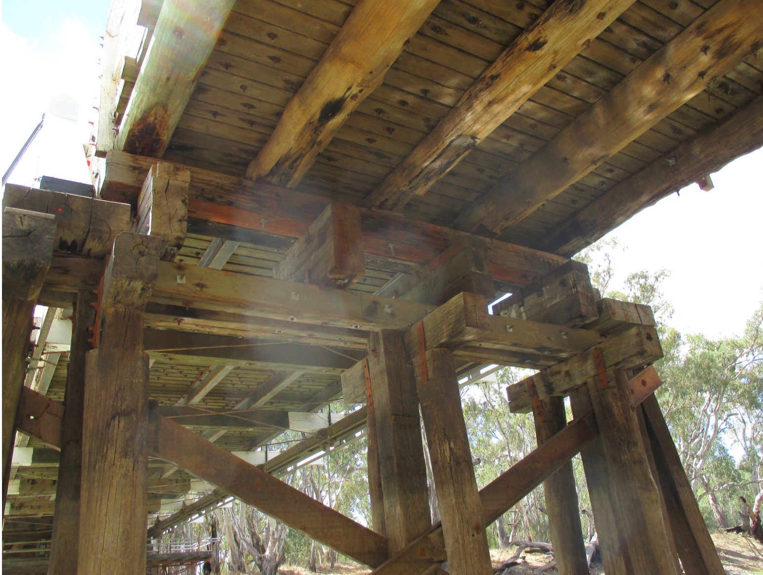
Plate 2 – Main Bridge including piers, piles and bracing
