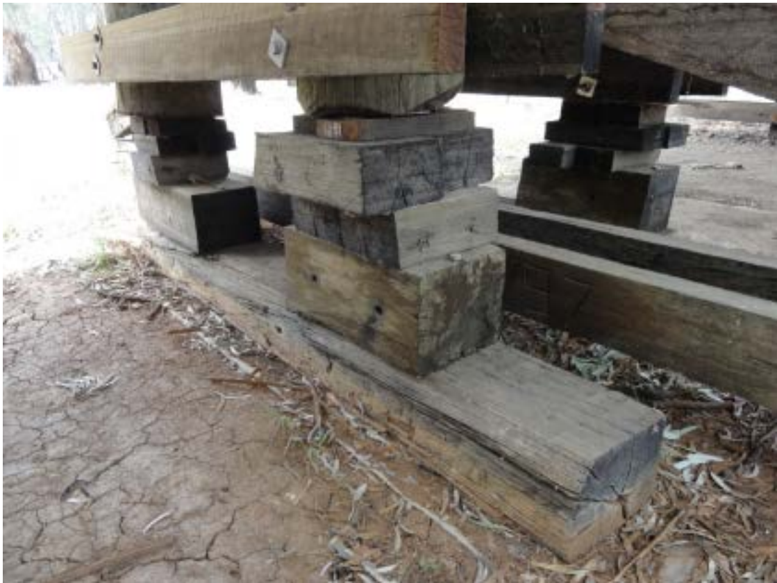
Plate 16 – Example of additional timber retro-fitted to Piers
