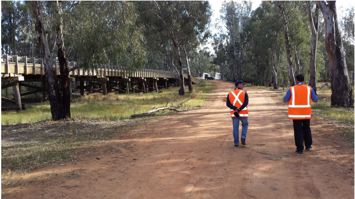
Plate 13 – Approach Bridge access track
