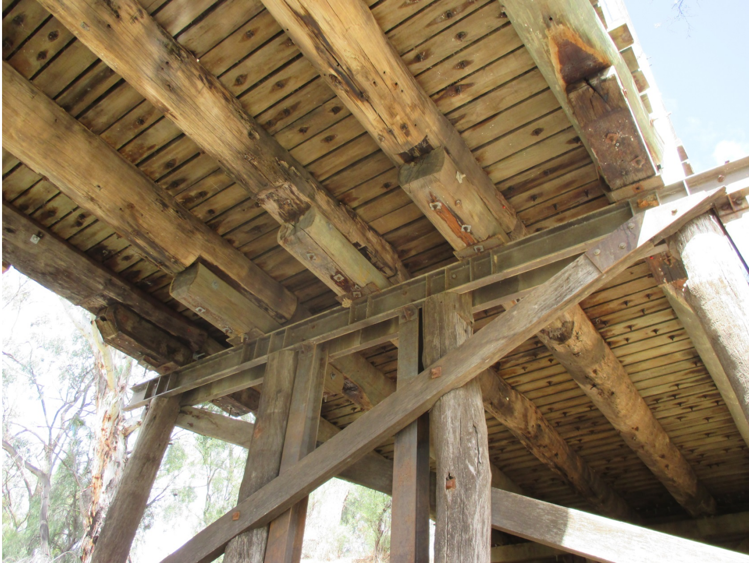
Plate 1 – Main Bridge from the ground
