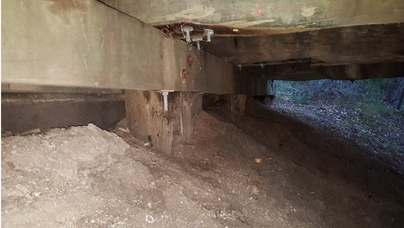
Plate 15 – Main Bridge Abutment B, fully replaced with treated timber
