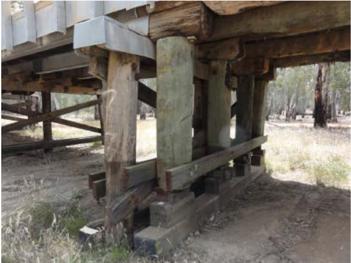
Plate 15 – Example of additional timber retro-fitted to Piers
