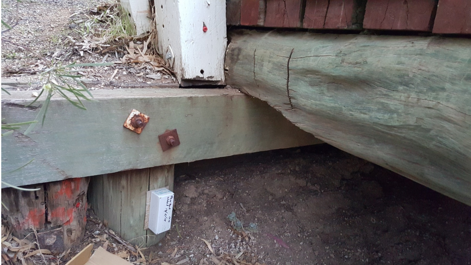
Plate 14 – Main Bridge Abutment B, fully replaced with treated timber
