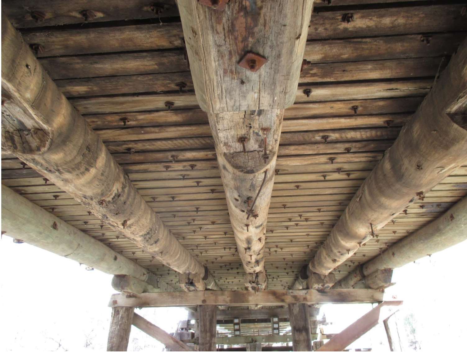
Plate 6 – Bridge cross girders
