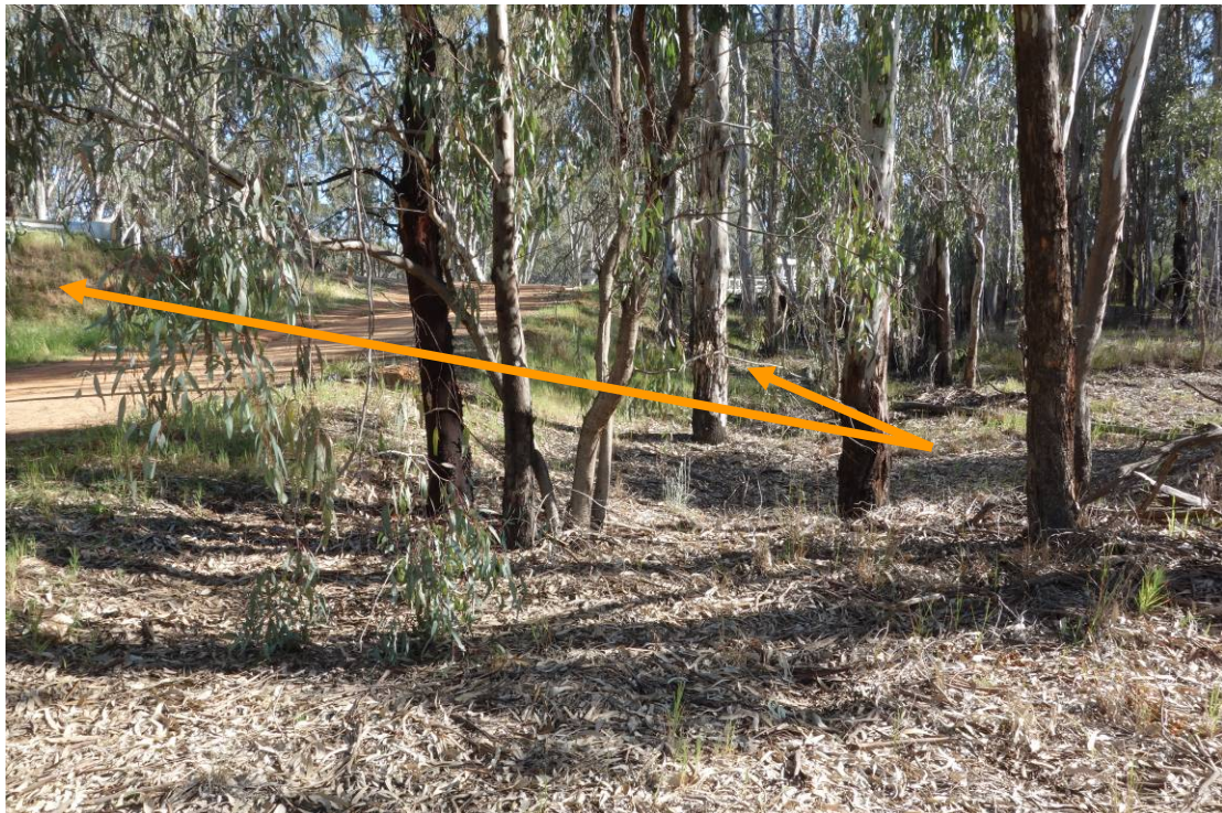
View Downstream Road Embankment between the two bridges – Remove road embankment and access track to match existing natural level
