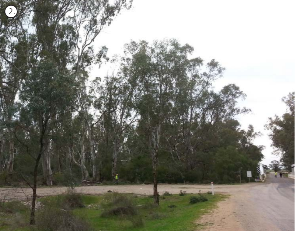
View 2 : South-western approach to the bridge
