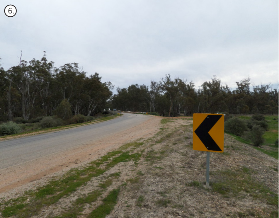
View 6 : View at curve of road to start of bridge
