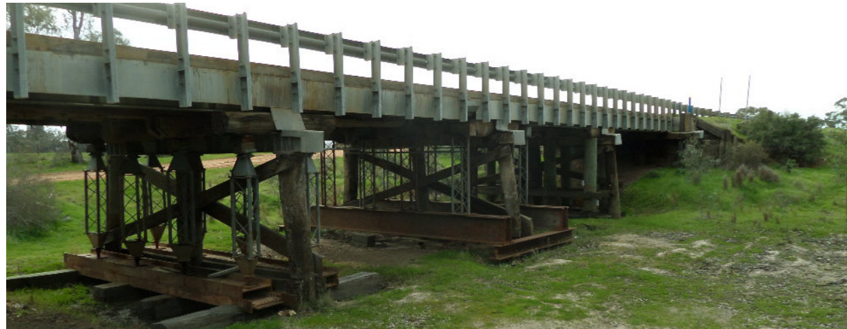
Figure 15 The northern-eastern bridge approach Source: GAO, 2015
