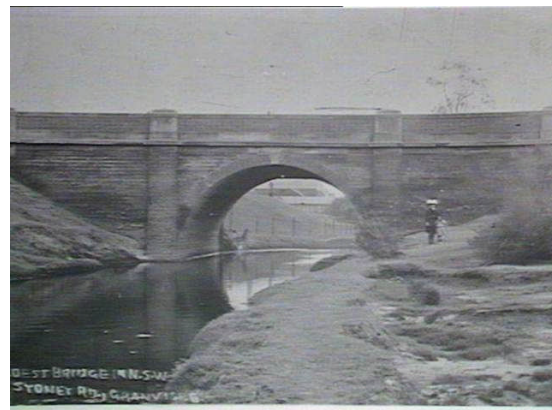
Early photograph of Duck Creek Bridge, 1838
