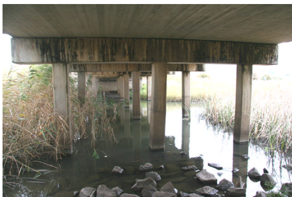
Furracabad Bridge showing flat slab reinforced concrete superstructure
