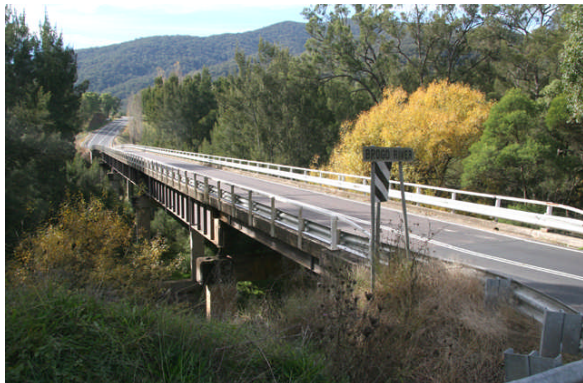
Steel girders of Brogo River Bridge.
