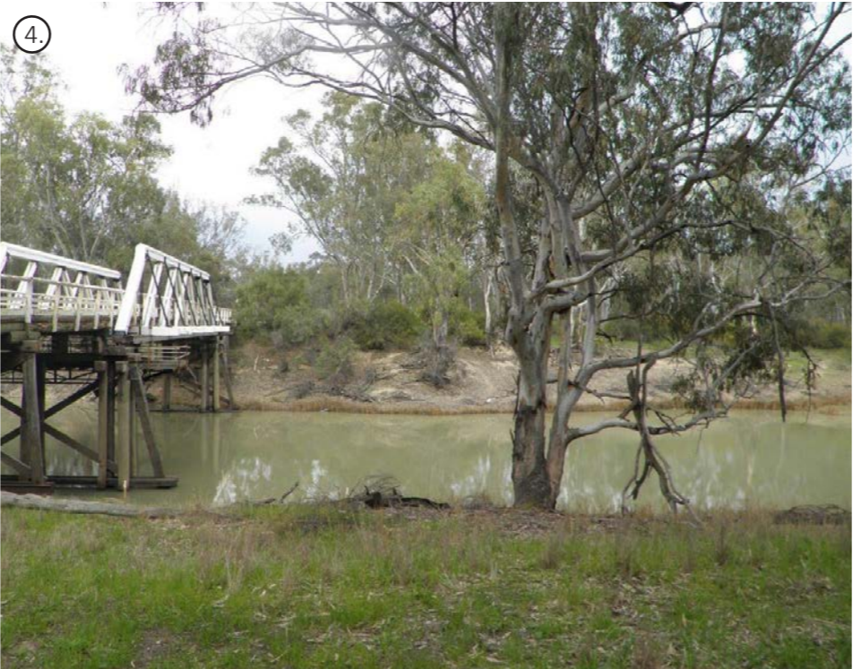
View 4 : View from top of northern side of river bank
