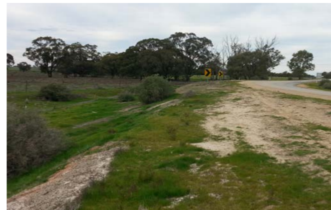
Figure 8 Banking along the eastern bridge approach Source: GAO, 2015
