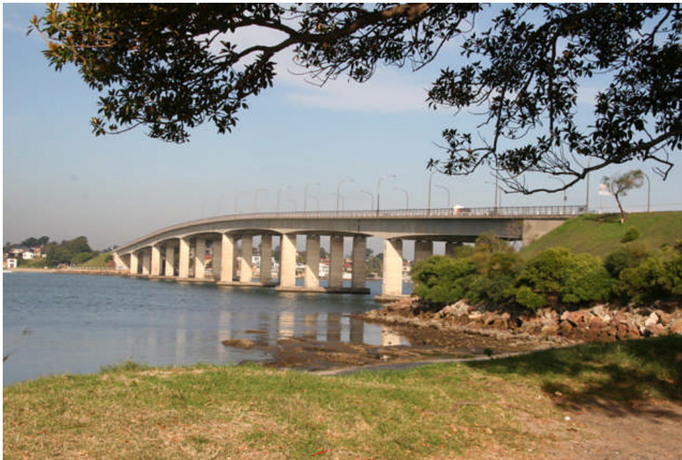
Captain Cook Bridge [RTA Bridge No 118] 1965
