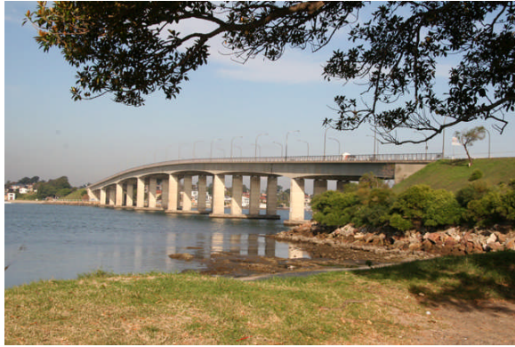
Captain Cook Bridge with elegant elliptically curved box girder soffits and slender piers
