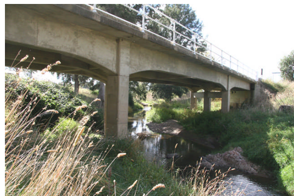
Winburndale Rivulet Bridge displaying aesthetics of curved camber and strong skew
