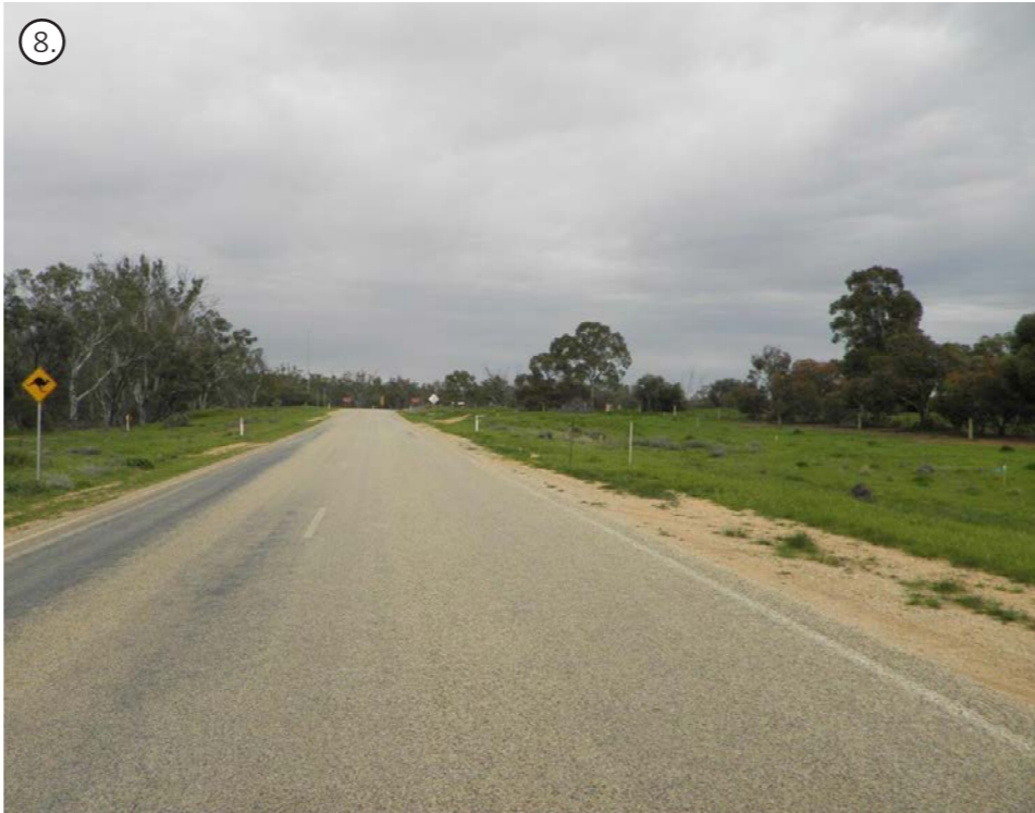
View 8 : View from the start of the new bridge approach road
