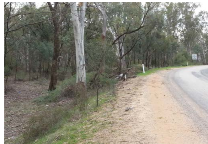
Figure 9 Banking along the western bridge approach Source: GAO, 2015
