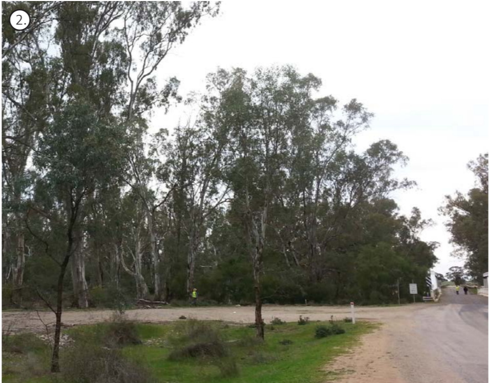
View 2 : South-western approach to the bridge
