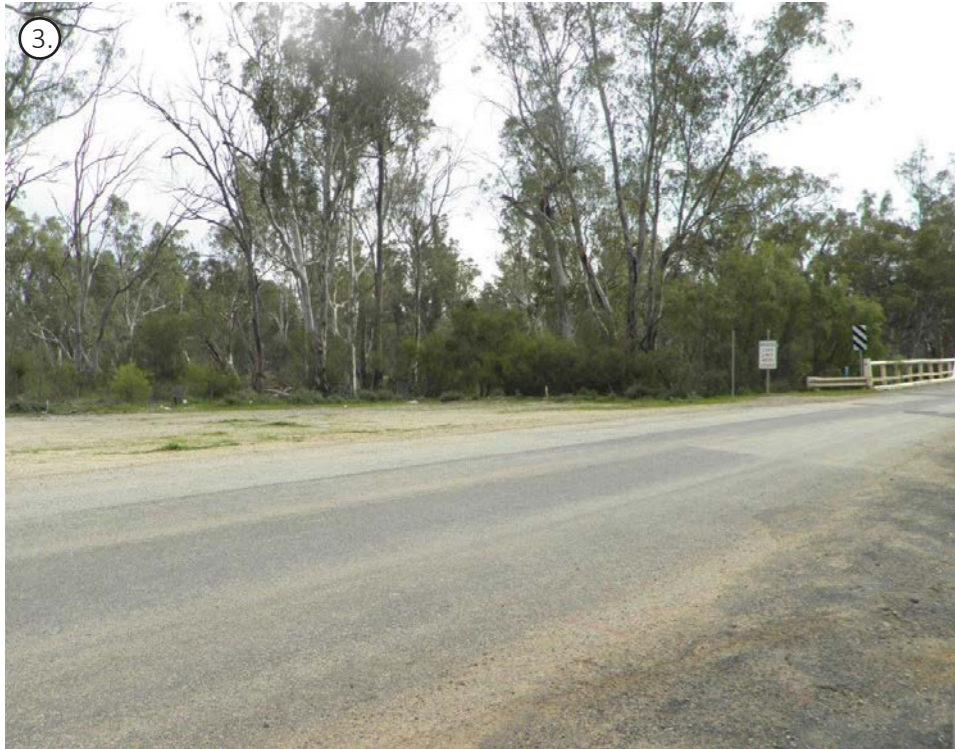
View 3 : View from top of southern side of river bank
