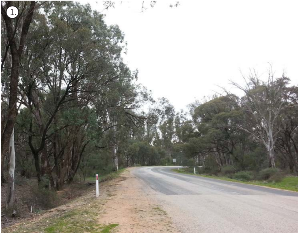
View 1 : Start of new road leading to south-western approach to the bridge
