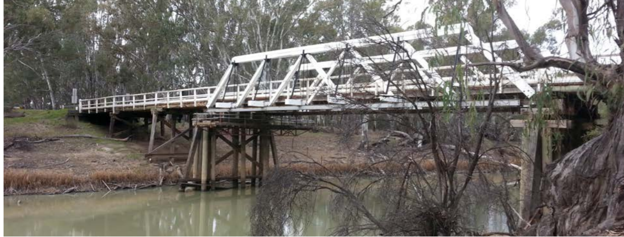
Figure 14 The Bridge - single Dare Truss and southern approach span Source: GAO, 2015
