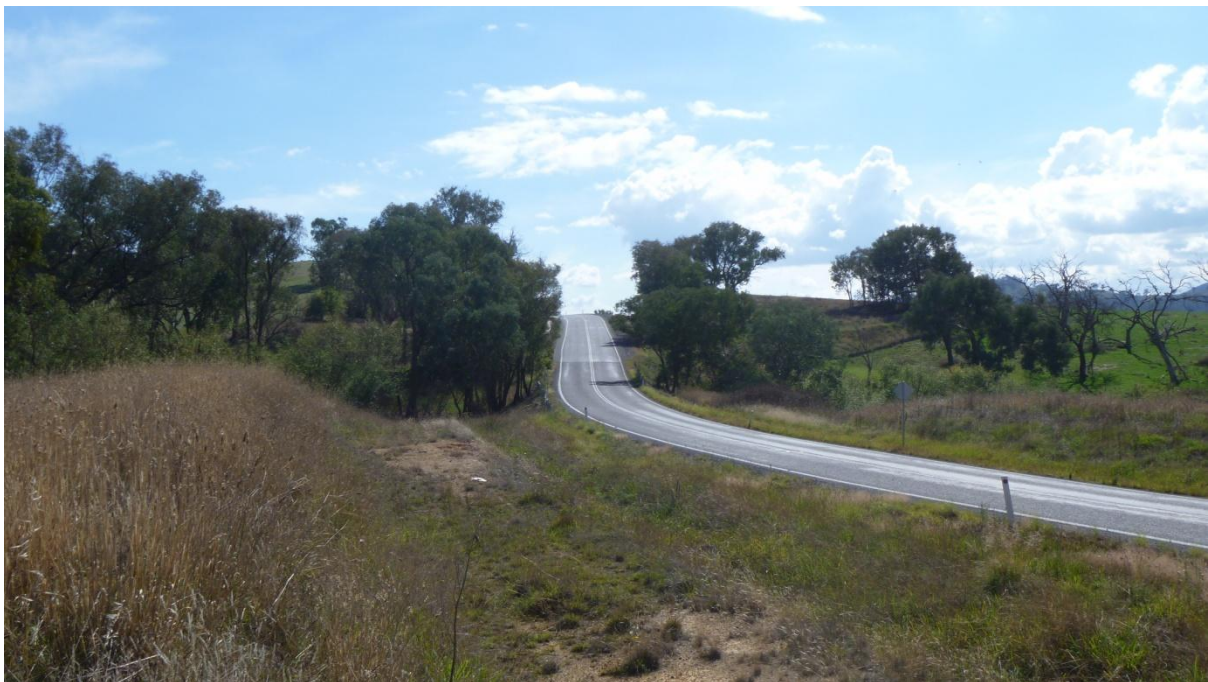
Figure 4.56: Context view of the current Gocup Road alignment, looking north, with the timber crossing located in the drainage line at left of view. A section of the old road surface is visible in foreground.
