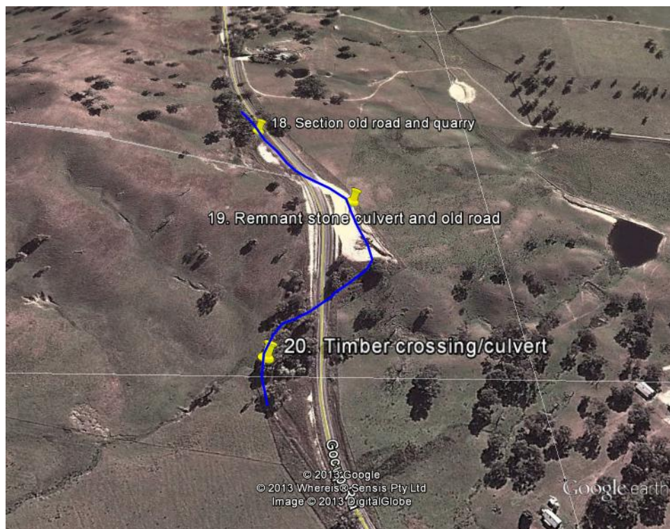
Figure 4.48: Location of section of old road surface and quarry #18 in relation to the abandoned road alignment (shown in blue), the current Gocup Road alignment, and two associated sites #19 and #20. Source: Google Earth, 2103.
