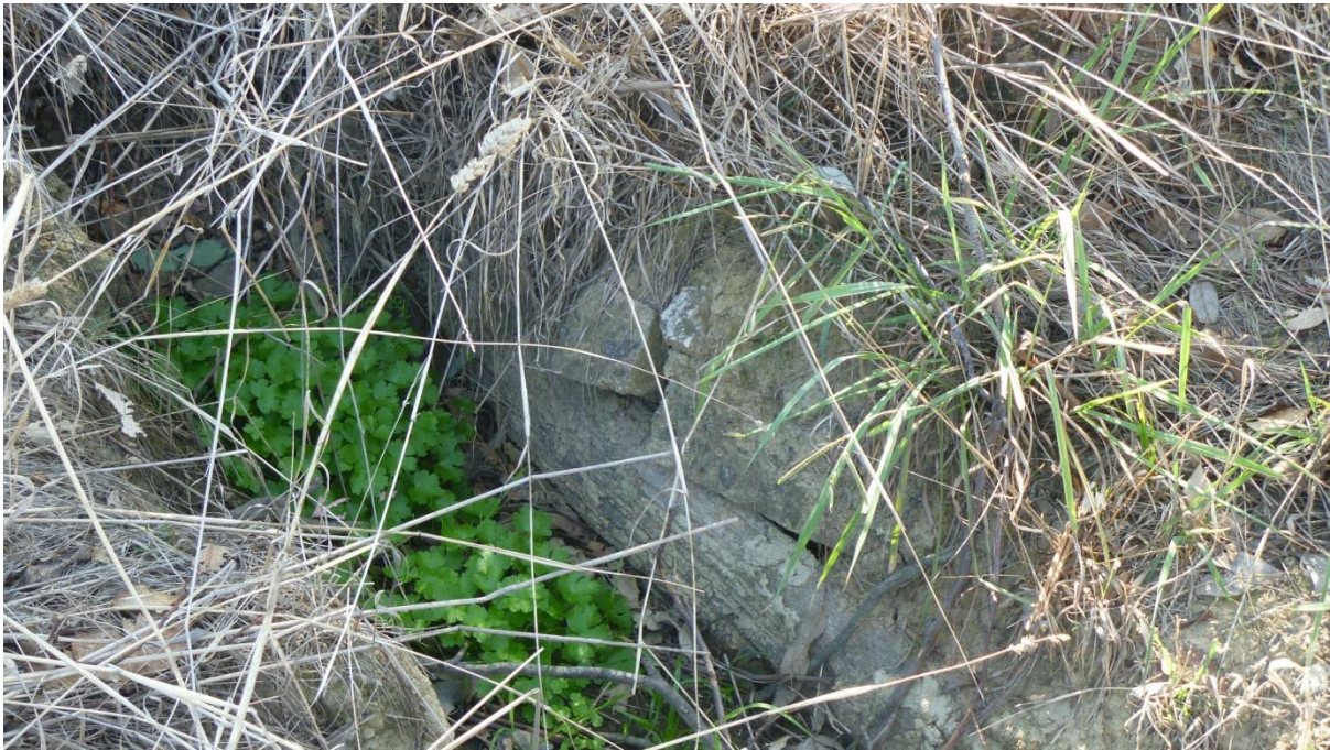
Figure 4.61: Detailed view of timbers with stone rubble and earthen surface.
