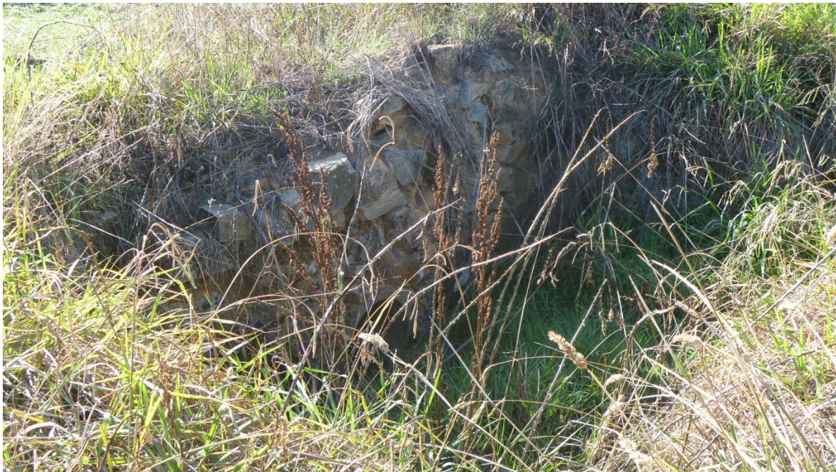
Figure 4.19: Detailed view of stone and earthenware pipe culvert.
