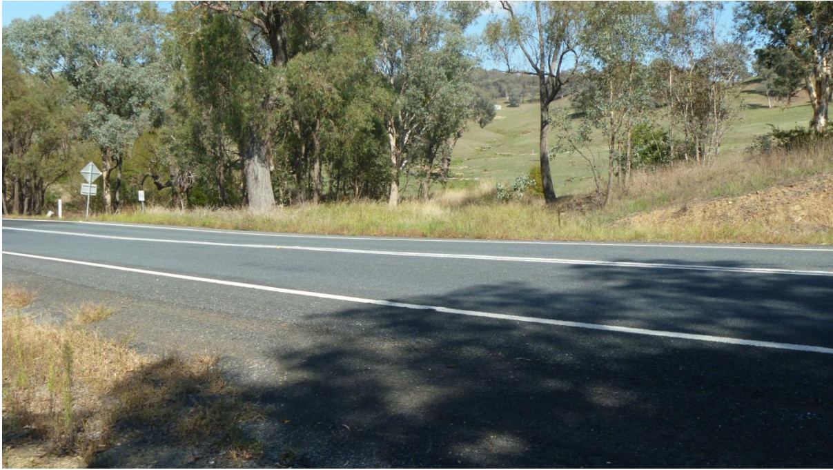
Figure 4.57: View of the approach to the timber crossing. The former road alignment crossed the present Gocup Road at this point and continued along the tree line to the gully below. .
