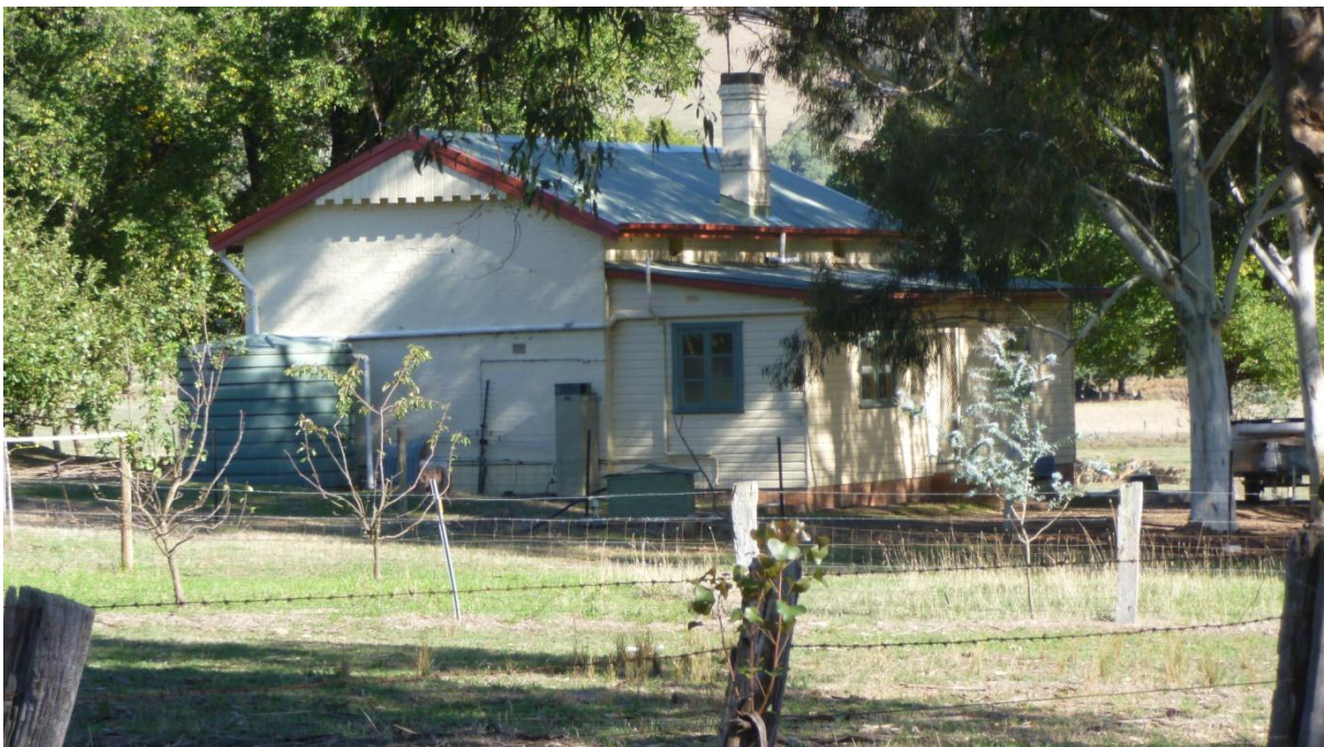
Figure 4.46: Detailed view of school house building, looking north-west, now being utilised as part of a private residence.
