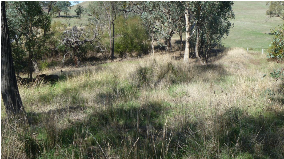
Figure 4.58: Northern approach to the timber crossing with the old road surface obscured under demolition rubble of old road. The old road surface would have provided a solid base for heavy vehicles to dump their loads.
