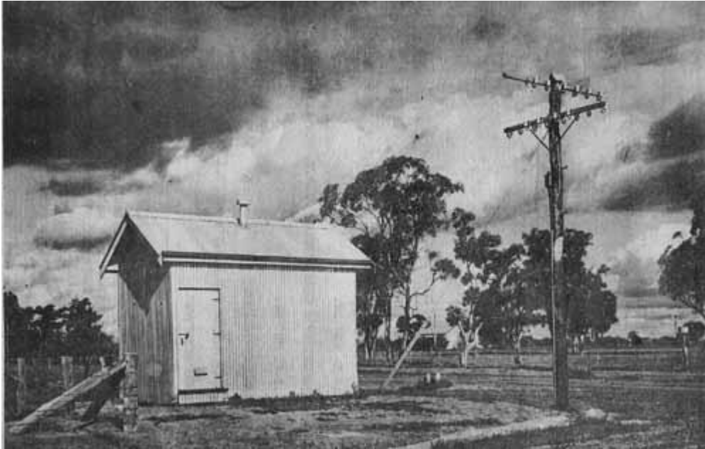
Figure 4.41a: An example of a rural automatic telephone exchange circa 1920, housed in a corrugated iron shed.
