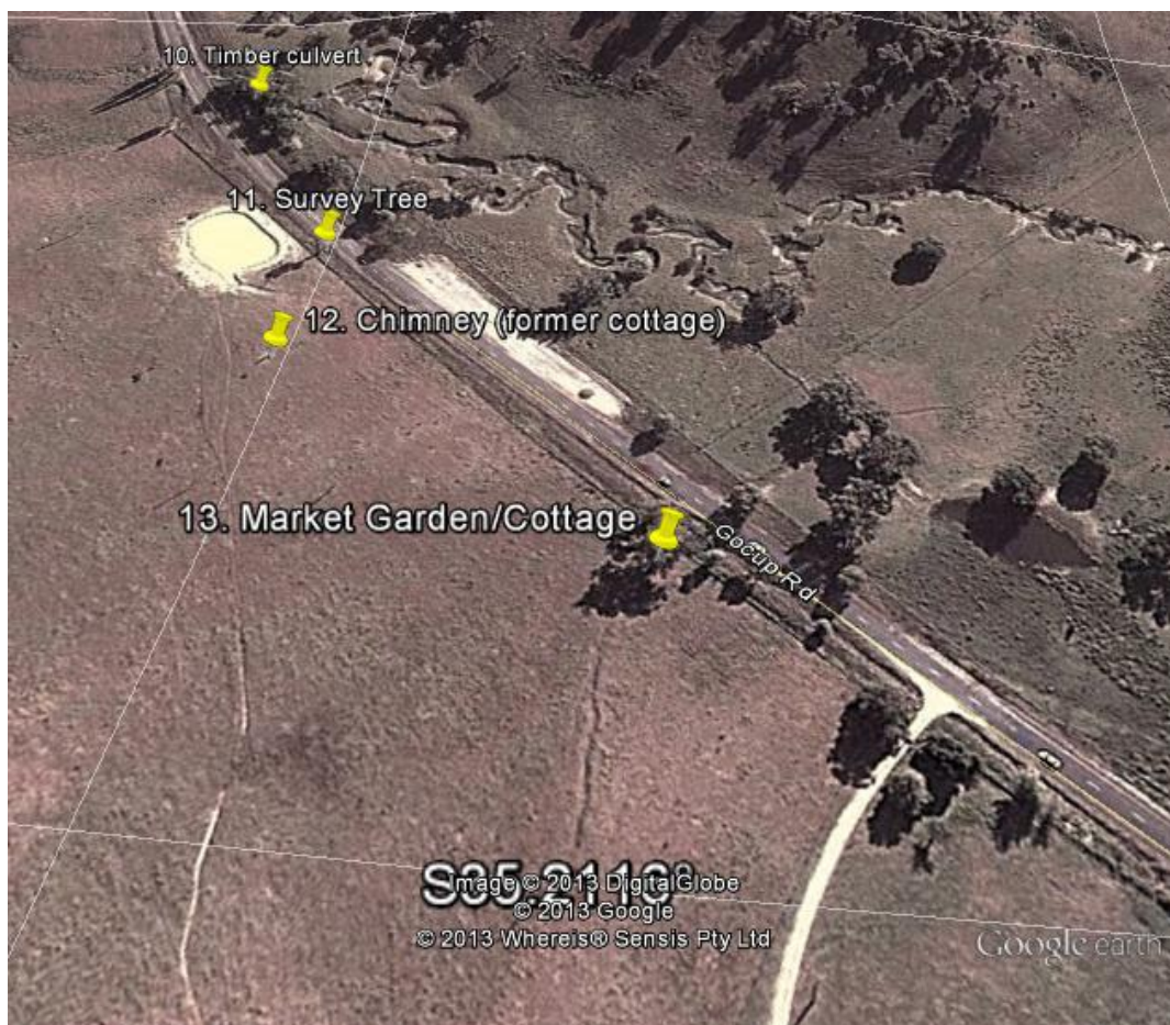
Figure 4.30: Location of former market garden and cottage in relation to the brick chimney #12 and SSM 5356 #11 showing close proximity to Gocup Road.
