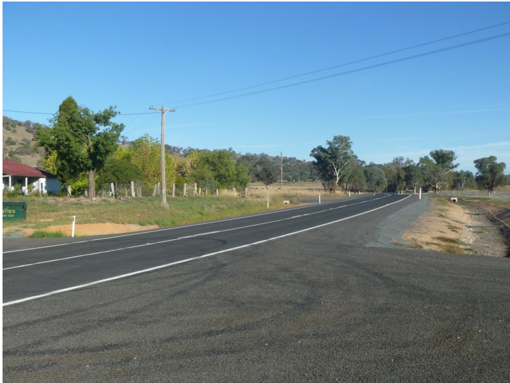
Figure 4.40: View of recent upgrade works adjacent to the former telephone exchange, which is just out of view to the left.
