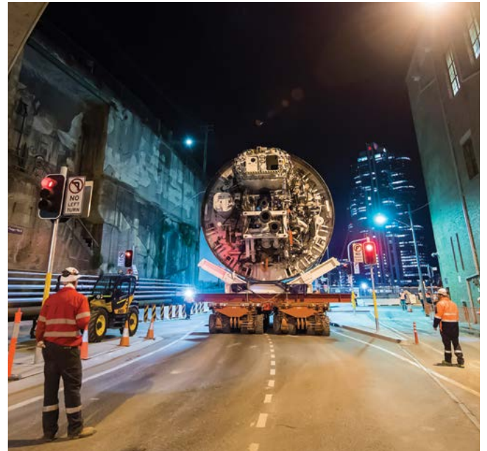
Tunnel boring machine used on the Sydney Metro project.
