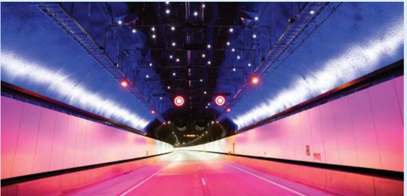
Longer tunnels, such as NorthConnex (pictured) include aesthetic design features to reduce monotony and help motorists maintain their concentration, reducing risk of incidents.
