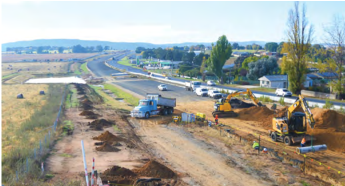
Drainage pipe extension work at Raglan, looking east.
